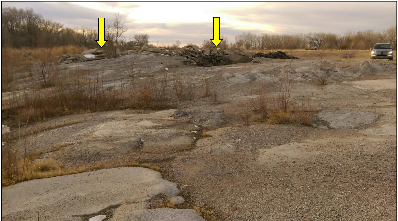
Photo 8. View looking west across layer of concrete along northern edge of small “slurry pond” in west mining area. Unhardened concrete was poured here many years ago during batch plant operation. Note location of inert material imported for backfilling stored adjacent to pond (indicated).
