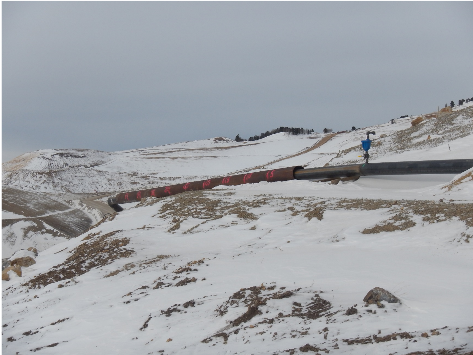
Photo 4 Edge of the Ball Mill Geomembrane Liner
