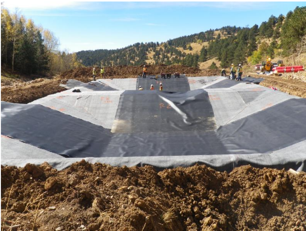
Underdrain Ponds – Geomembrane deployment.
