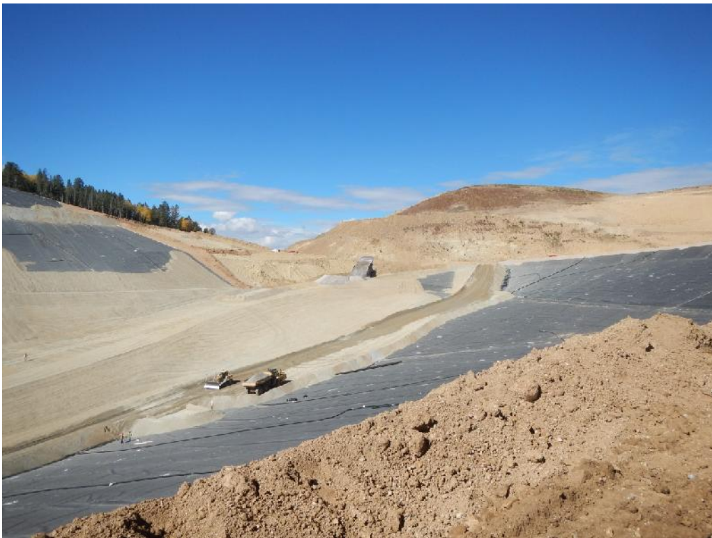
Phase 1 – Crushed Ore delivery.
