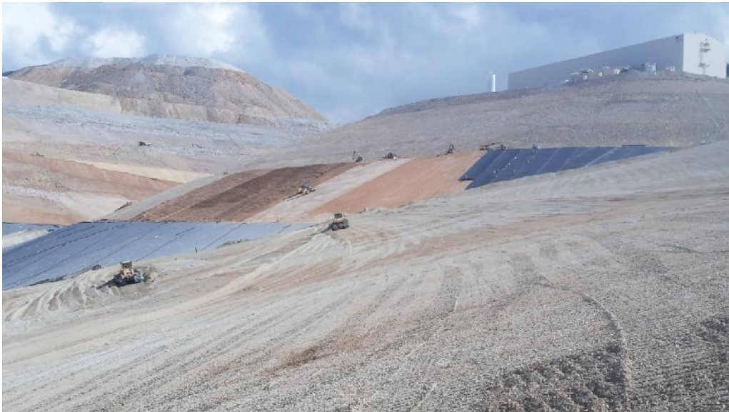
Phase 1 – DCF placement, geomembrane deployment and SLF compaction.
