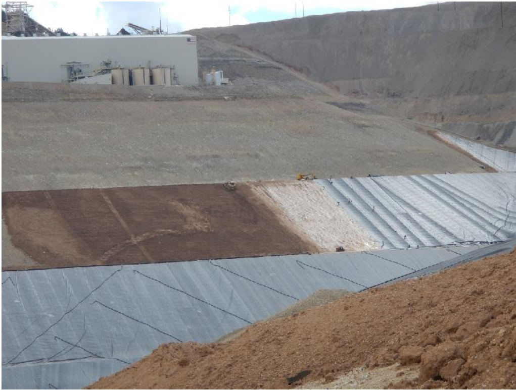
Phase 1 – SLF placement and geomembrane deployment.
