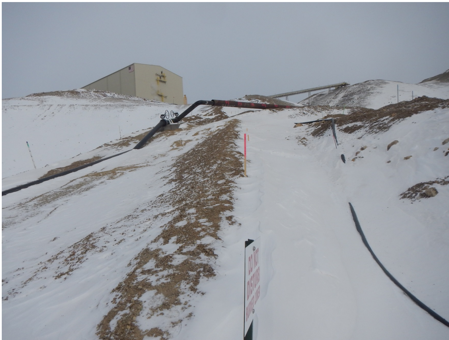
Photo 3 Posts Denoting Edge of SGVLF Geomembrane Liner
