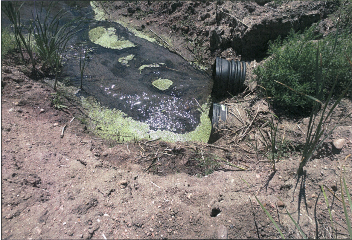
Photo 3: Two 18-inch CMP pipes, installed through the slurry wall. As approved under the temporary plan.
