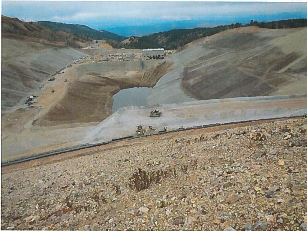
PSSA – DCF and Crushed Ore placement.
