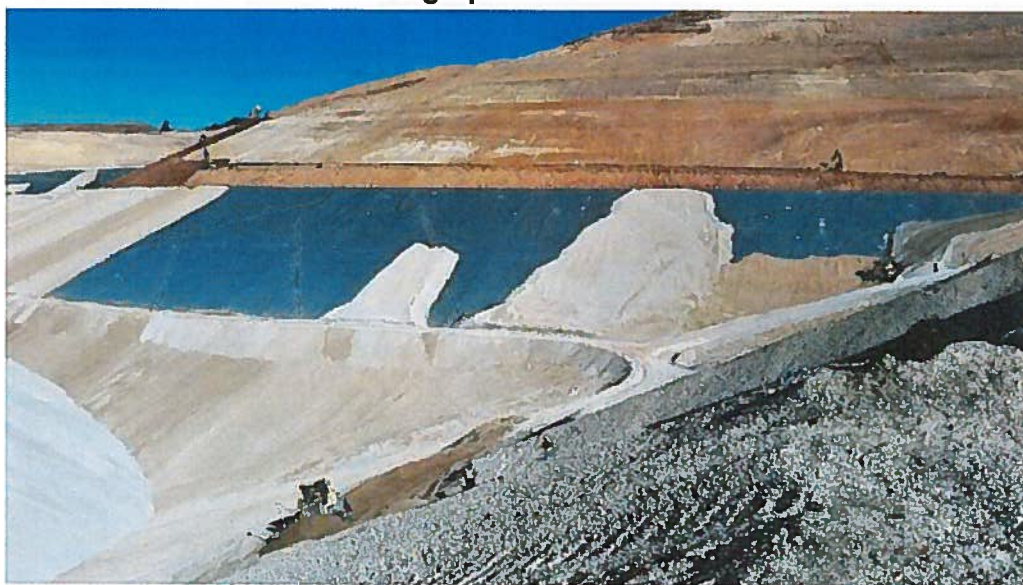
Phase 1 – DCF placement, leak detection excavation and SLF haul.
