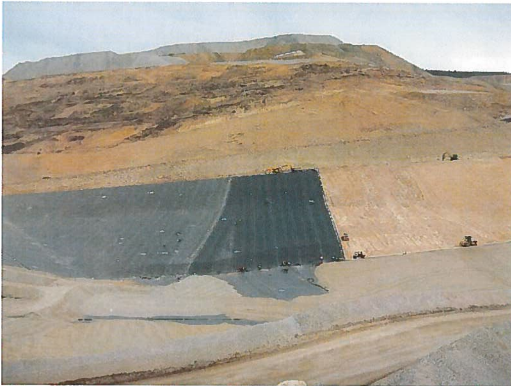
Phase 1 – Geomembrane deployment.
