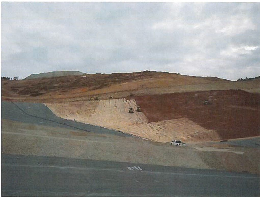
Phase 1 – SLF placement and compaction.
