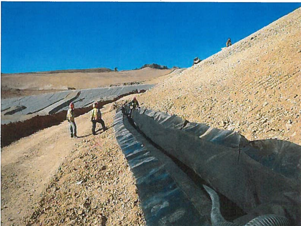
Phase 1 – Leak Detection installation.
