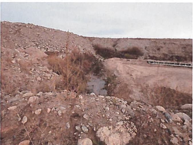
Figure 5: Diversion ditch placed at the base of the highwall
