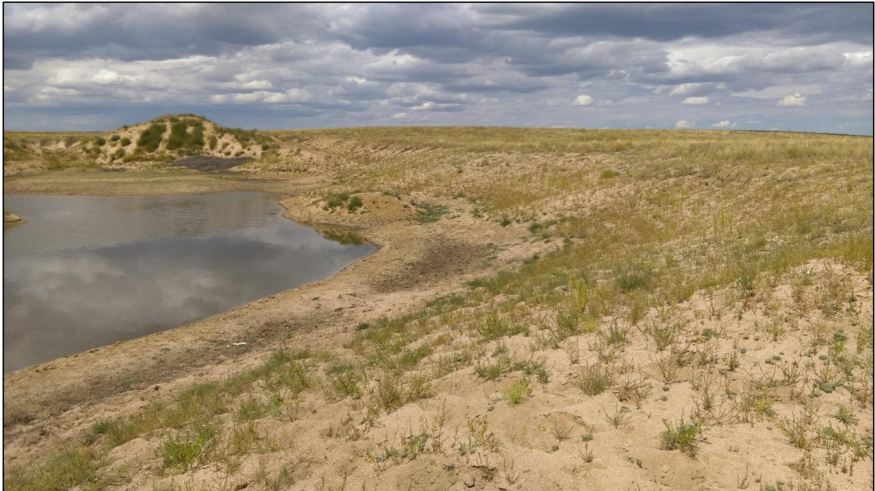
Photo 13. View looking west across northern mined bank, showing slopes graded to 3H:1V or flatter.
