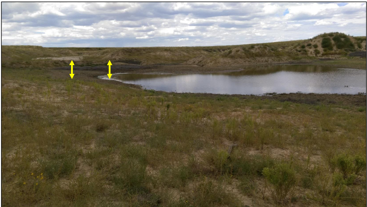
Photo 4. View looking northwest from southern pond bank, showing standing water in pit. Note pit floor is approximately 5 feet below upstream creek bed elevation (indicated).
