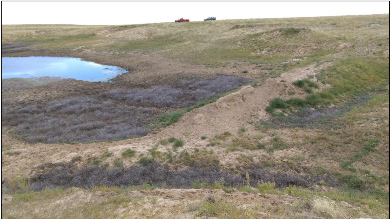
Photo 9. View looking southeast, showing damage to earthen berm caused by high flow event(s) in the creek
