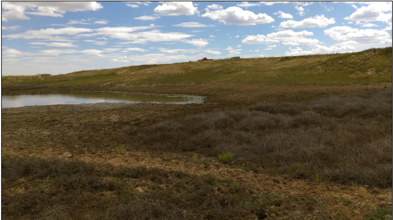
Photo 15. View looking southeast across southern pond bank, showing slopes graded mainly to 3H:1V or flatter, with some slightly steeper portions.
