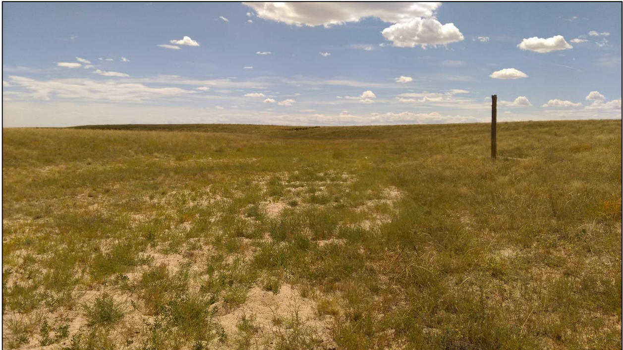
Photo 3. View looking downstream from southeastern edge of permit area, showing creek bed dry at the time of the inspection. Note creek bed is relatively level with surrounding topography just downstream of pit.
