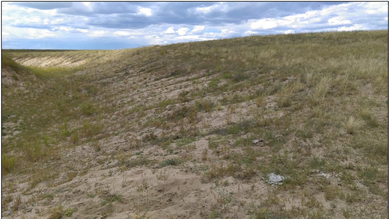
Photo 14. View looking southwest across northern mined bank (behind material stockpile), showing slopes graded to 3H:1V or flatter.
