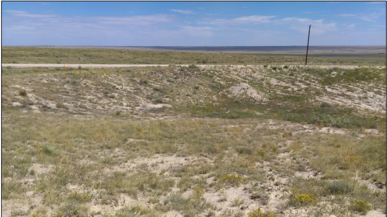
Photo 9. View looking north across (earlier mined) northwestern portion of site, showing slopes graded to 4H:1V or flatter. Note slightly more vegetative cover here than in other disturbed areas.
