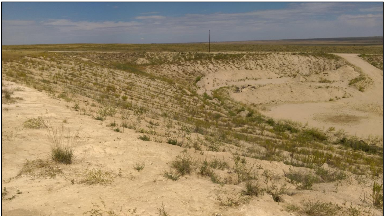
Photo 6. View looking north across western mined wall, showing slopes graded mainly to 3H:1V or flatter.
