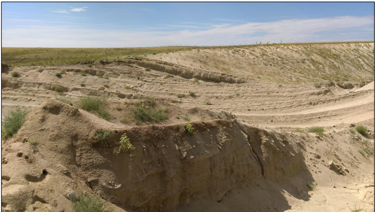
Photo 4. View looking south across most recently mined eastern pit wall, showing slopes graded mainly to 3H:1V or flatter.
