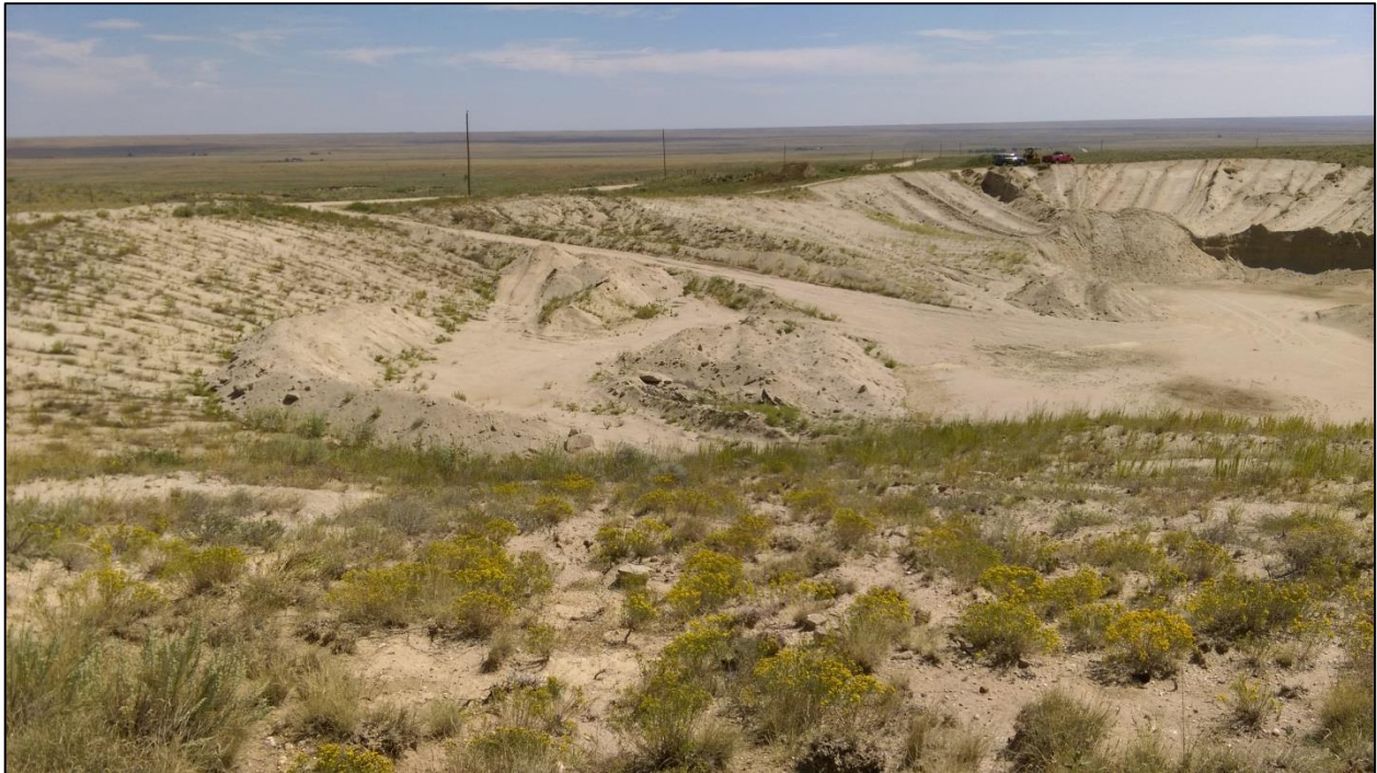
Photo 7. View looking northeast across (earlier mined) northwestern portion of pit, showing slopes graded closer to 4H:1V.
