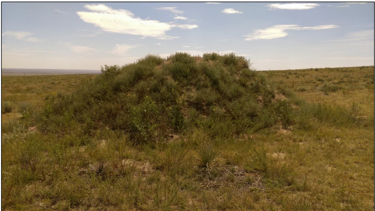
Photo 8. View of small topsoil stockpile stored east of pit, stable with vegetative cover.
