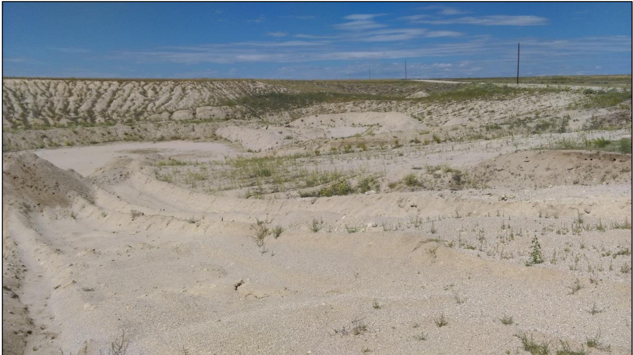
Photo 3. View looking northwest across pit from eastern edge, showing slopes graded mainly to 3H:1V or flatter.
