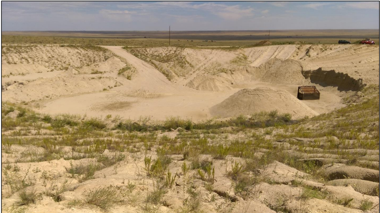
Photo 5. View looking east across pit from western edge, showing slopes graded mainly to 3H:1V or flatter. Note the few small material stockpiles stored on pit floor.
