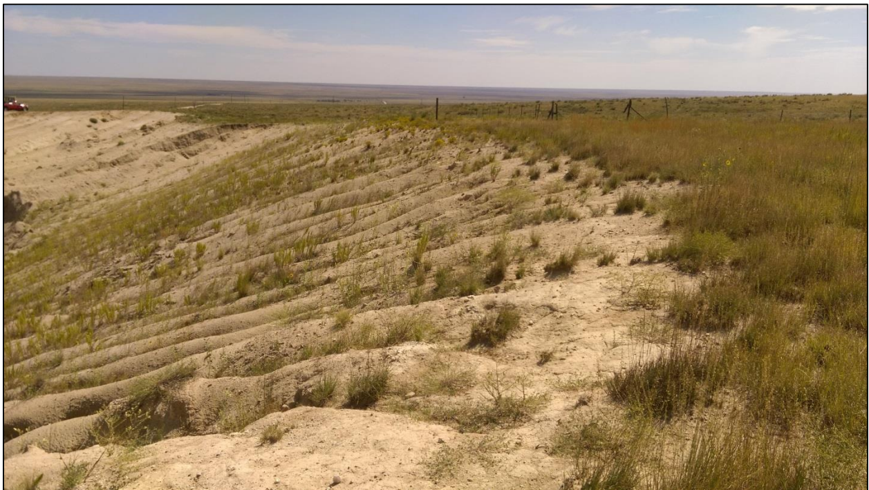
Photo 10. View looking east across southern mined wall (graded to 3H:1V). Portions of this disturbance are within only 10-20 feet of the southern permit boundary.
