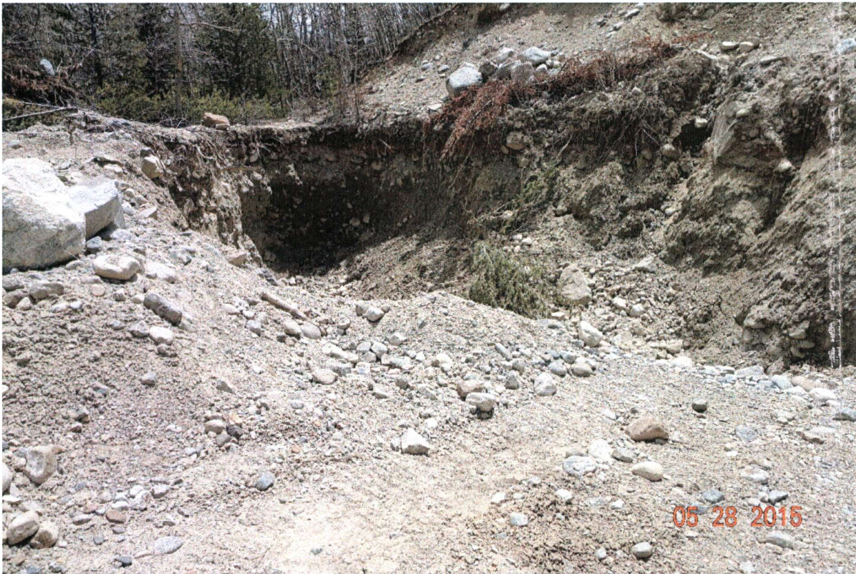
Photo 2- Settling Pond 3 showing no water present.
