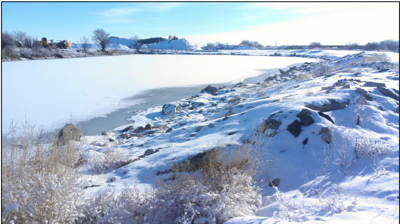
Photo 10. View looking northeast from southwestern edge of pond, showing concrete rubble lined bank with approximate 2.5H:1V slope gradients.
