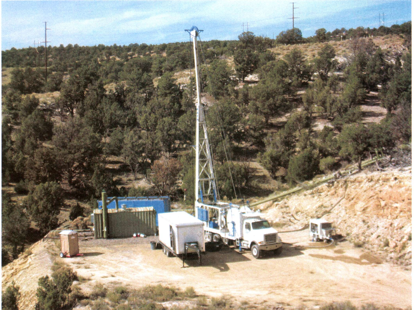
Photo 21 – Rigging up to plug and abandon production well 29-34 in October 2014. The smaller drill rig and shallow coil are ideal for the work needed on these small footprint well pads. The lateral pipe extending to this well comes in from the top across the undisturbed ground rather than parallel to the access road for this well. This was a shorter distance to lay the pipe. Care will be observed in removing this run of pipe from the well field so that the established vegetation is not disturbed.
