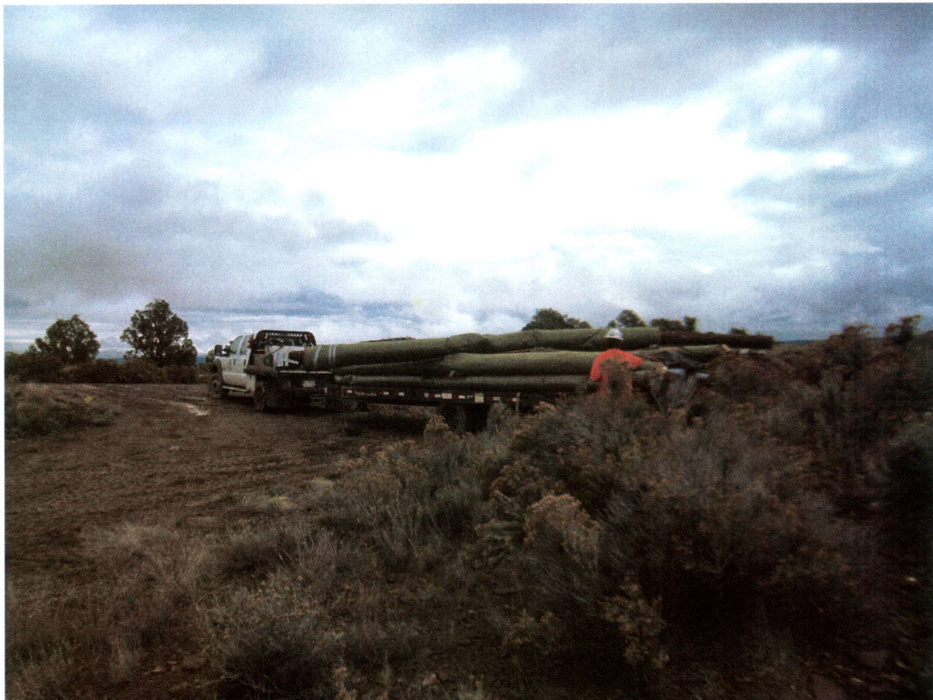
Photo 26 – An estimated 44,000 feet of carbon steel pipe twists and runs through the well field extending down the lateral lines and along the main well field road. Nearly all runs of pipe are in pairs and in some sections there are three runs of pipe side-by-side. Along each run of pipe is a series of 4 to 12 cables which also have to be removed. Both the pipe and the cable bundles are cut into 27 foot sections and loaded for transport to the Parachute site. Before the loaded pipe trailer leaves the well field the ends of each section of pipe are capped to prevent debris from blowing out as the pipe is transported. Insulation that is removed from one foot sections of the pipe where it is cut is gathered up and put into a large covered dumpster at the test mine pad. A fire watch and water truck is on location during all work activity at the Picenace site. Once the pipe is transported to the Parachute site the remaining pipe insulation is removed on an asphalt pad that is easily cleaned.
