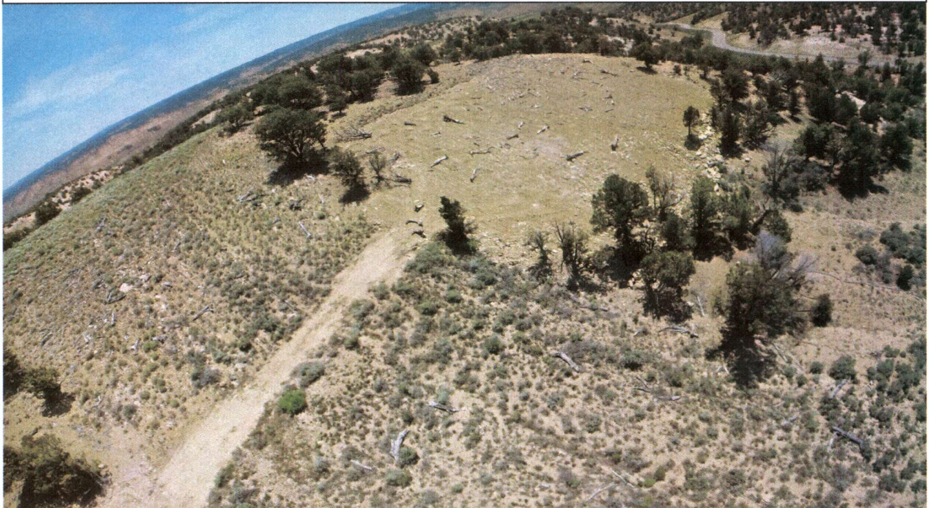
Photo 7 – Production well pad 20-35 after the pad was re-contoured, top soil distributed across the disturbance area and drill seeded. Trees removed during the construction of the pad which were stock piled then are now spread out across the reclamation area to provide habitat and to restrict access for motor vehicles. Photo taken June 2015.
