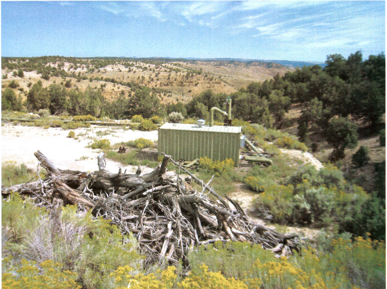
Photo 3 – Production well 29-26 location prior to plugging and abandonment. The short string on production well 29-26 failed to hold pressure and was plugged and abandoned using tremie- line cement placement through shallow coil tubing in September 2014. The long string was also plugged to close out the location. The well skid was removed from the pad, the piping was all cut and removed and the location was restored to the original contours. The top soil pile was distributed over the newly contoured pad and the pad was drill seeded. All of the cut trees you see that were originally harvested from the location and stockpiled when it was created in 2000 are now spread out over the pad to provide habitat and to restrict vehicle access.
