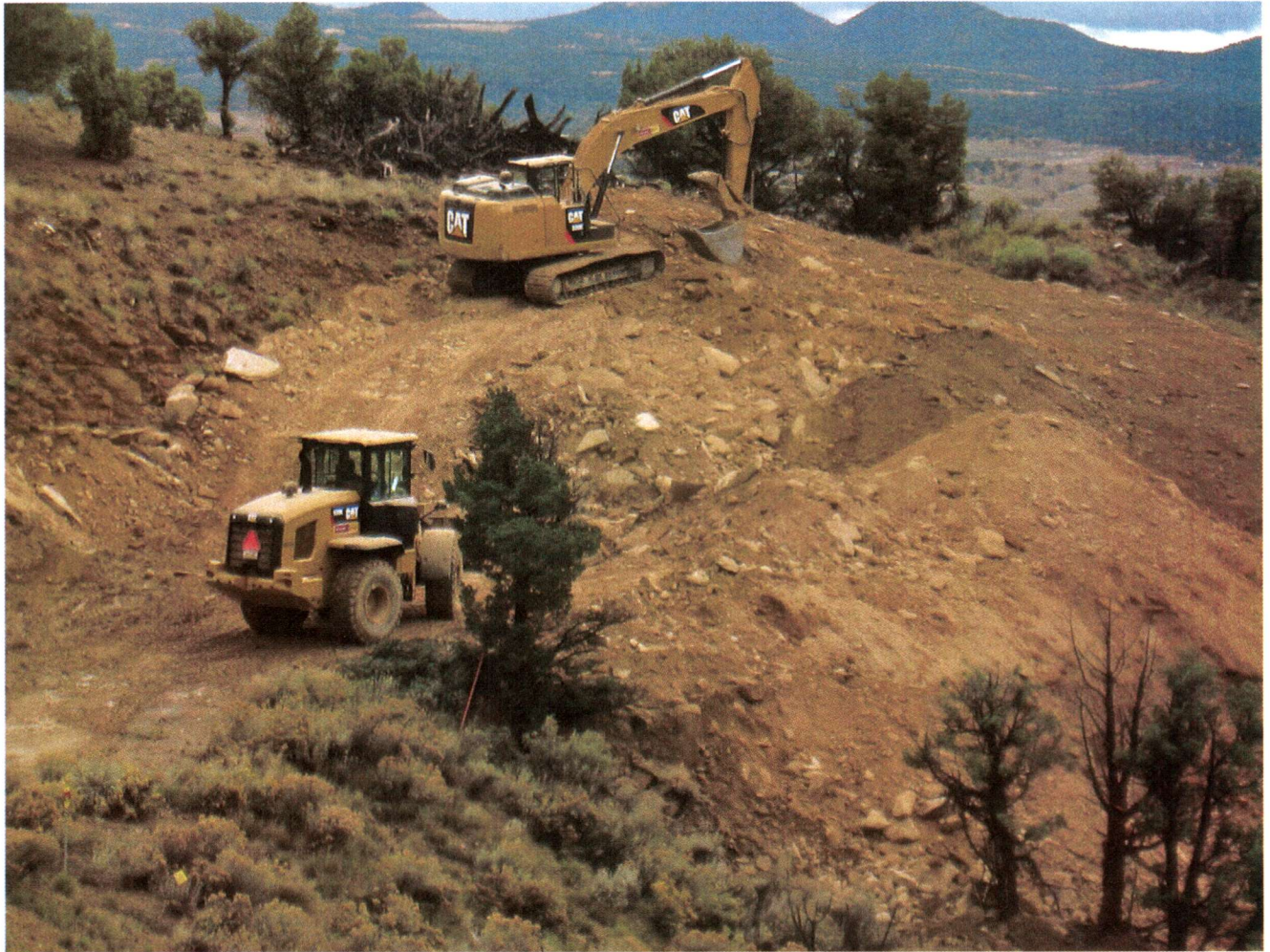
Photo 24 – Construction equipment moving dirt to re-contour production well pad 20-35 in September 2014. Smaller sized equipment that can move in a tighter radius is used for this work so that the maximum amount of mature pinion juniper trees along the margins of the pads can be preserved as cast over slopes are restored. The loader easily works around the pinion juniper tree on the edge of this pad so it can remain undisturbed.
