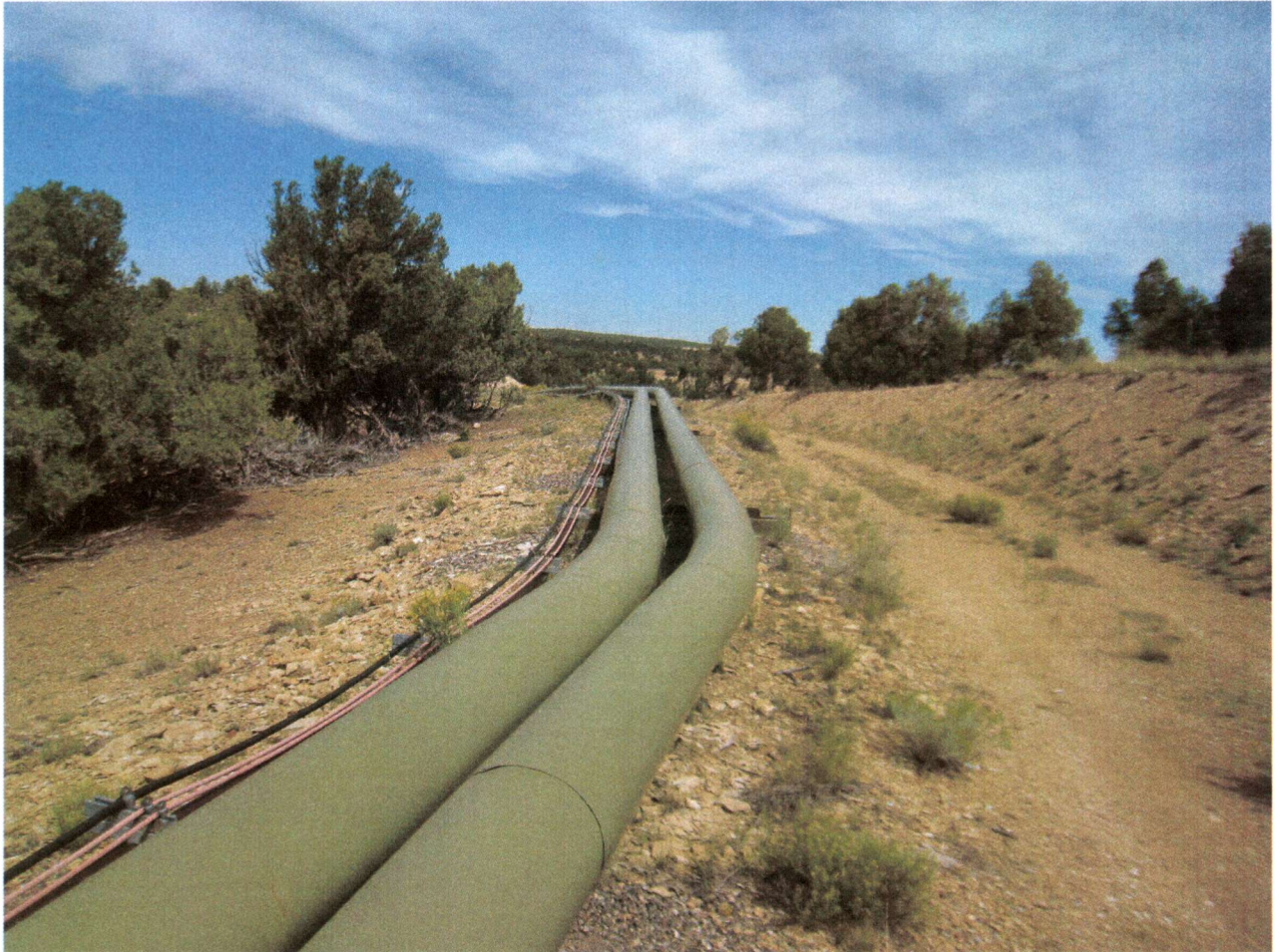
Photo 27 – Dual lateral piping and accompanying four lines of cable extending along the access road to production well 29-28. All of the piping and cables extending to production well 29-28 were removed and transported to the Parachute site in October 2014. Not all pipe lines run adjacent to the lateral roads. Pipe lines extending from the main well field road across country in a more direct route for a shorter distance to wells which are more remotely located are carefully removed to preserve the established vegetation.
