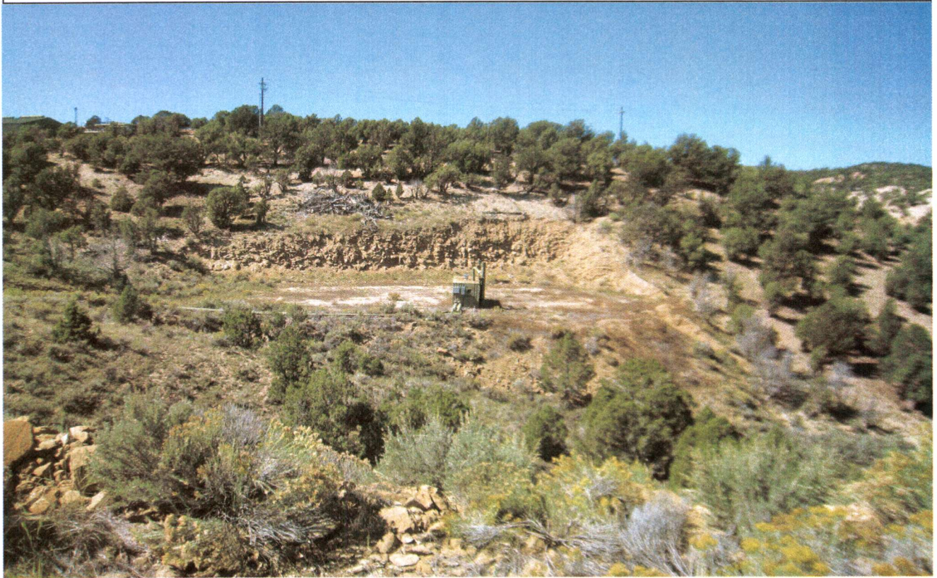
Photo 16- Production well pad 29-24 in fall 2014. Well skid and piping are still in place. This location has an extensive cut slope and the lateral access road into it intersects a complex two leg drainage into Yankee Gulch.
