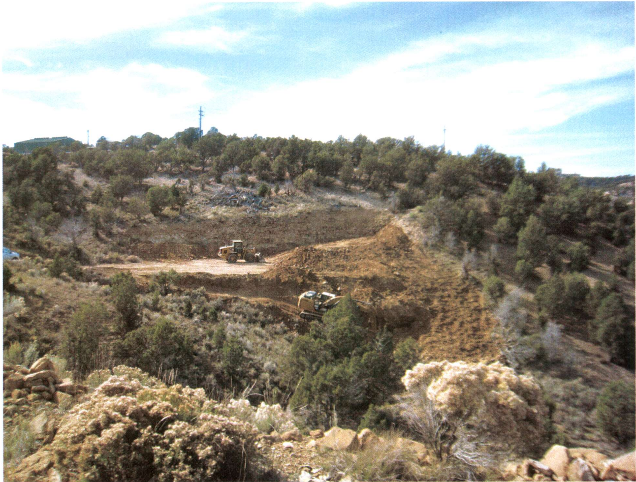
Photo 25 – Re-contouring and drill seeding of production well pad 29-24 has been the most time consuming location to reclaim so far. The cut slope on this location is substantial and the cast over slope and lateral road incorporated a more complex storm drainage system that had to be self- sustaining and stable once the culverts were removed. The reclaimed slope was drill seeded by pulling the seeder across the slope with a skid steer. Some areas of this location were hand seeded.
