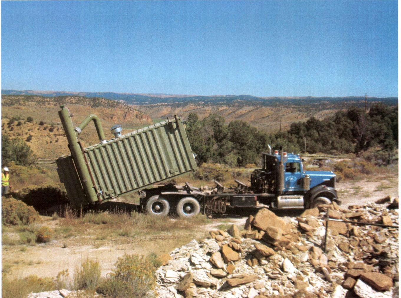
Photo 23 – After a production well is plugged and abandoned the well head is cut down and capped and a marker is welded in place to identify the well. Next the well skid and pipe are removed so the site is ready for re-contouring. In the photo above a well skid is being loaded on a truck for short transport to the test mine pad. The well skids are being temporarily staged on this location until they are all ready to be hauled out. Five well skids still remain on location connected to piping in the well field. Before transport on public roads each well skid must have the gas separator (14 foot tall pressure vessel mounted on the side) removed from the side and piping removed from the top to meet height and width road restrictions. Inside of some of the containers large valves not connected laying on the floor must be strapped down with chains to keep them from going through the end of the container as they are tilted onto a wench truck for transport. All of the pipe openings in the well skids are also covered to prevent loose materials from blowing or vibrating out during transport. This well skid is being removed from production well pad 29-68 in the fall of 2014.
