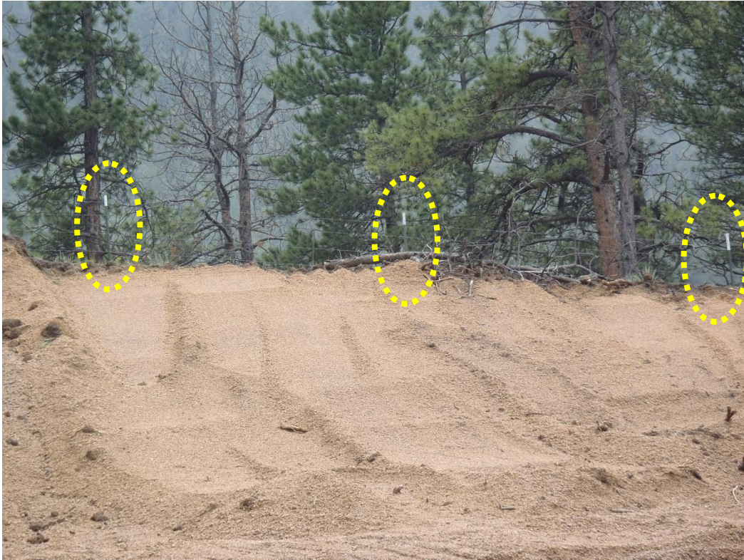
Photo 6. Backfill material being pushed down from the southern permit boundary (looking north). Note boundary fence posts.
