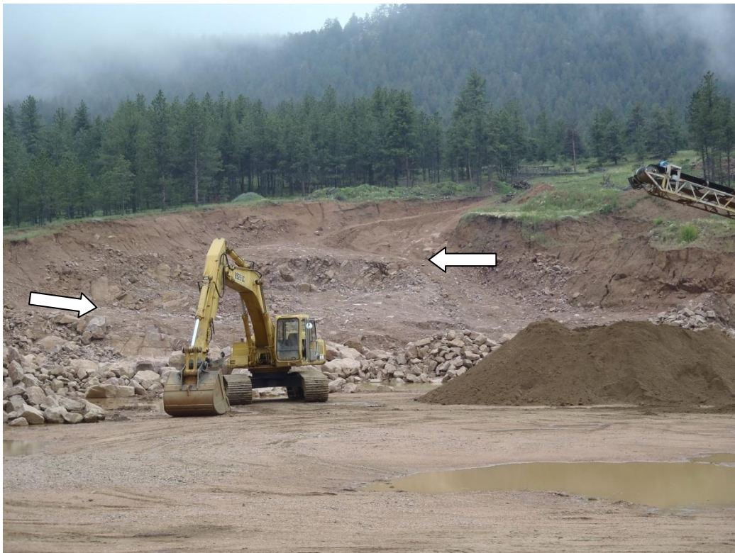
Photo 3. Southern end of pit, Note benches (looking south).
