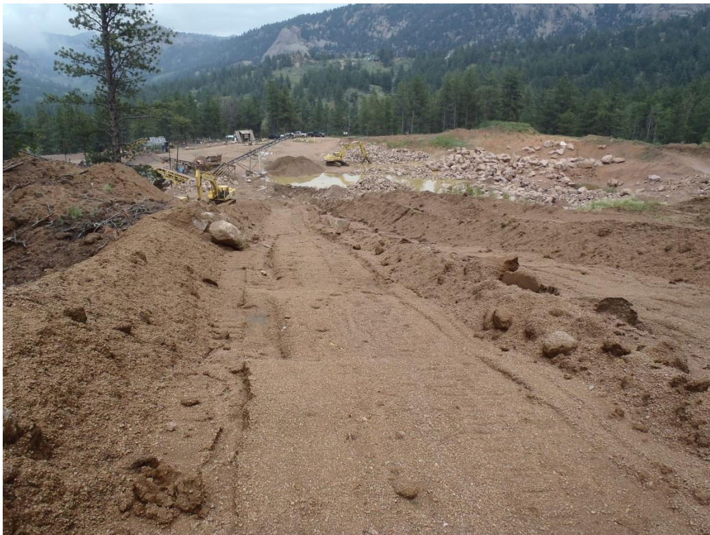
Photo 5. Backfill material being pushed down towards the pit floor (looking north).
