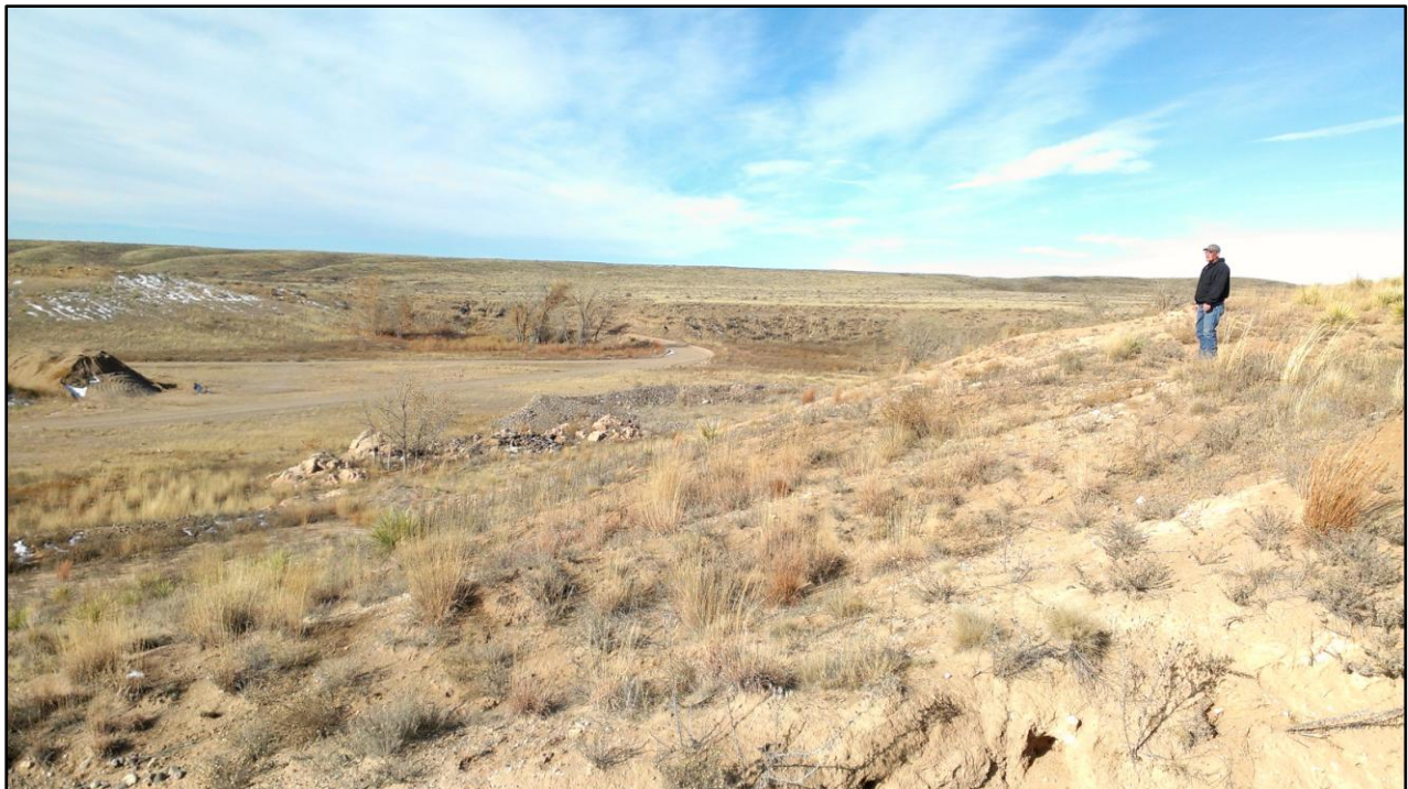
Photo 6. View looking northwest into pit from top of eastern pit wall, showing slopes graded to 3H:1V. Note native grasses and shrubs establishing across pit slopes.
