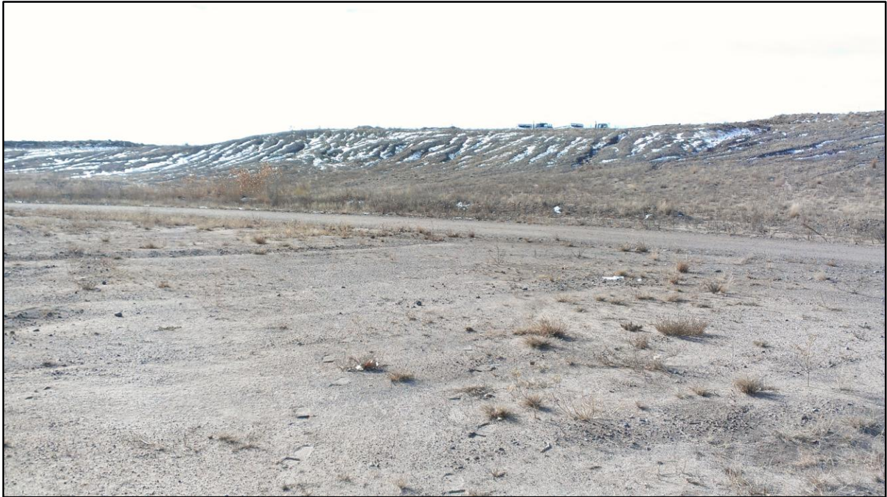
Photo 7. View looking southwest from northern portion of pit floor, showing western pit wall graded to near 3H:1V. Note some native grasses establishing across the slope. Also note some minor erosional damage present along some portions of the slope.
