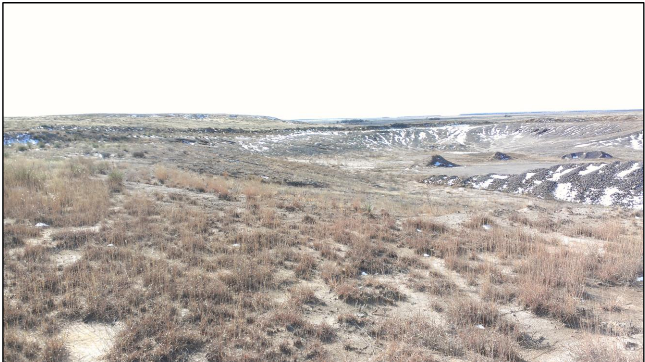
Photo 4. View looking southwest into pit from top of eastern pit wall, showing slopes graded flatter than 3H:1V. Note native grasses and shrubs establishing across pit slopes.
