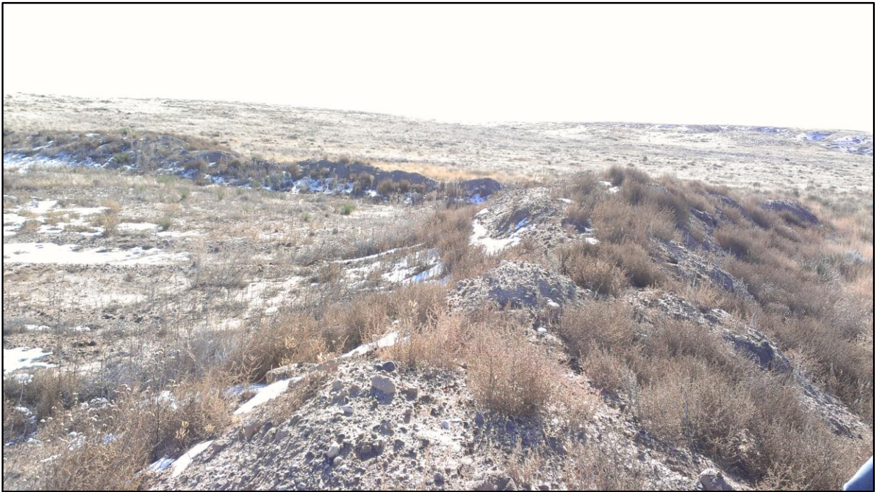
Photo 8. View of portion of topsoil berm stored along top of southern pit wall. Note berm appears to be stable with some vegetative cover (mainly Russian thistle).
