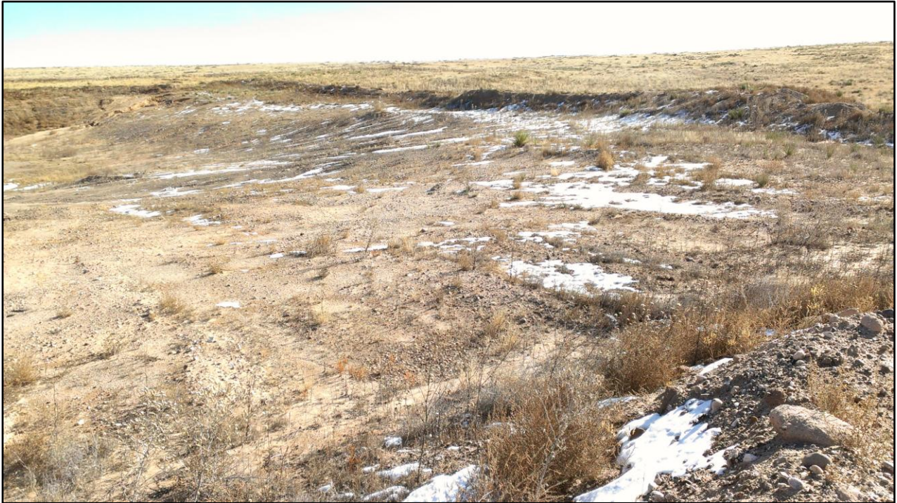
Photo 3. View looking south at southern pit wall, showing slopes graded flatter than 3H:1V.
