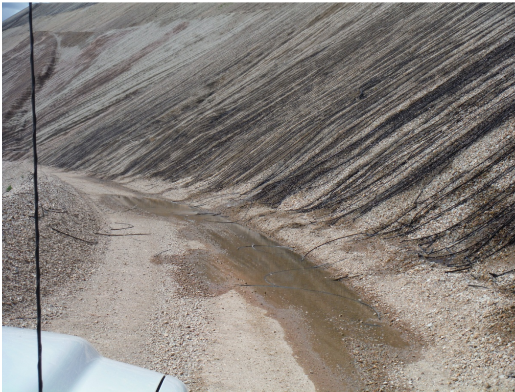
Photo 8. Poned solution from faulty drip line along the Phase V PSSA access road; looking northwest.
