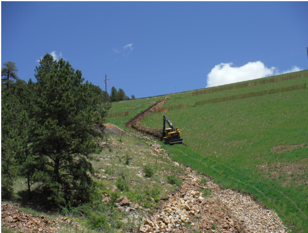
Photo 10. Trench being constructed for a temporary SGVLF underdrain pumpback line; northeast.
