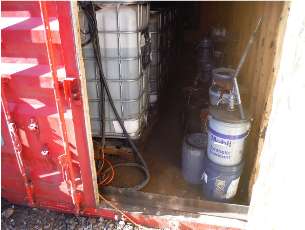
Photo 13. Conex storage container unit, welded lip at door is the secondary containment; looking south.
