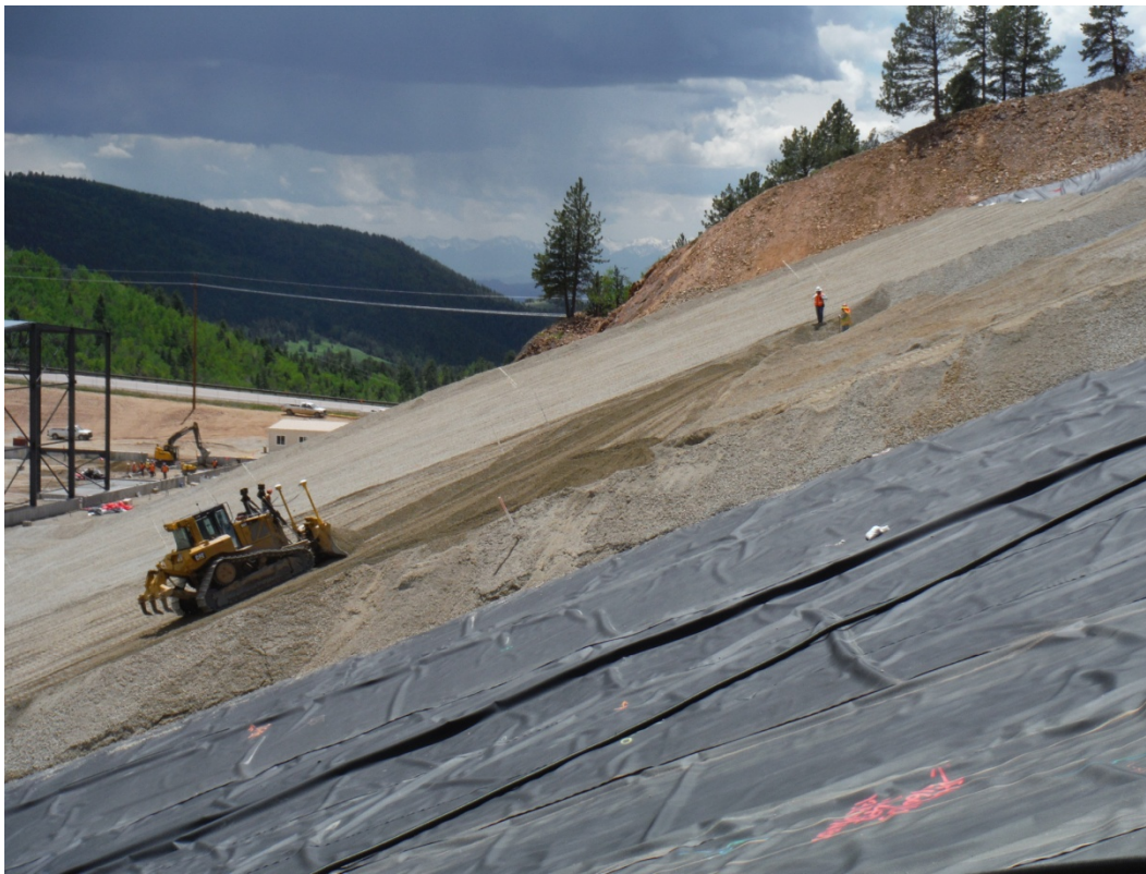
Photo 12. DCF placement; looking southwest.
