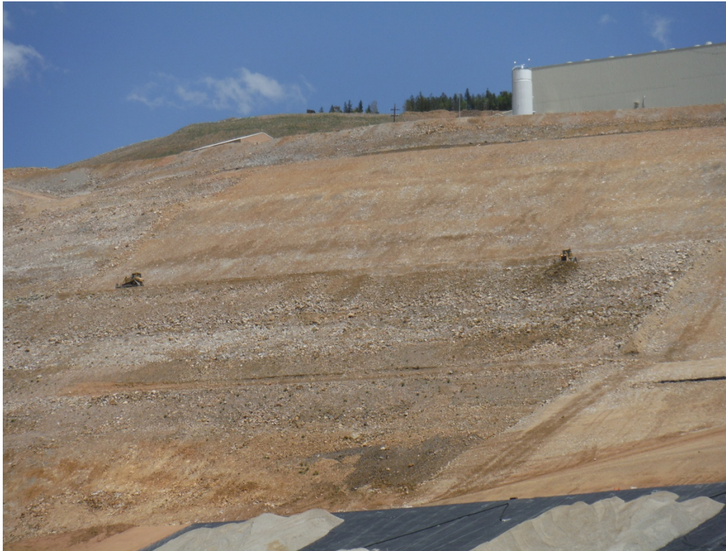
Photo 11. Bulldozers grading the ball mill slope; looking east.
