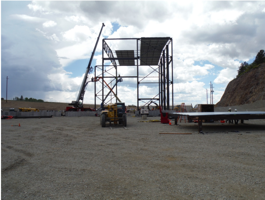
Photo 9. Construction on the ADR2, Low Volume Solution Collection System building located in the back right of the photo; looking southwest.
