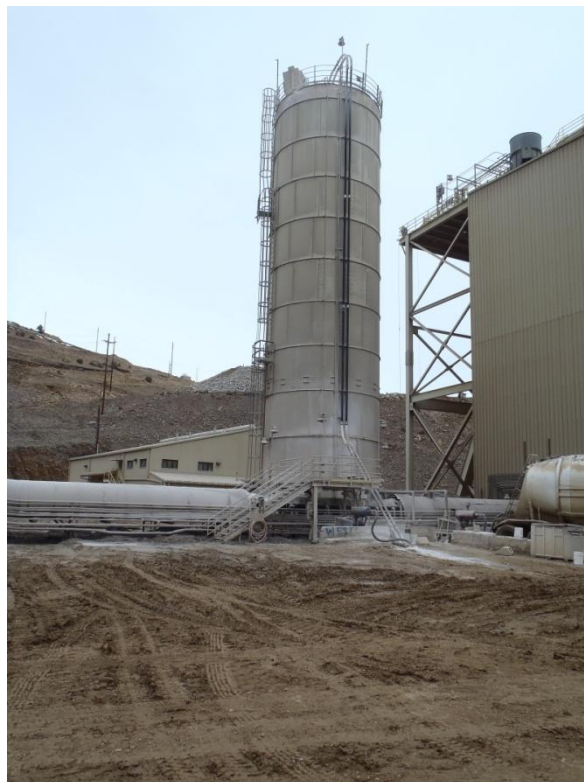
Photo 8. Lime Silo is located near the crusher and northeast toe of the Phase IV VLF (looking east).
