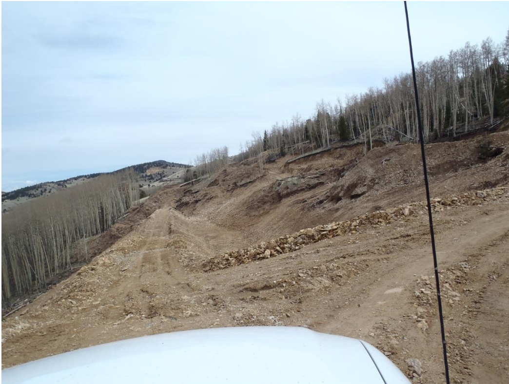
Photo 3. Nearly completed EMP 021 sediment ponds (looking NE).
