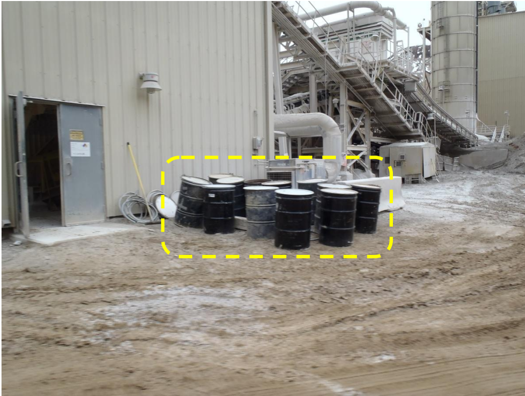
Photo 9. 55-gallon drums near Lime Silo appeared in good condition / no leaks were observed.
