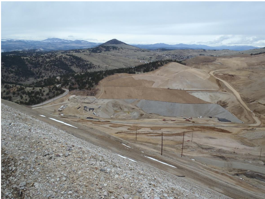
Photo 4. SGVLF construction progress (looking NW).
