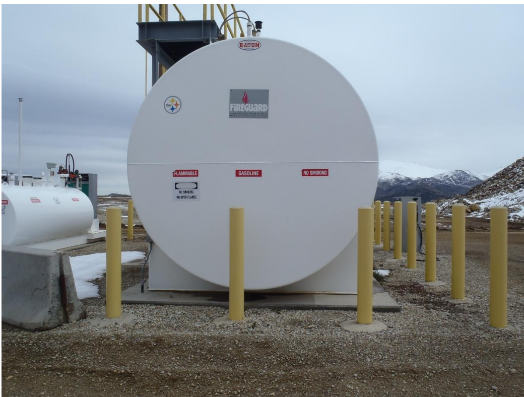
Photo 6. Fuel Island gasoline storage tank over liner with pipe bollards (looking NE).
