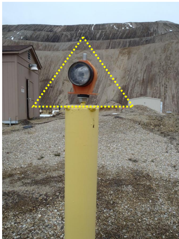
Photo 2. Retro-reflector used to monitor AGVLF slope movement (near Phase V LVCS shed).
