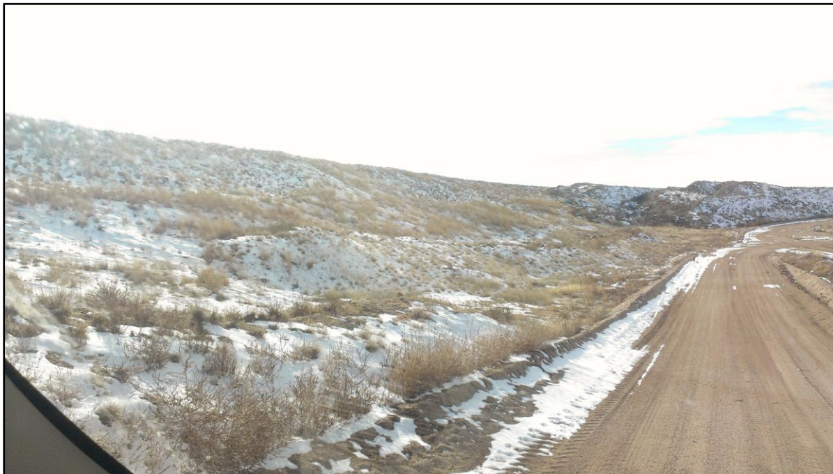
Photo 6. View looking west from haul road, showing portion of southwestern pit wall graded to approximately 2H:1V. This wall will need to be graded to 3H:1V or flatter before final release.
