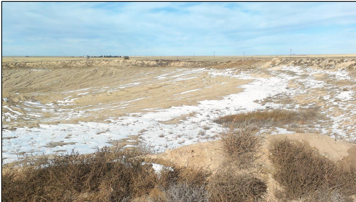
Photo 4. View looking northeast from top of southern pit wall, showing mined slopes kept at 3H:1V gradient or flatter. Note topsoil stockpiled in berms around edges of pit.
