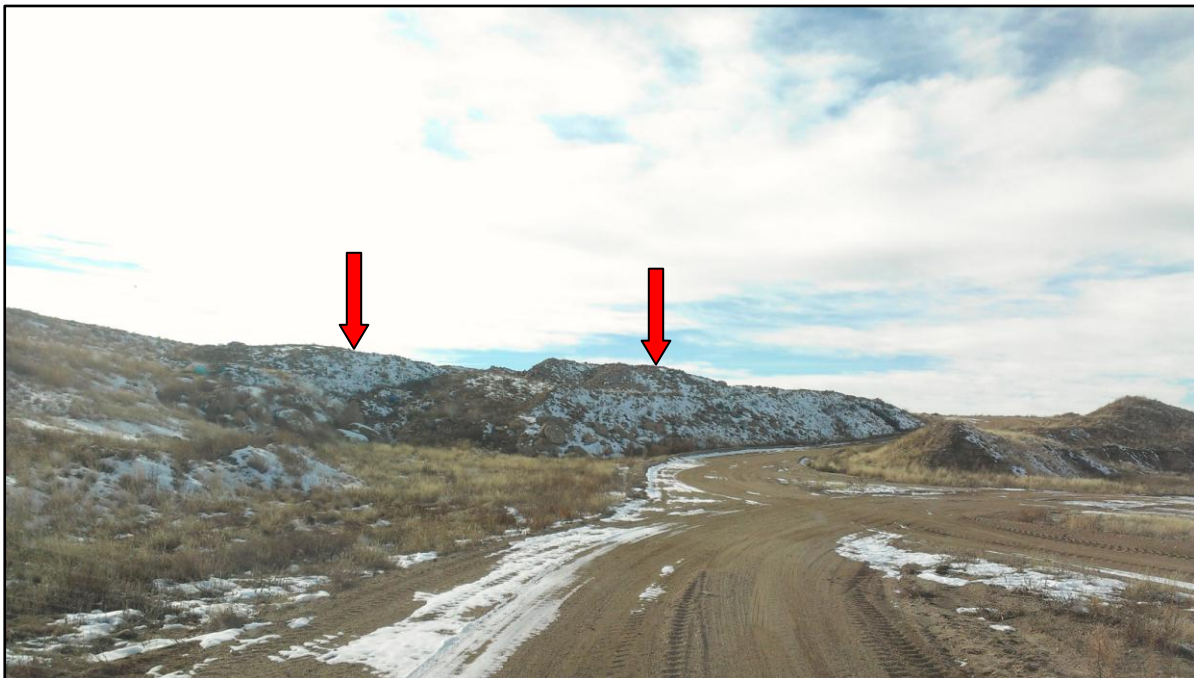
Photo 8. View looking west from haul road, showing portion of waste rock stockpile (indicated) that will need to be used for final reclamation or graded to 3H:1V or flatter before final release.
