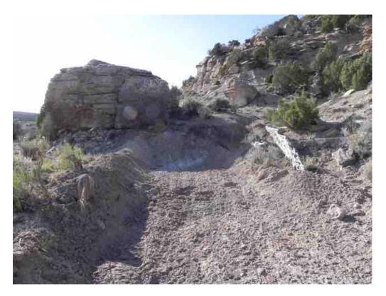
Subsided Guadalcanal shaft that was backfilled, with the two replaced barrier rocks that had washed off during the flood:
