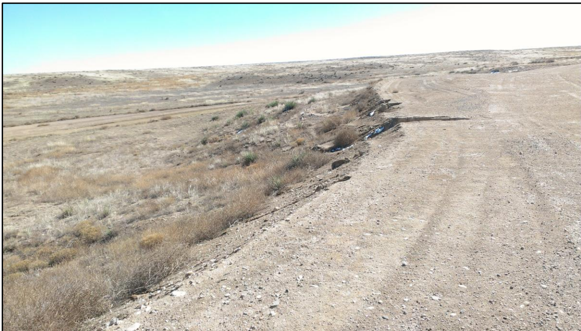
Photo 10. View looking east from northern edge of site, showing slope gradients of approximately 2.5H:1V to 2H:1V.
