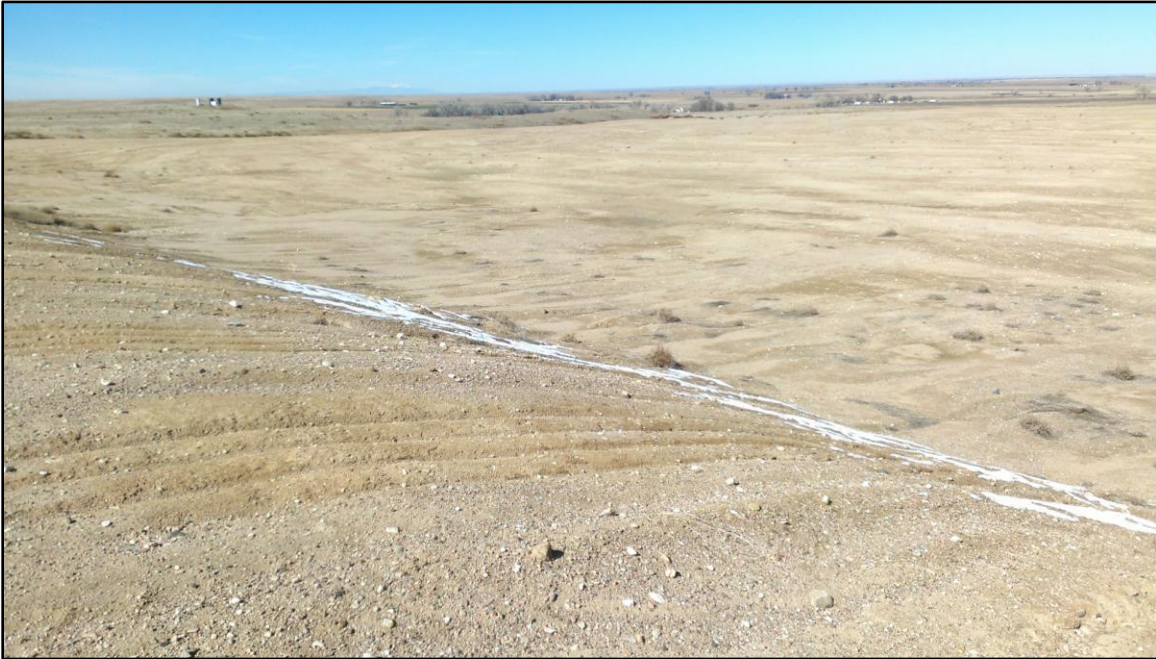
Photo 5. View looking northwest from top of southern mined slope, showing site has been graded to nearly flat.
