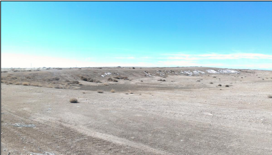
Photo 6. View of southern mined wall that was backfilled and graded to 4H:1V.
