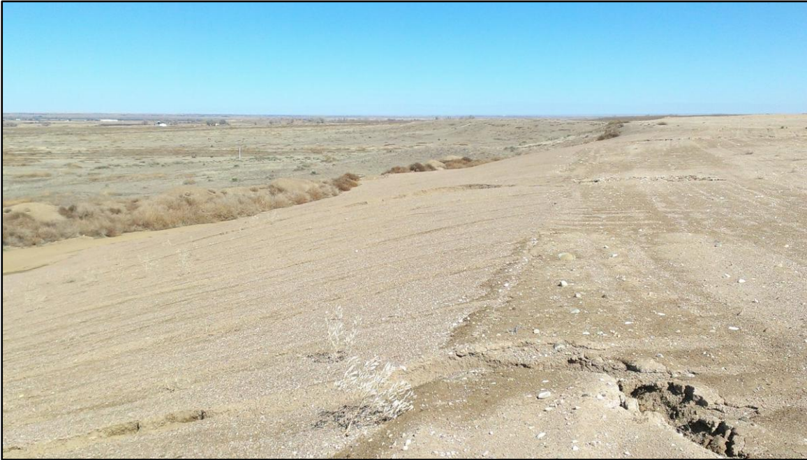
Photo 7. View looking north from western edge of site, showing slope gradient of approximately 4H:1V.
