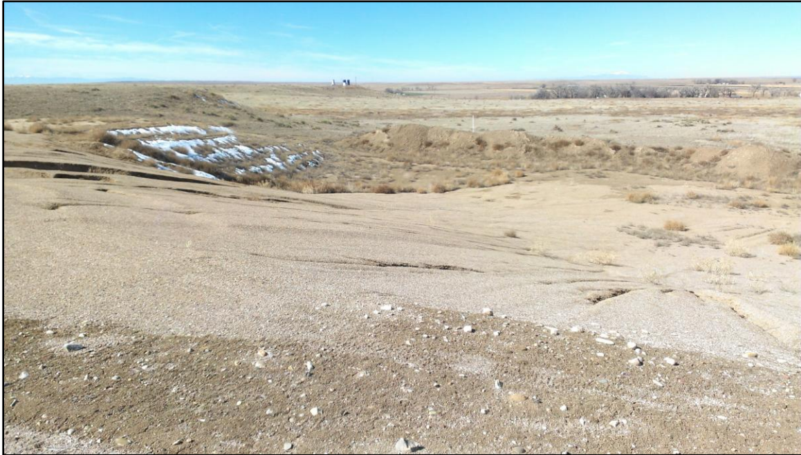
Photo 9. View looking southwest from western edge of site, showing slope gradient of approximately 4H:1V. Note low-lying berm constructed along western edge of lower elevation disturbance.
