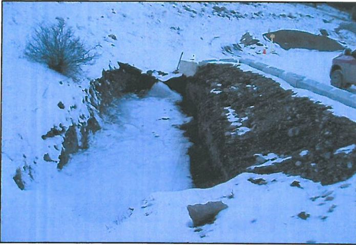
L and R, above: Stormwater catchment sump at base of road up to 9400 level portal
