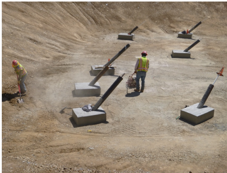
Photo 1 Closure Drain Pads
