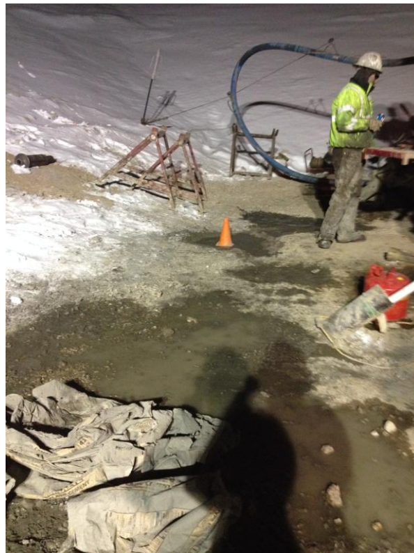
Photo 3. CD-5 was grouted to the surface and the casing was cut approximately 0.5ft below grade per Ames.
