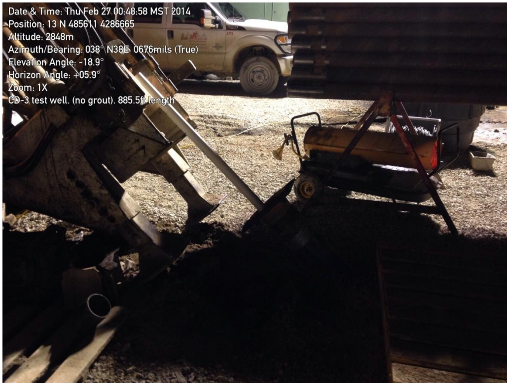
Photo 5. Drain is installed to 885.5 ft depth
