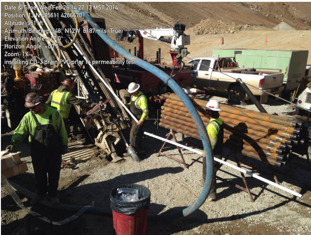
Photo 2. This is the first attempt to install the drain
