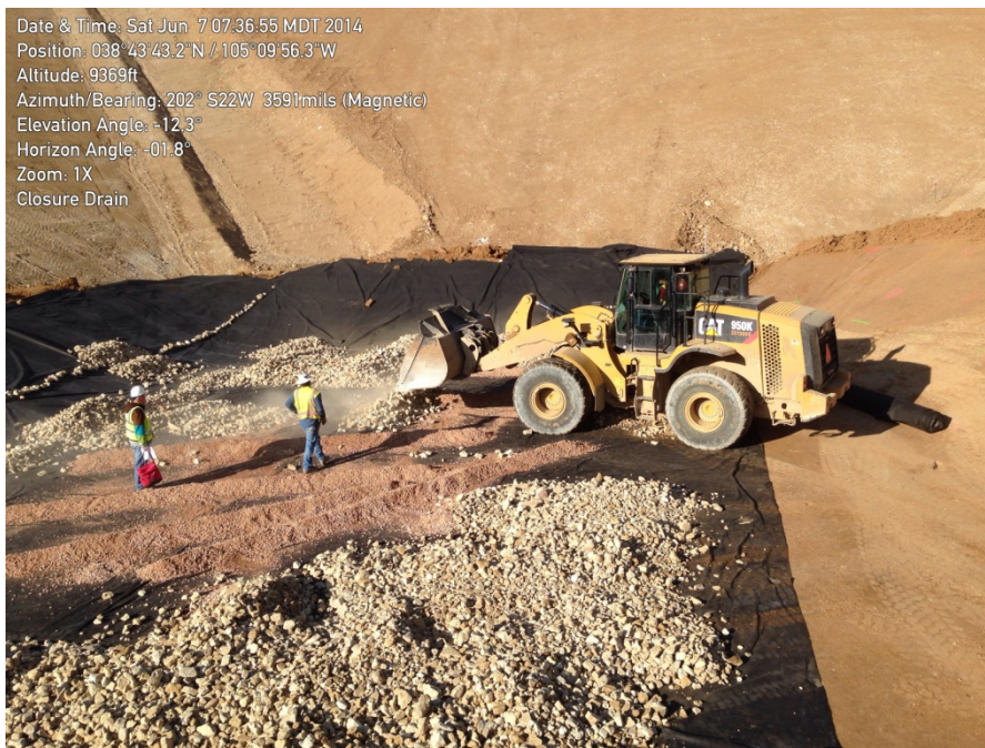
Photo 3 Placement of Non-woven Geotextile and PVC Drains
