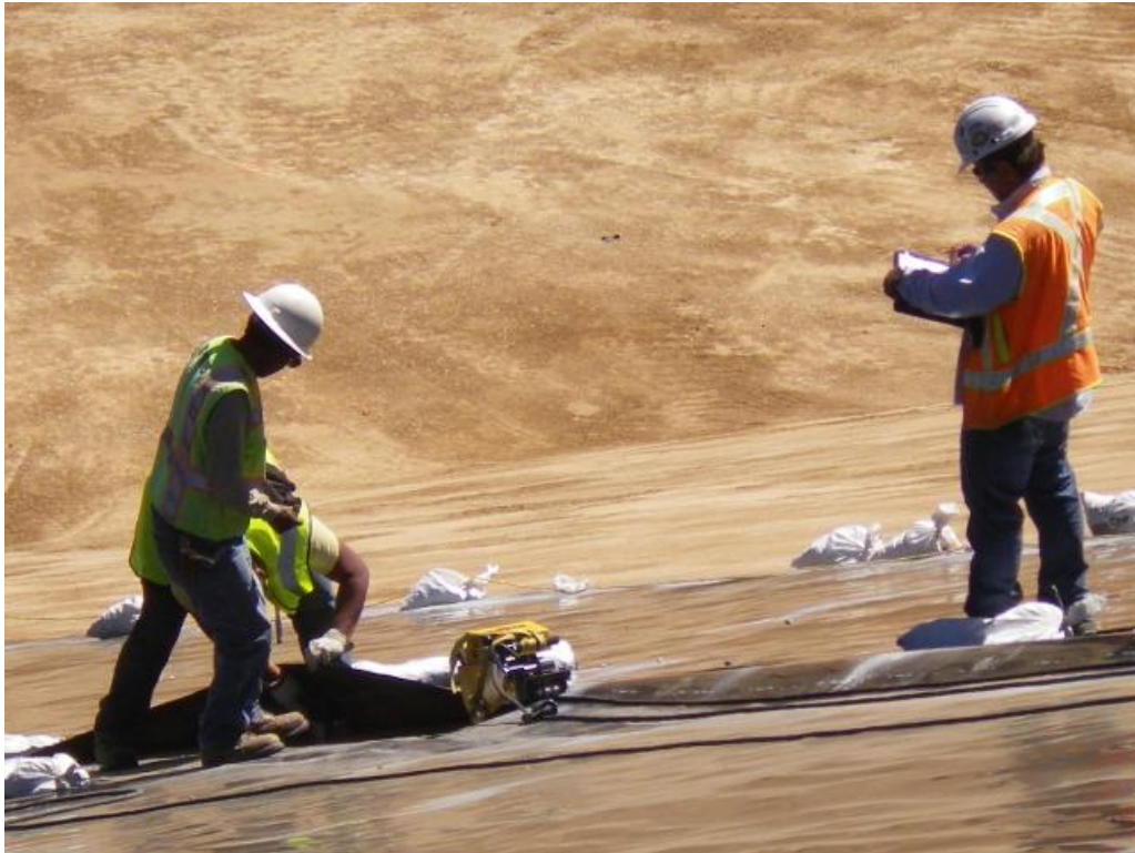
Photo 3: Fusion welding the geomembrane.
