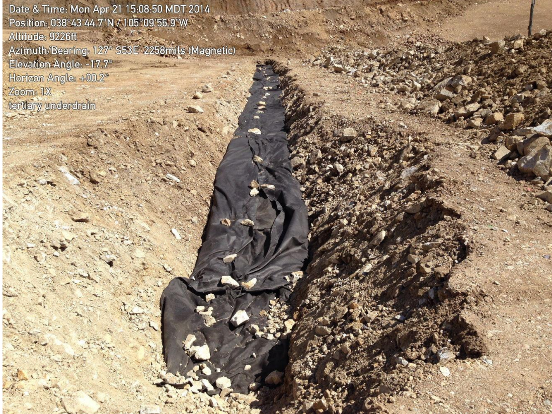
Photo 1: Tertiary underdrain on the PSSA floor.
