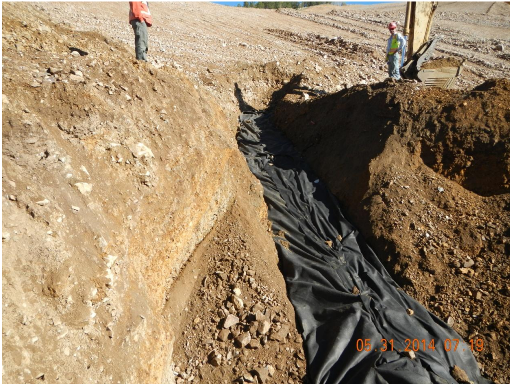
Photo 1 Secondary Underdrain Installation near Station A6+00
