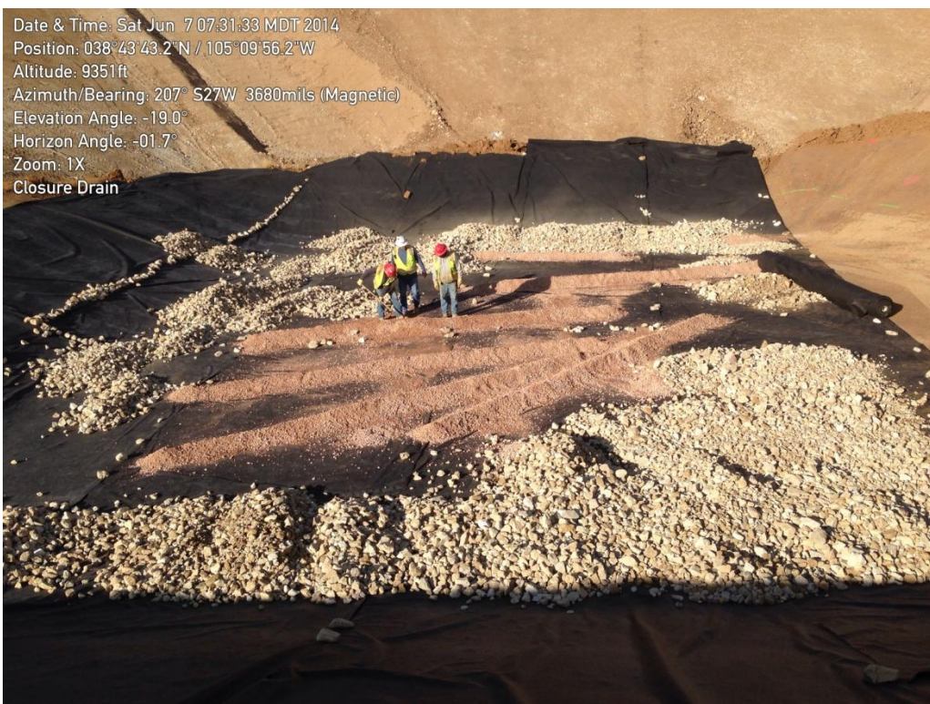
Photo 4: Drain Cover Fill Placement over the Leak Detection Fill and Geotextile in the Closure Drain Area
