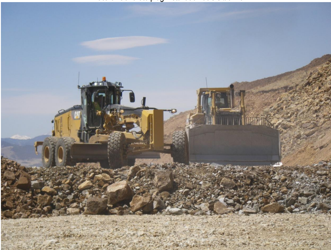
Photo 4: Fill placement at the Buttress fill Area
