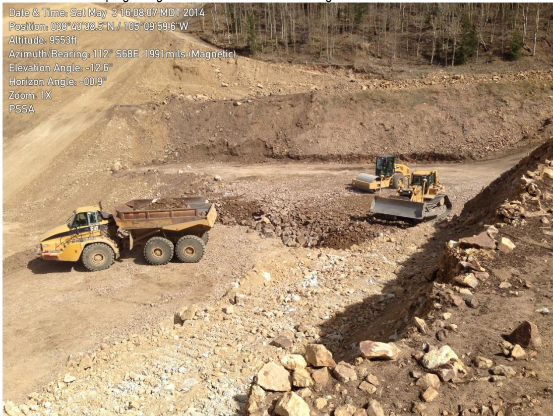
Photo 4: Fill placement at the PSSA Embankment.
