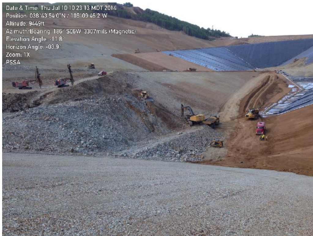
Photo 2: Production drilling and shot rock removal.
