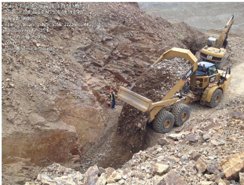
Photo 2: UG#6446, backfilling shaft with coarse shaft backfill.
