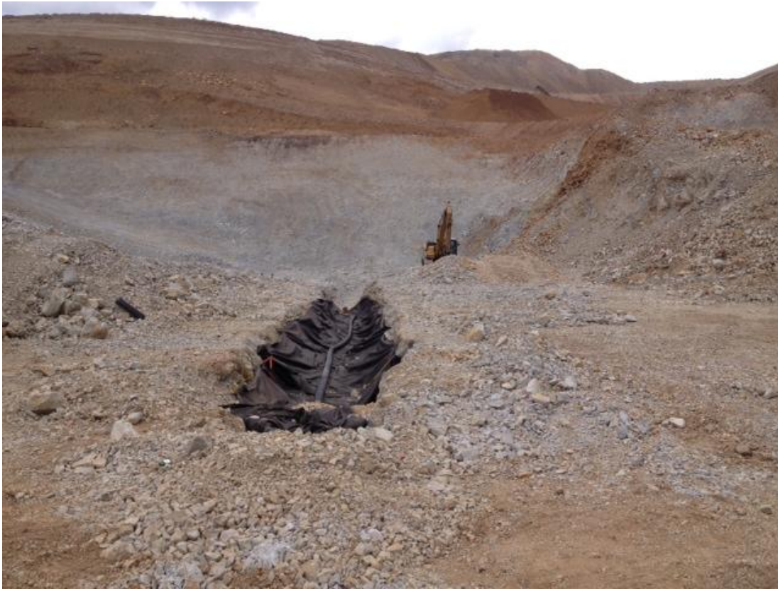
Photo 3: Primary underdrain installation on the north PSSA floor
