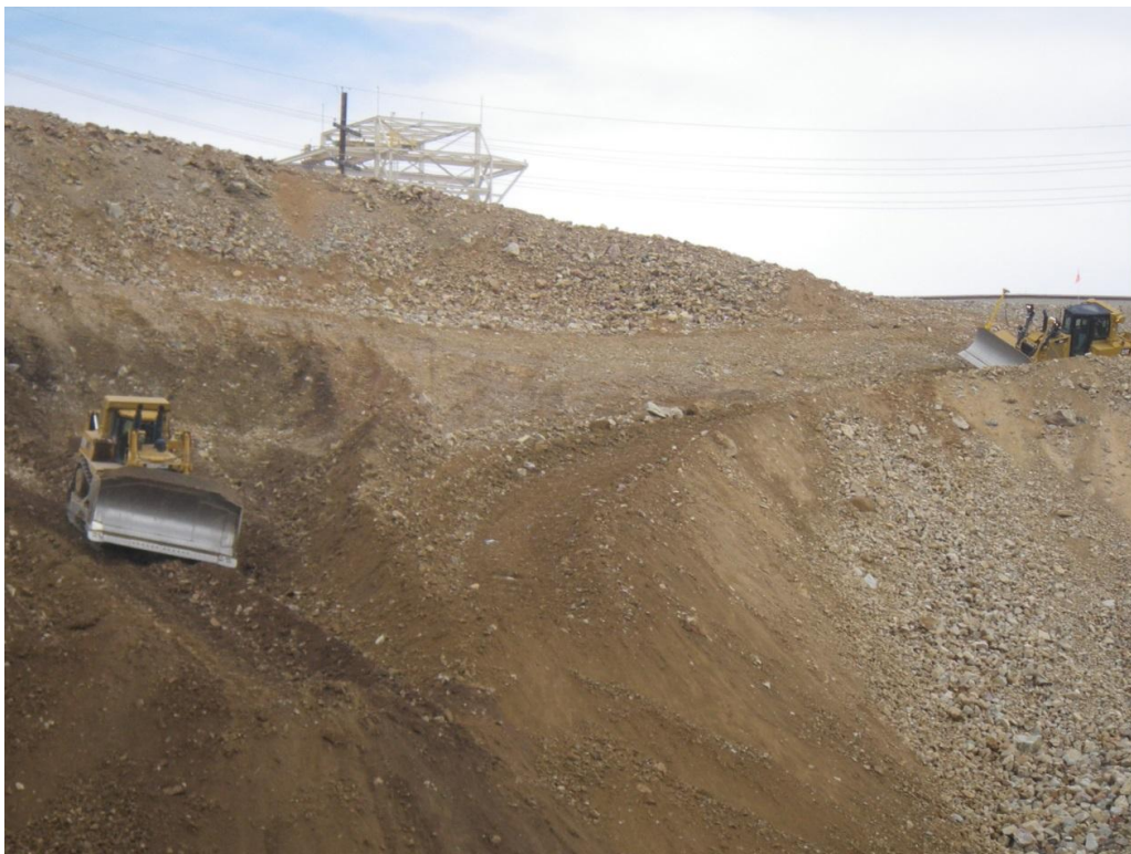
Photo 2 Slope Grading Below the Ball Mill Platform
