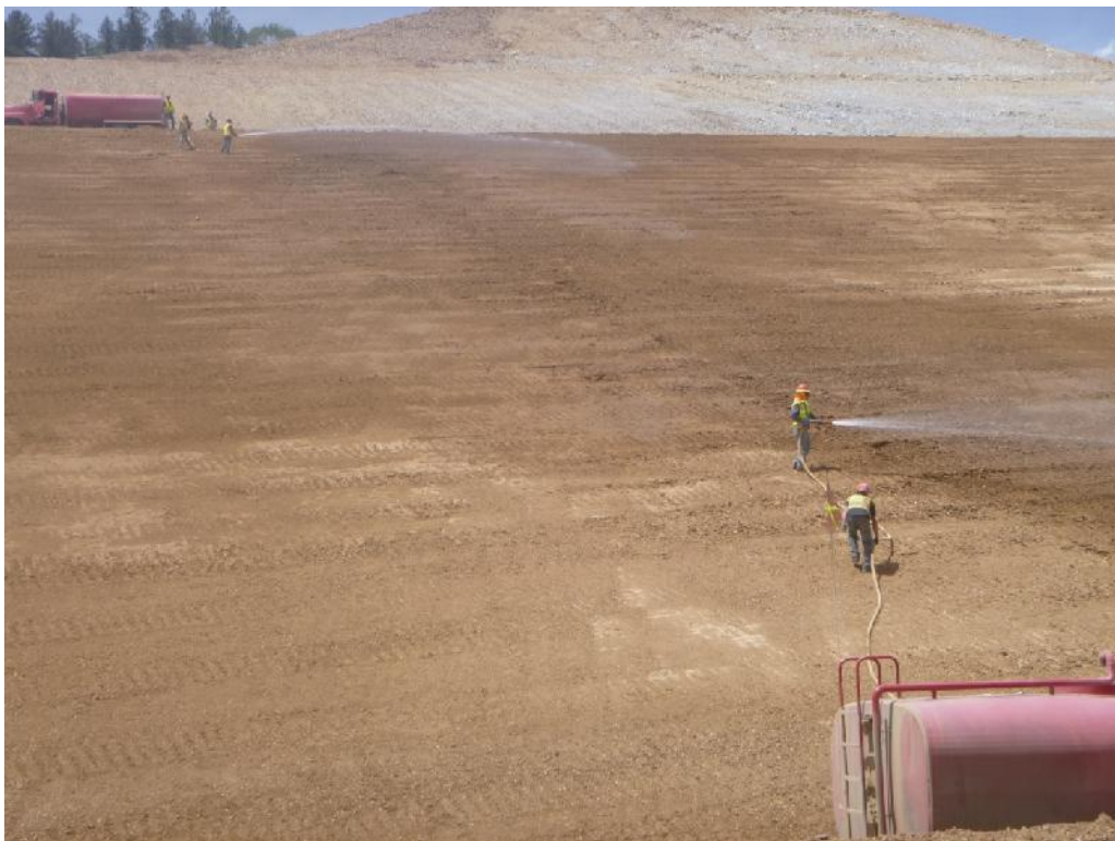
Photo 4: Moisture conditioning clay lined slopes.
