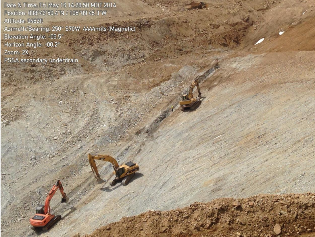
Photo 1: Trenching for secondary underdrain below station A14+00 in the PSSA.
