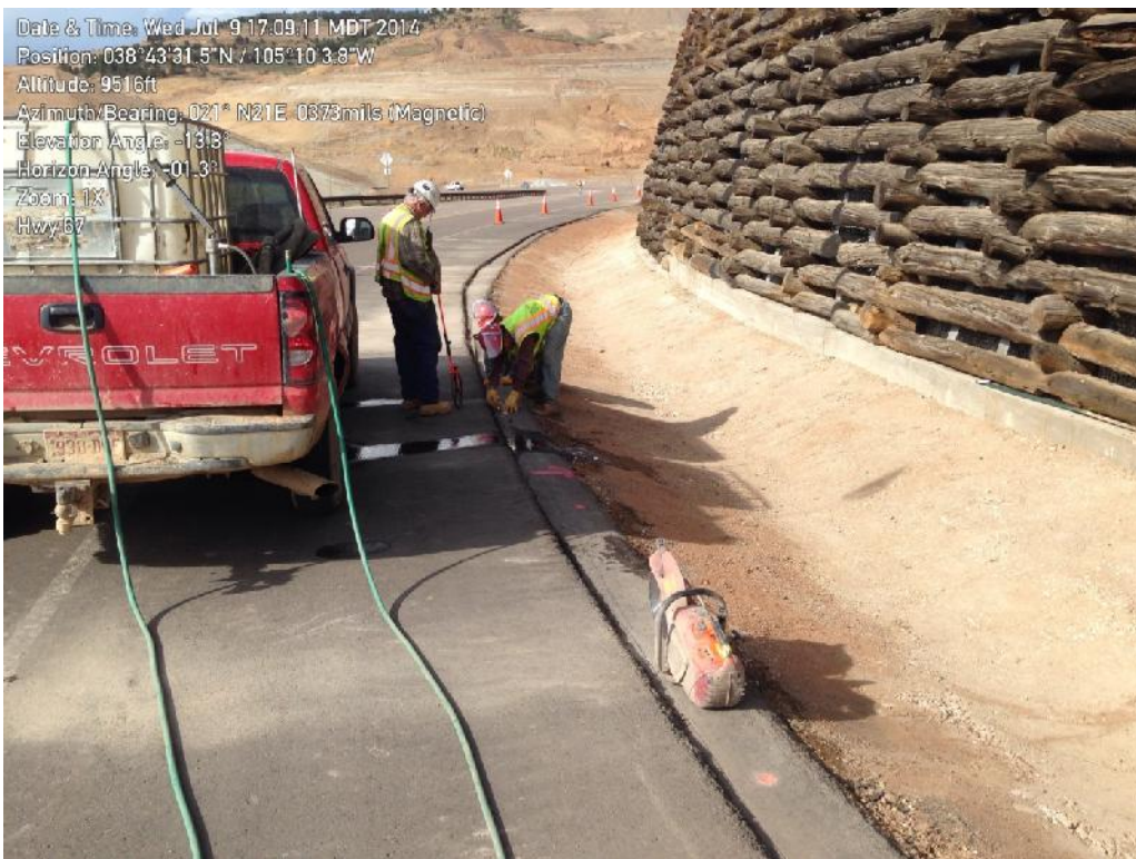
Photo 4: Preparing Highway 67 drainage channel.
