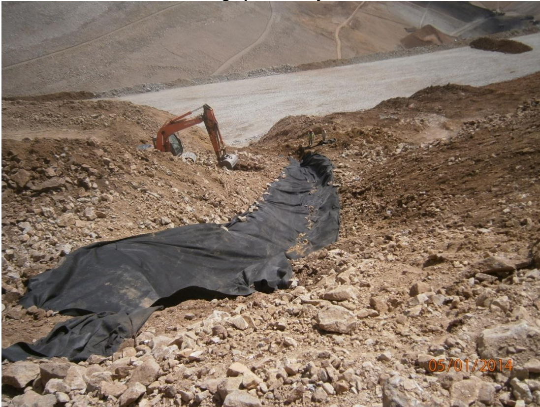
Photo 1: Secondary underdrain installation adjacent to Dump 4.
