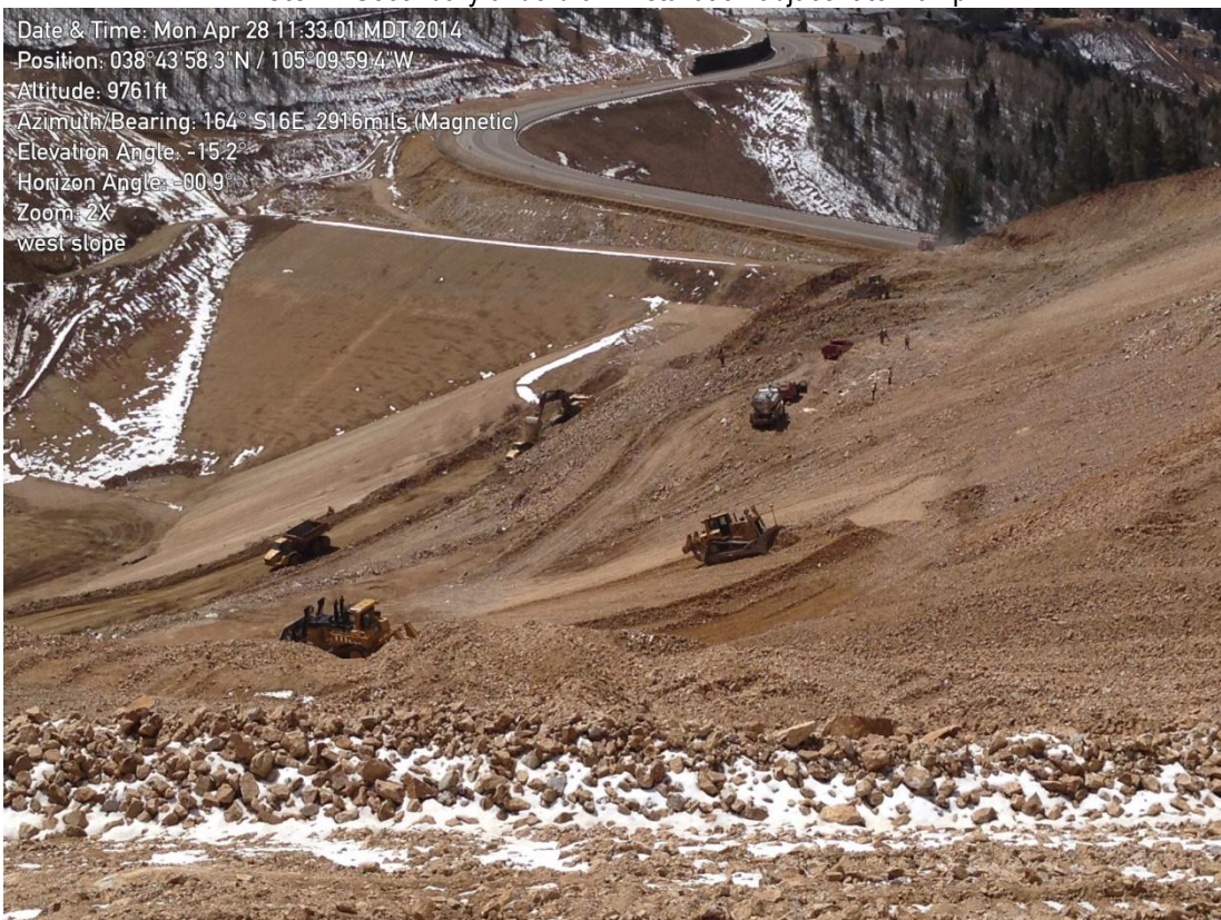
Photo 2: Fill placement, cut activities, and blasting preparation at the western VLF slope between the C and E benches.
