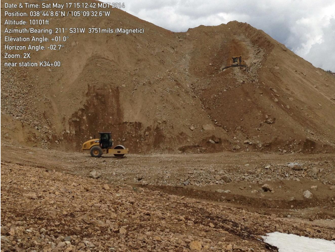
Photo 3: Fill compaction near station K34+00.
