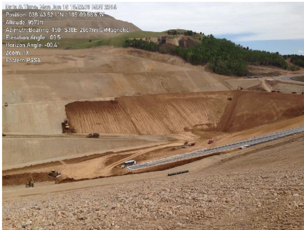
Photo 1: Soil Liner Fill Placement on the PSSA Slopes.
