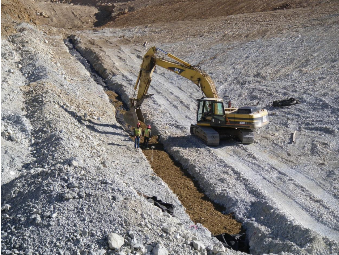
Photo 1: Secondary underdrain installation below station A14+50.
