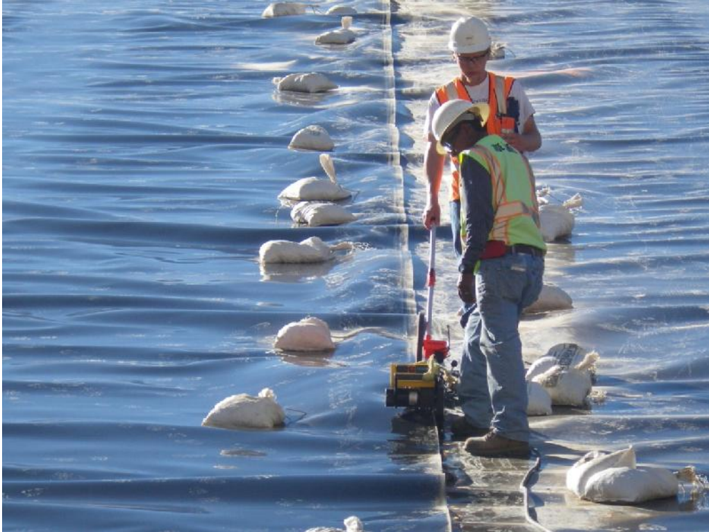
Photo 3: Geomembrane fusion welding.
