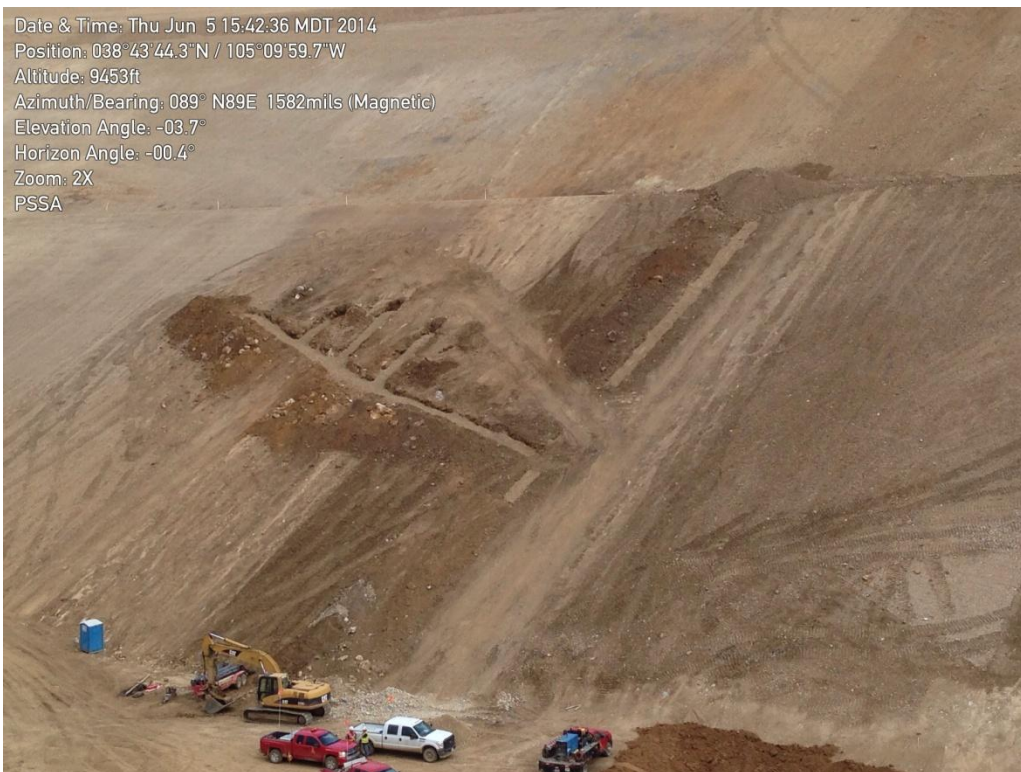
Photo 2: Tertiary Underdrain, Spurs, and Laterals on the East Slope of the PSSA.
