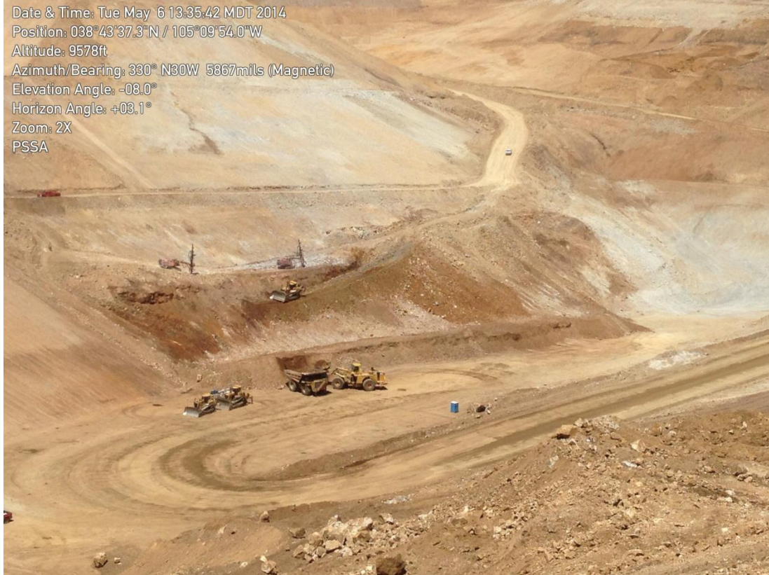
Photo 1: Slope grading, production drilling, and cut removal downslope of stations A7+00 to A12+00.
