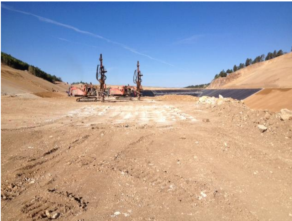
Photo 4: Production drilling near B16+00.
