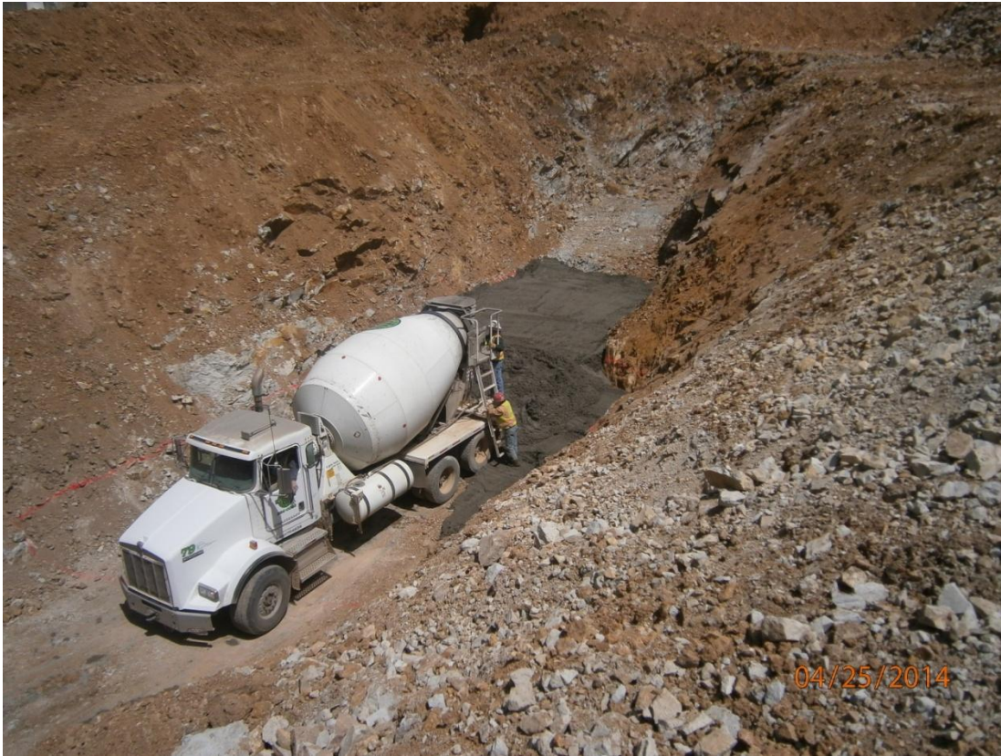
Photo 3: Concrete plug installation at UG #6273.
