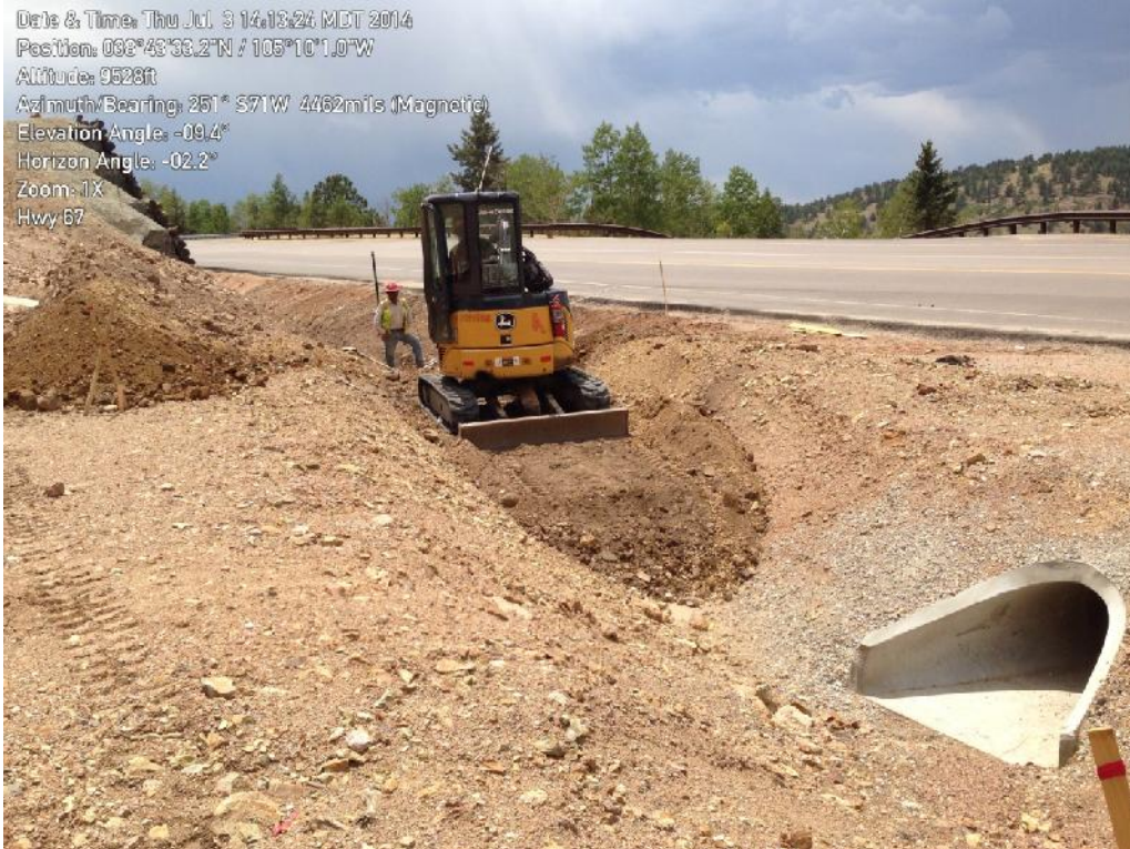
Photo 3: Highway 67 drainage channel preparation.
