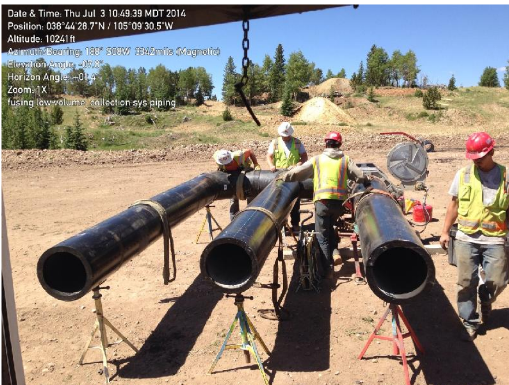
Photo 4: Low Volume Solution Collection System Manifold HDPE pipe butt fusion.
