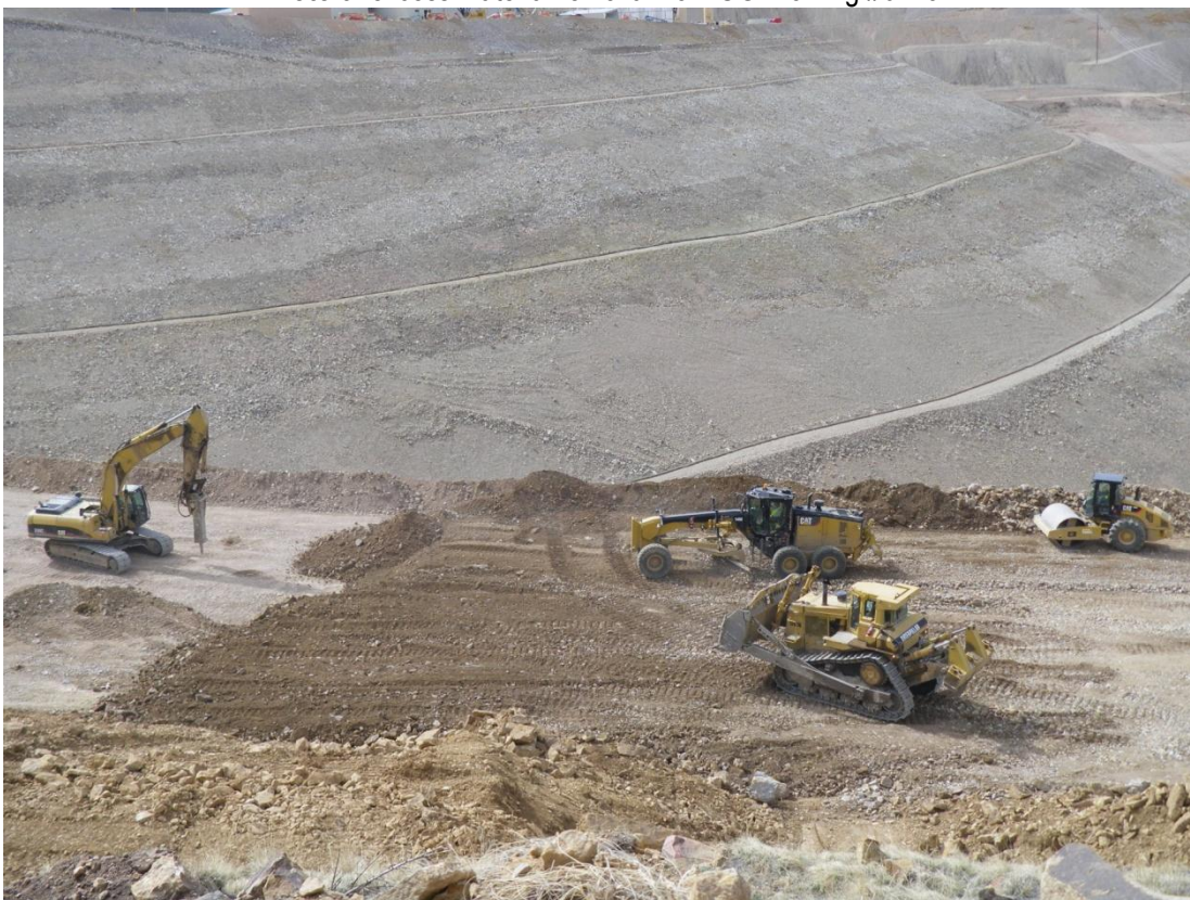
Photo 4: Fill placement at the ADR haul road fill area.
