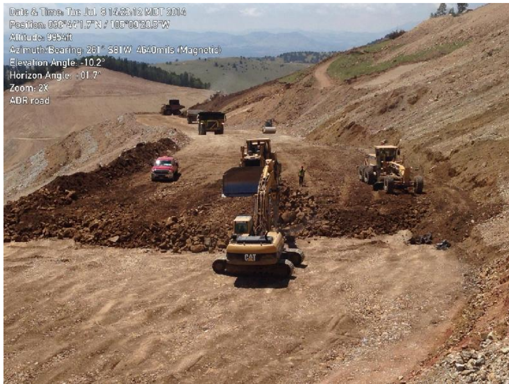
Photo 1: Structural Fill on ADR haul road.
