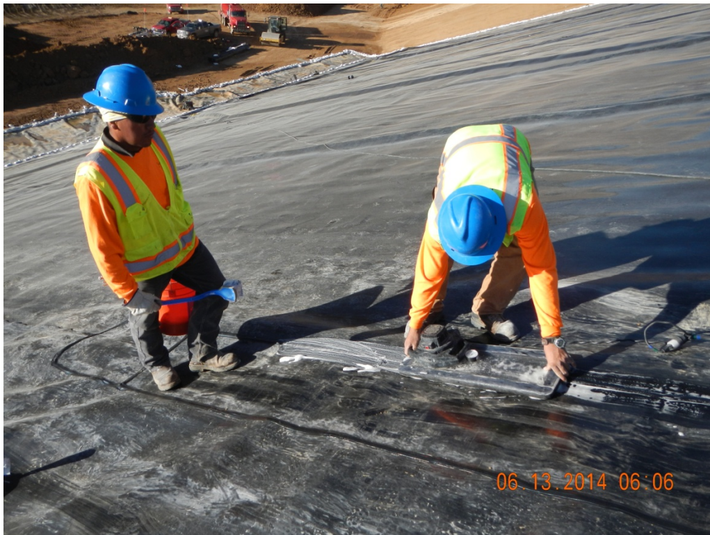
Photo 3: Vacuum testing extrusion weld during liner repairs.
