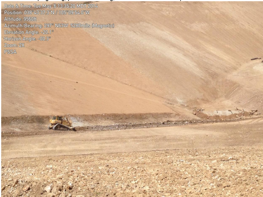
Photo 2: A Cat GPS D6 dozer shaping the trench for the Low Volume Solution Collection (LVSC) riser piping in the PSSA.
