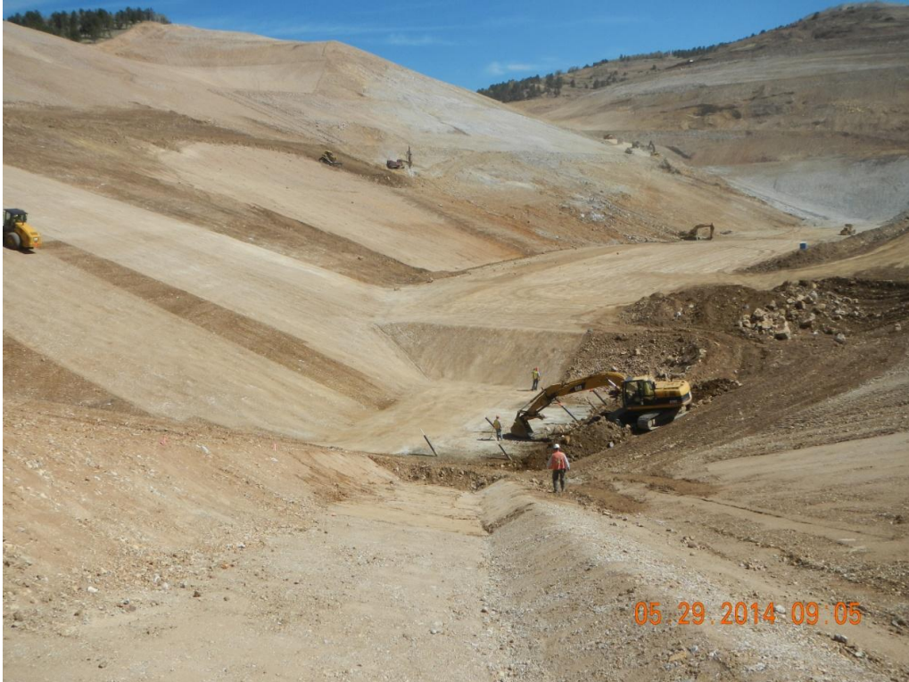
Photo 3 Progress at the PSSA and Closure Drain Subgrade Preparation
