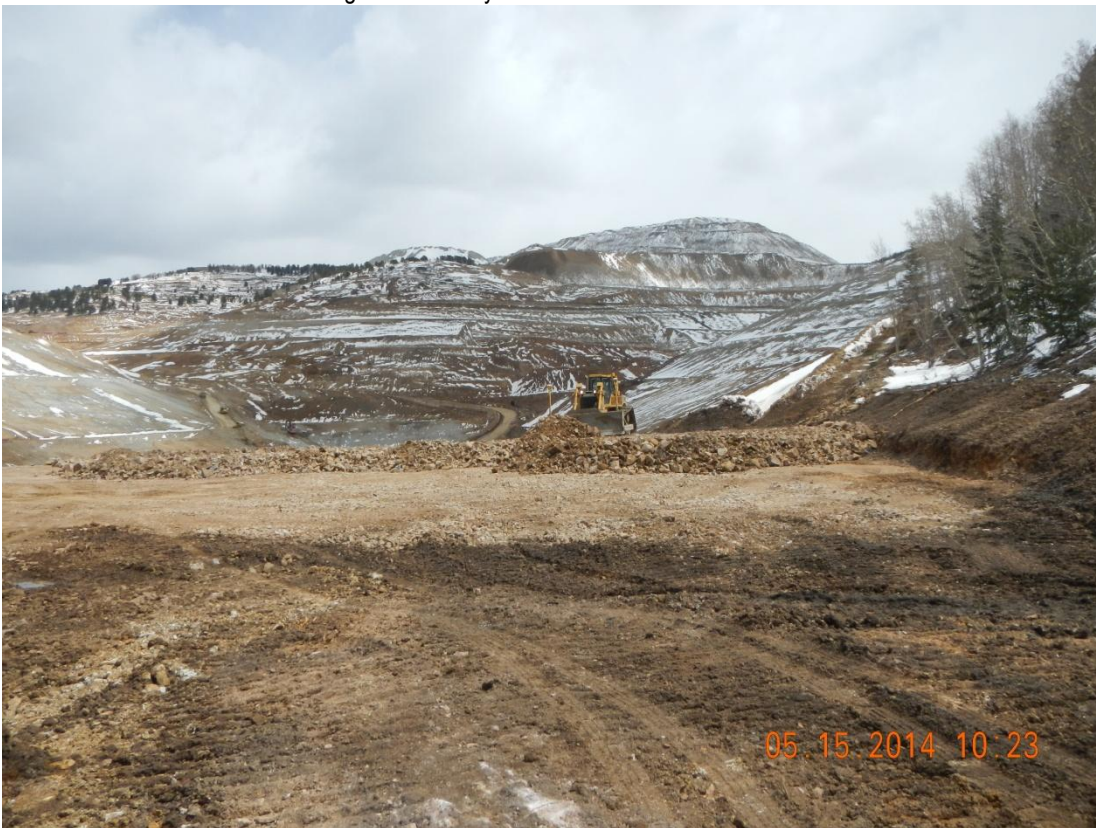
Photo 2: Fill placement at PSSA embankment fill area.
