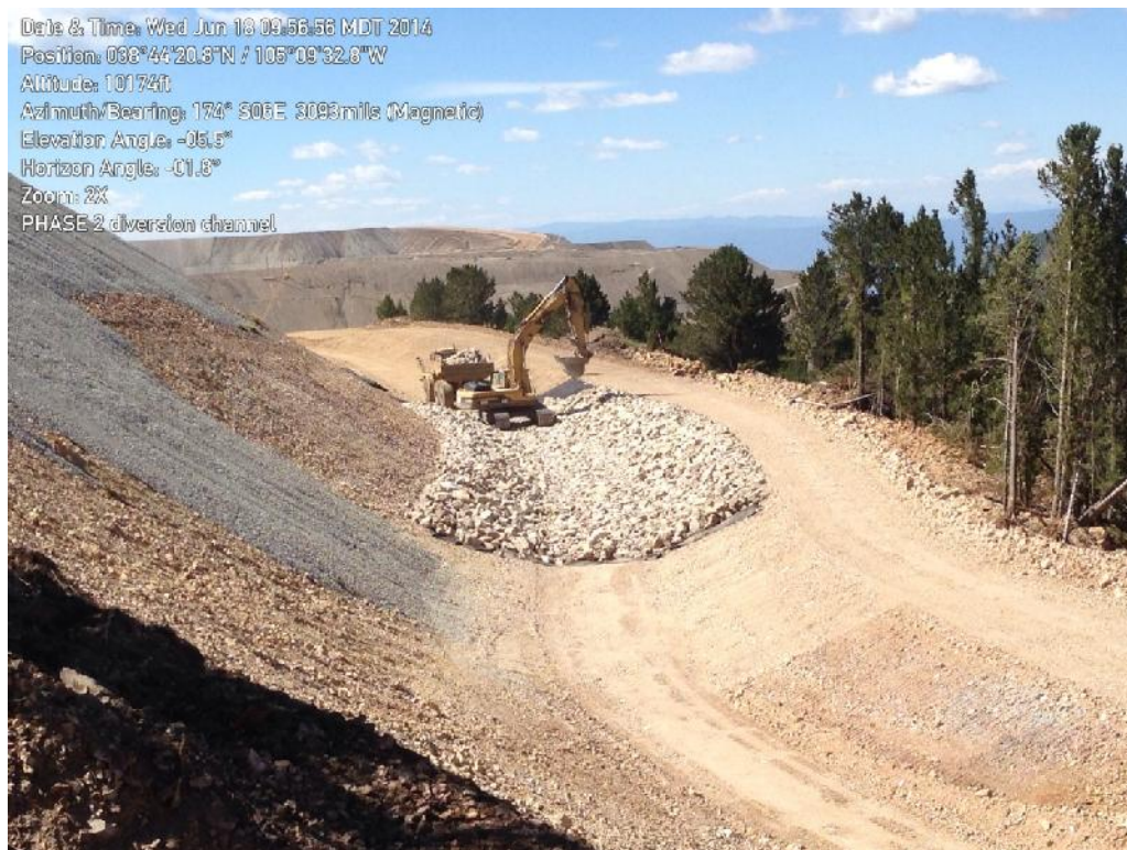
Photo 2: Rip rap placement in the Phase 2 diversion channel.
