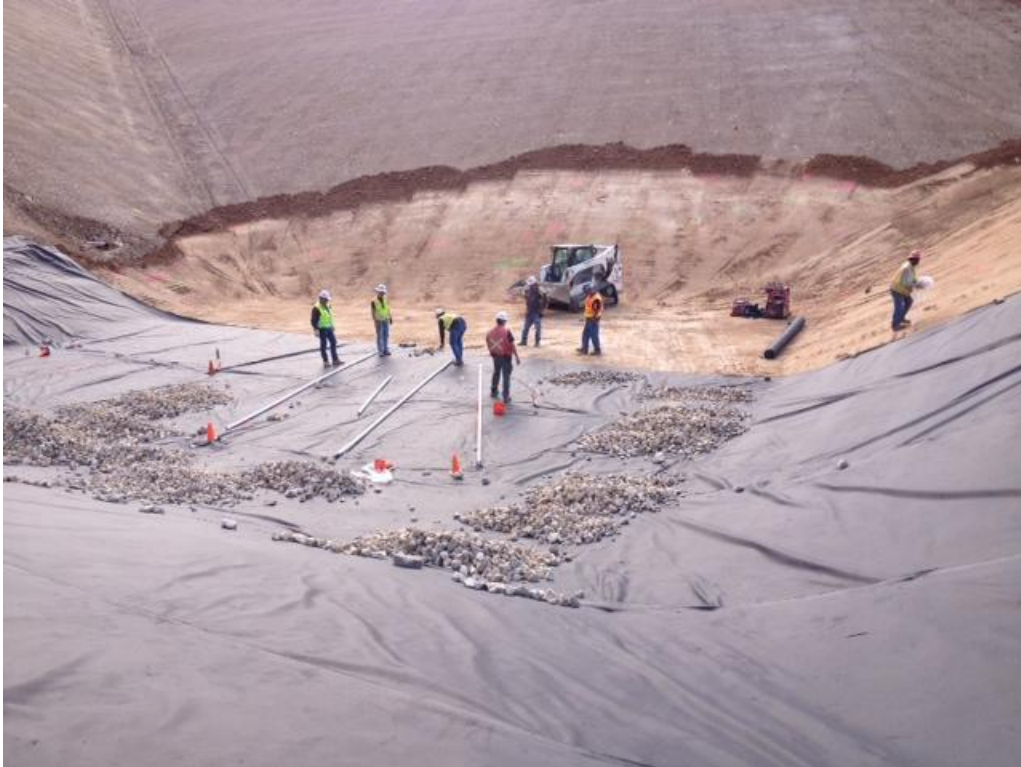
Photo 3: Geotextile and 2-inch well screen placement at the Closure Drain.
