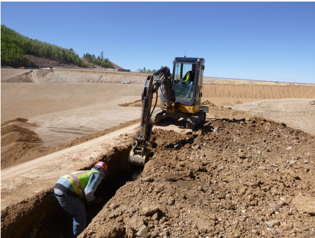
Photo 2: Excavating anchor trench.
