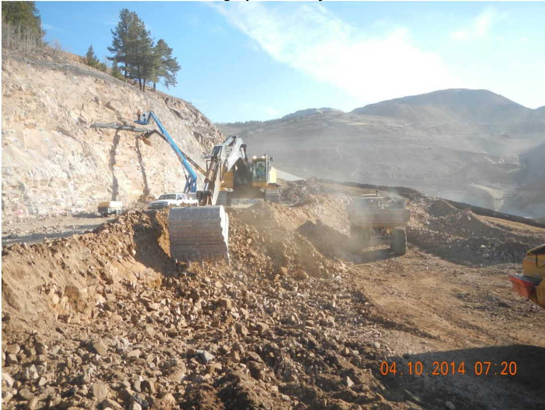
Photo 1: Excavation at the \frac{1}{2} :1 slope.
