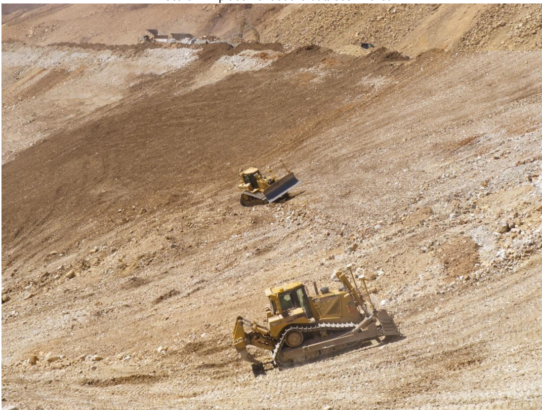
Photo 4: Slope grading down slope from stations H22+00 to H30+00.
