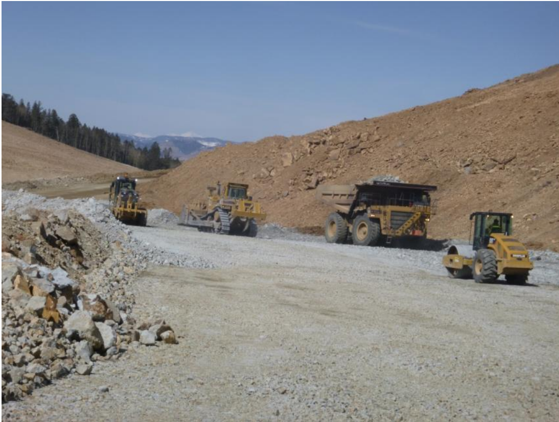
Photo 3: Structural fill placement.
