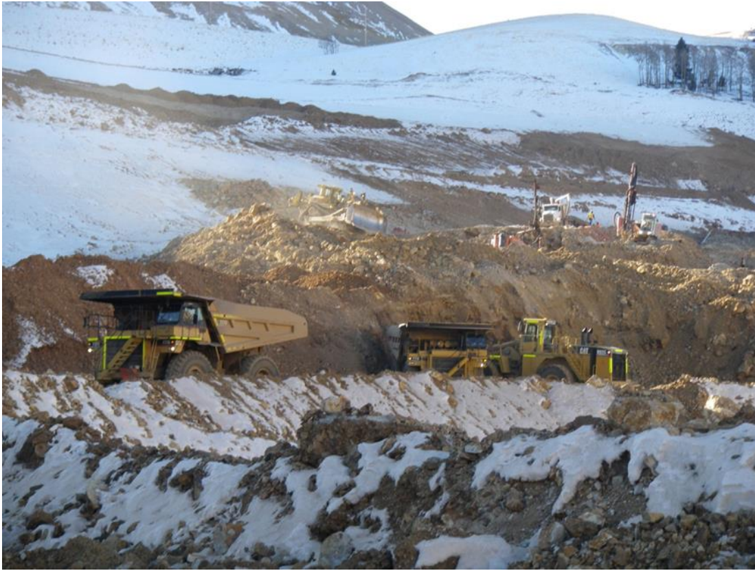
Photo 1: Loading out fill from under the historic crib wall and production drilling.
