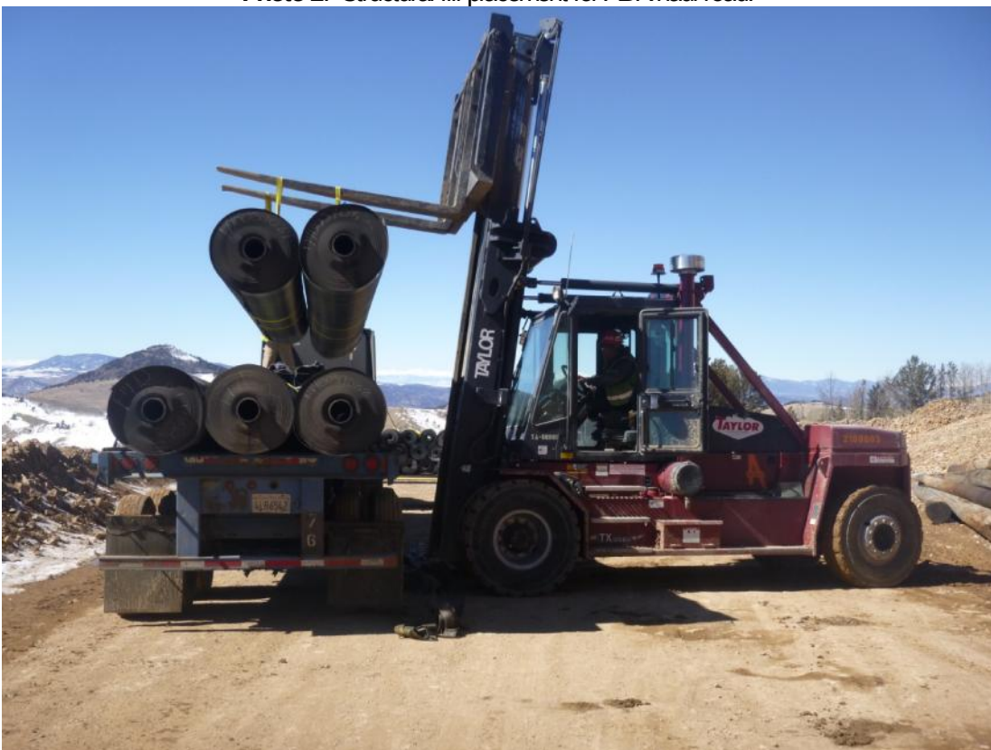
Photo 2: Liner delivery (100-mil LLDPE SSMS).
