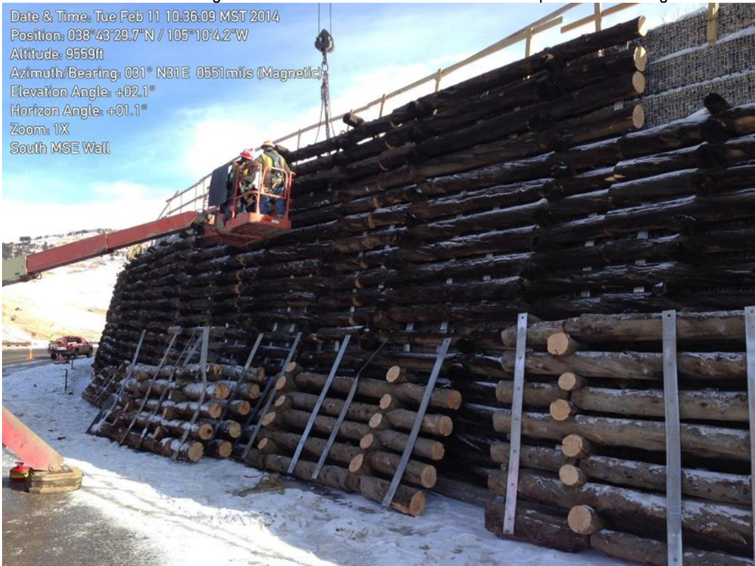
Photo 2: Timber panel installation at the South MSE Wall.
