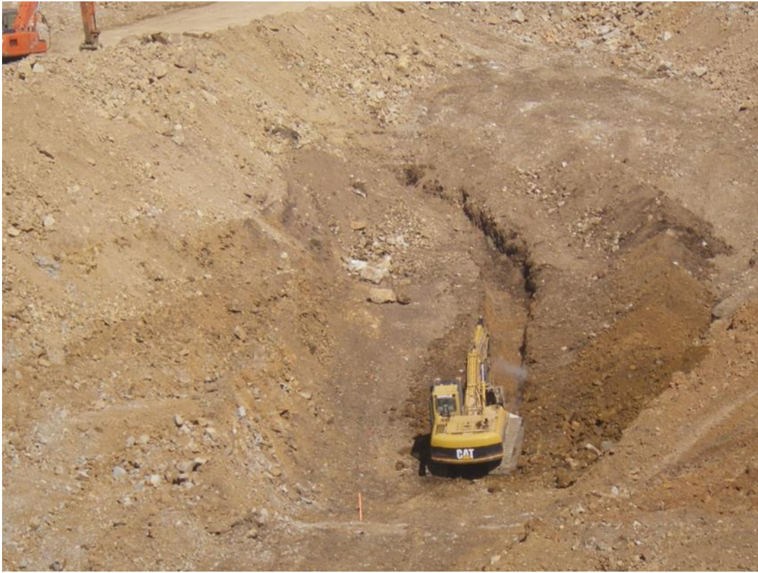
Photo 3: Excavating a trench for secondary underdrain below ADR Haul Road station 23+00.
