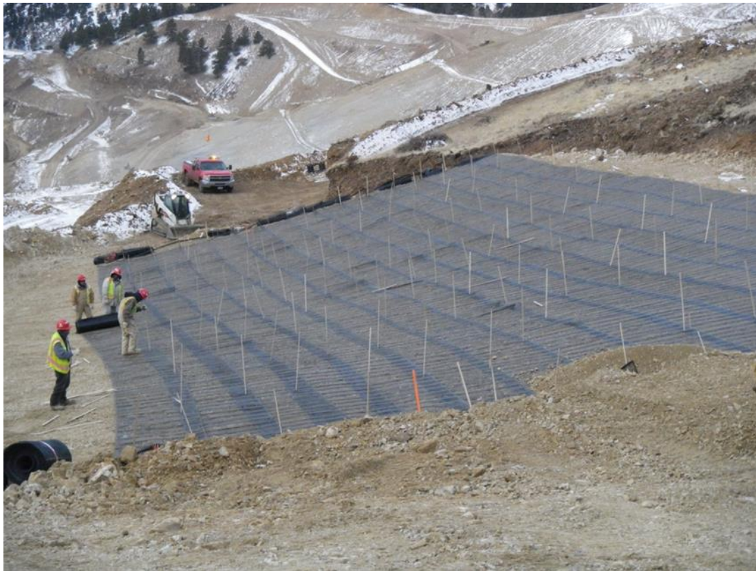
Photo 3: Placement of the final layer of geogrid at Underground Working UG 6123.
