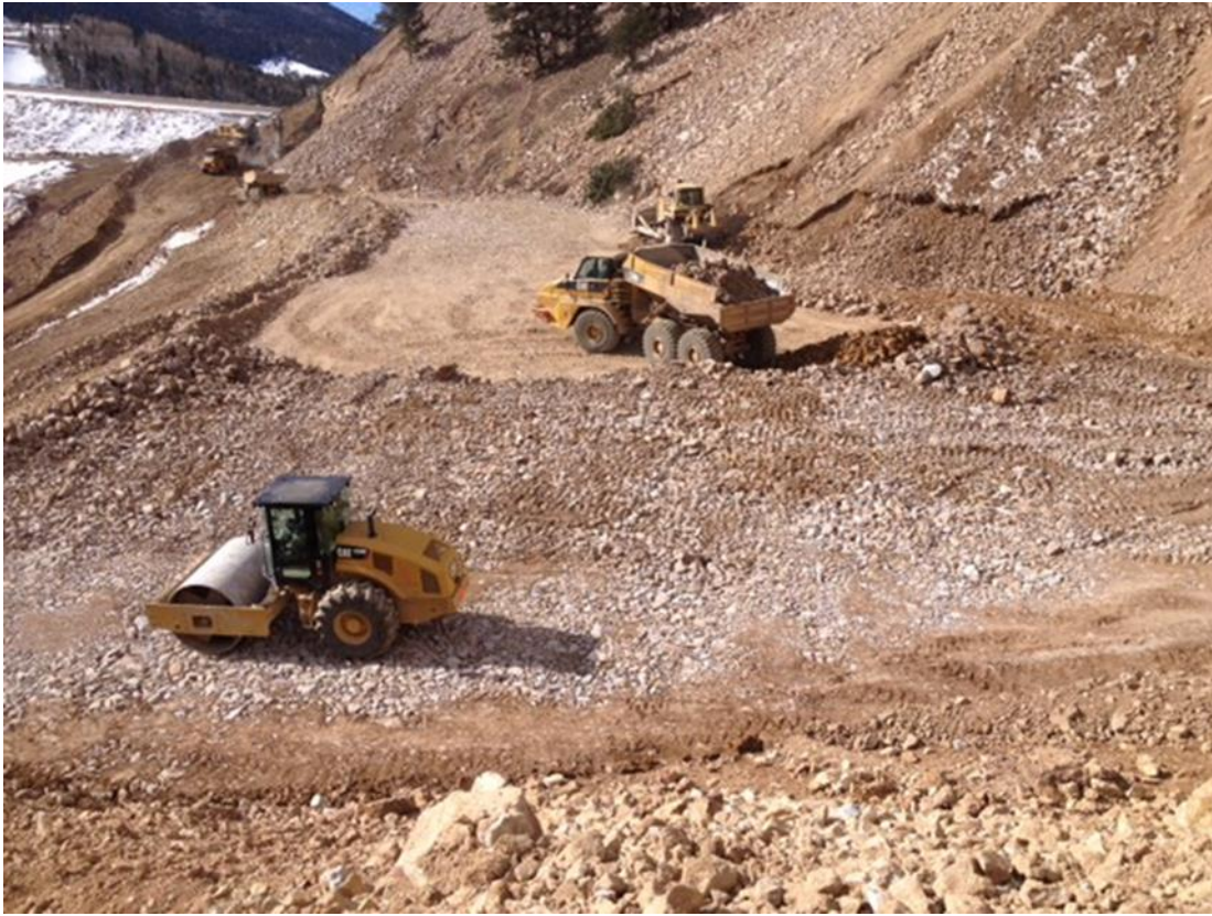
Photo 3: Fill placement near station C6+00.
