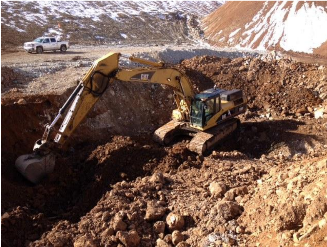
Photo 3: Shot rock removal from UG #U6273.
