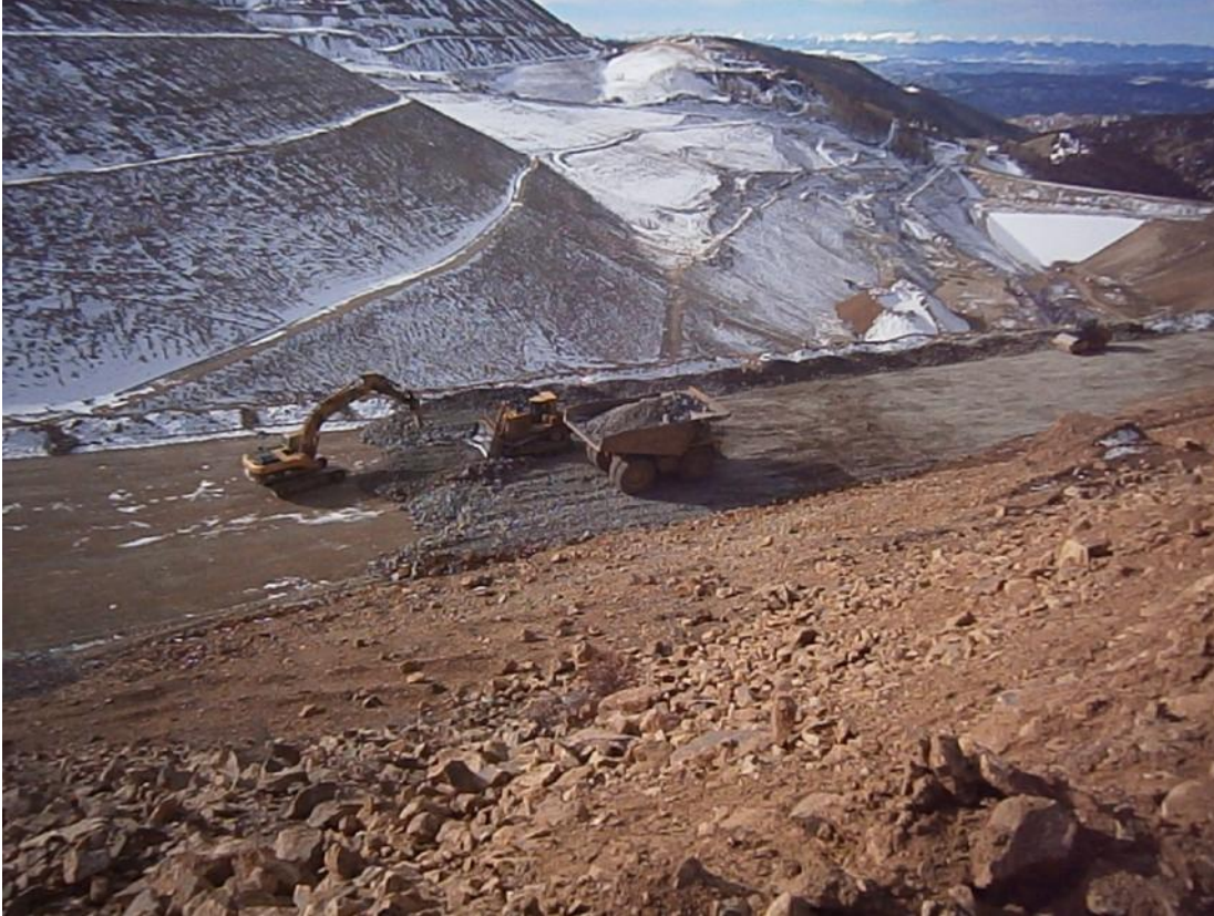
Photo 1: Structural fill placement for ADR haul road.
