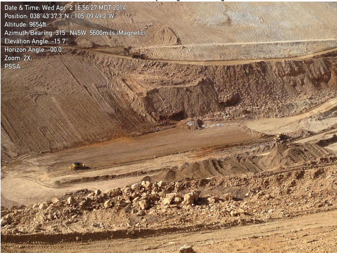
Photo 2: Rough grading on the south side of the PSSA floor.
