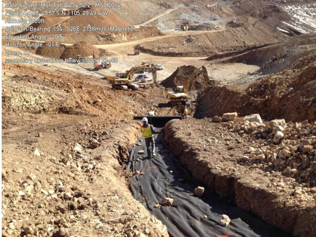
Photo 1: Secondary underdrain below ADR Haul Road station 23+00.
