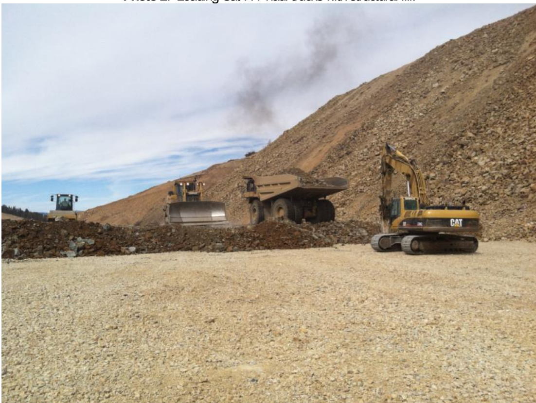
Photo 2: Structural fill placement for ADR haul road.
