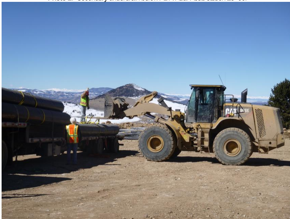
Photo 2: Liner delivery (100-mil smooth LLDPE).
