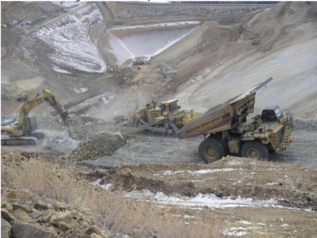
Photo 4: Fill placement at the ADR Haul Road.
