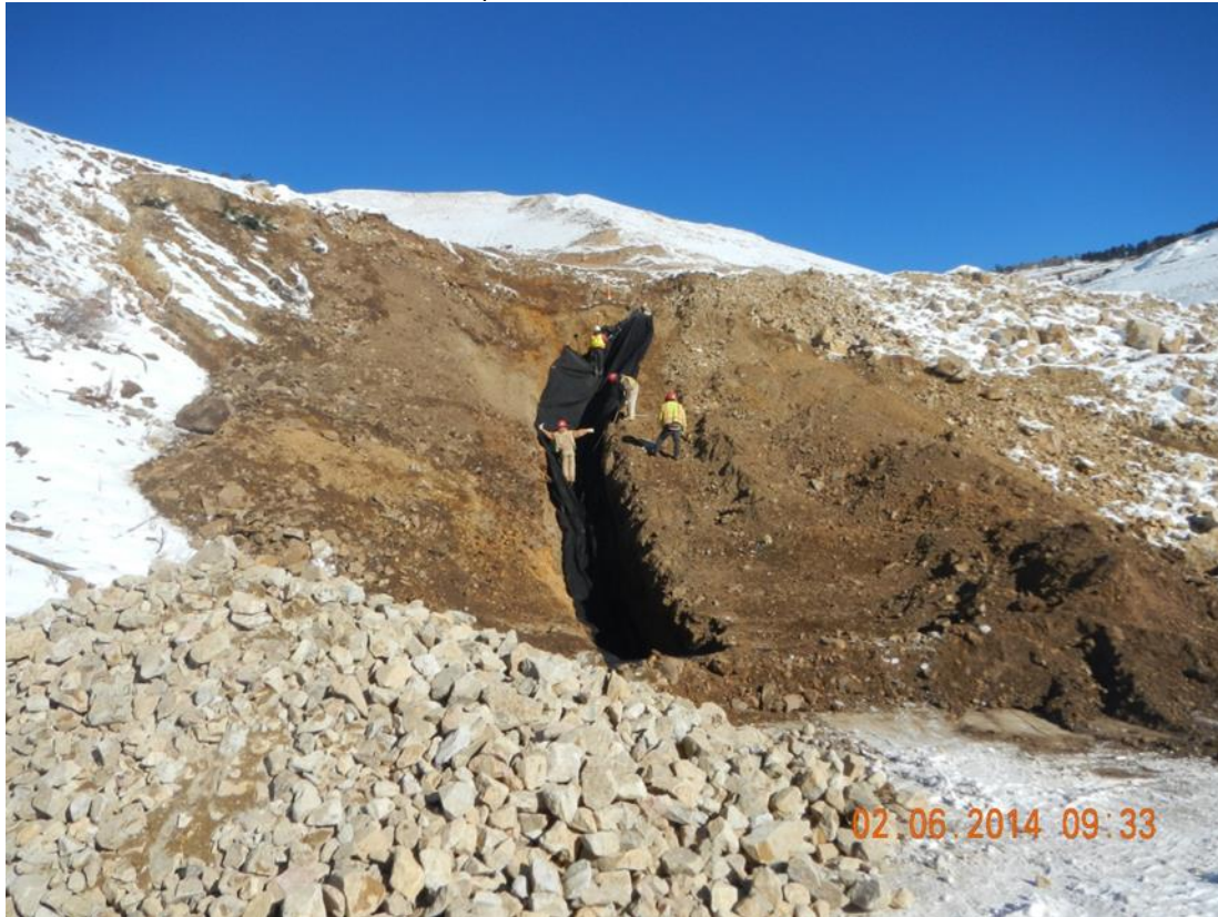
Photo 3: Secondary underdrain installation near station A6+00.
