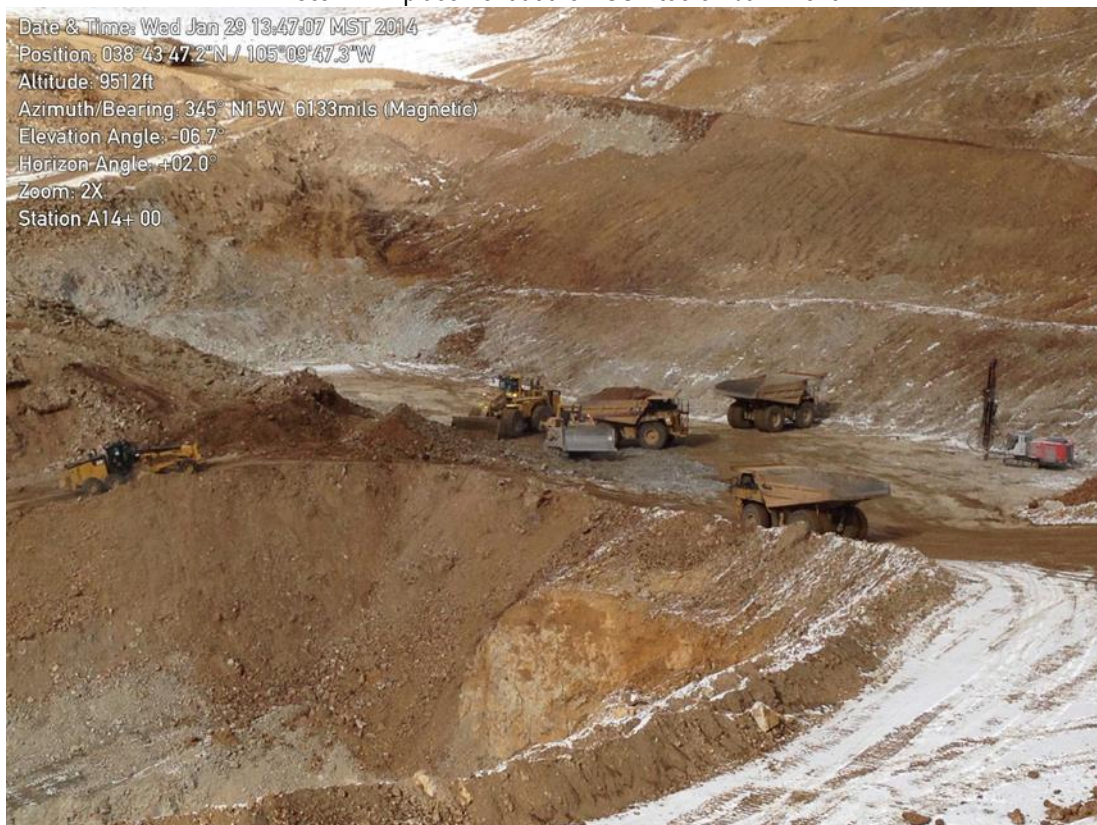
Photo 2: Cut removal near station A14+00.
