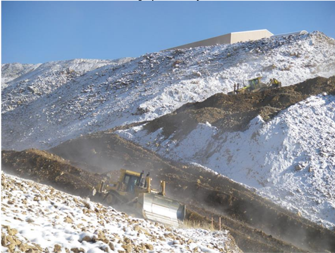
Photo 1: Cut and fill operations east of the Phase 2 Diversion Channel adjacent to Dump 4.
