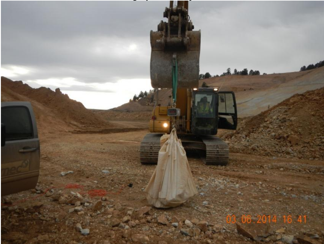
Photo 1: Large rock gradation on Structural Fill.
