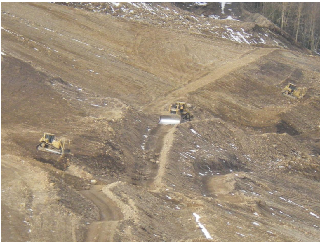
Photo 4: Slope grading near stations DD6+00 to DD10+00.
