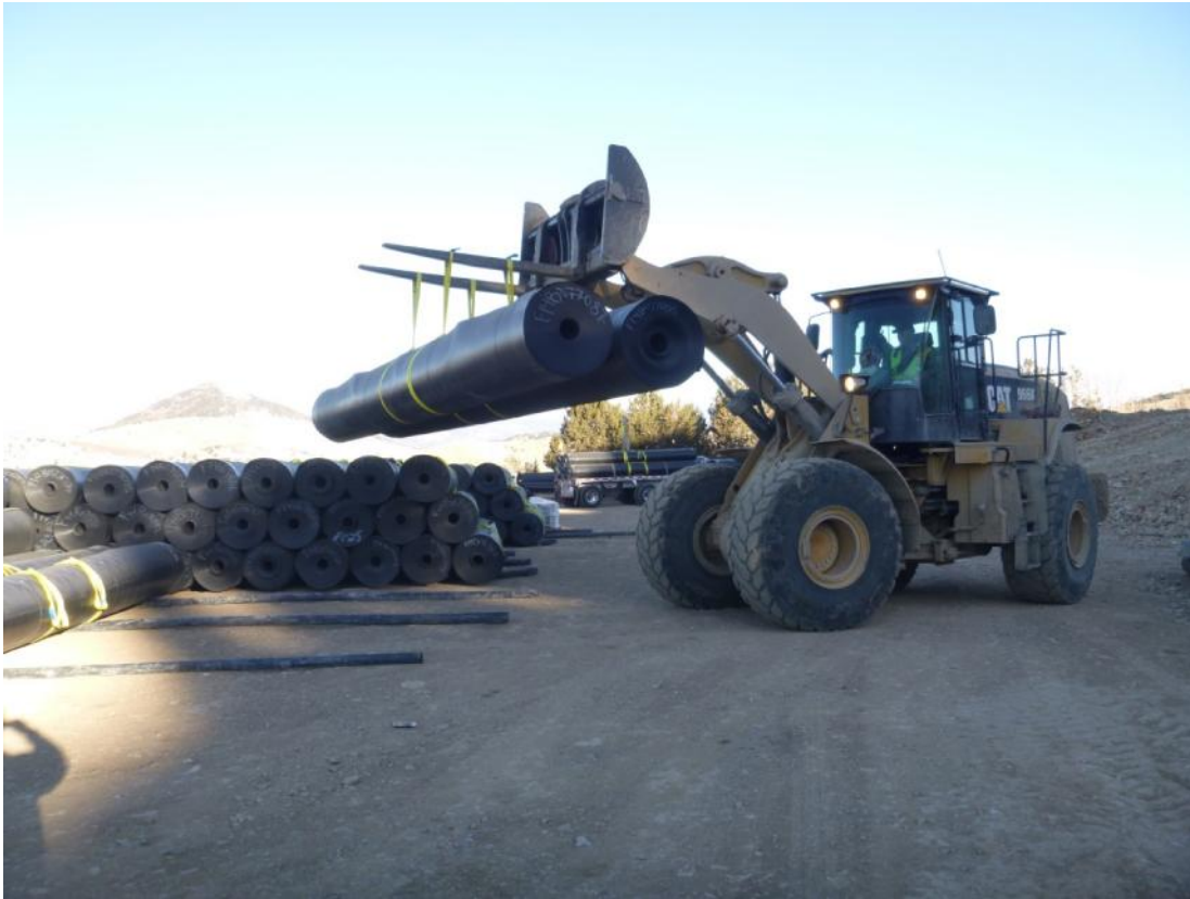
Photo 3: Liner delivery (100-mil LLDPE SSMS).
