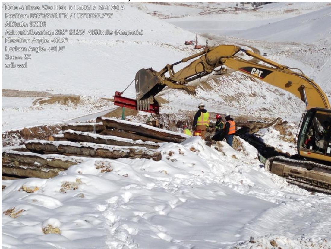
Photo 4: Historic crib wall dismantling.
