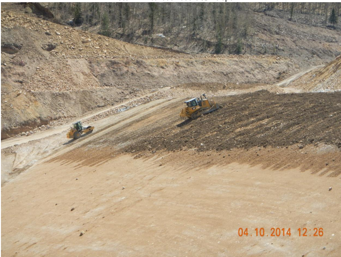
Photo 2: Slope grading at the PSSA.
