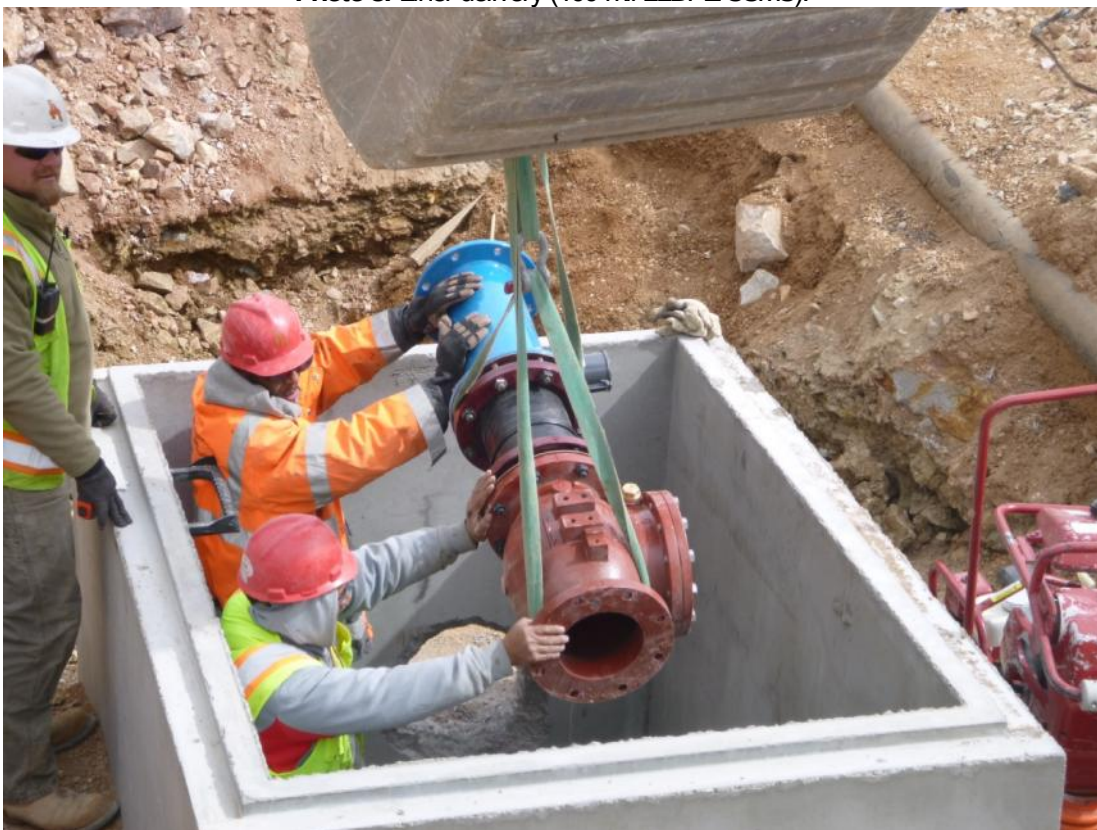
Photo 4: Installing precast manhole vault, flowmeter and valve at water stand pond tie-in.
