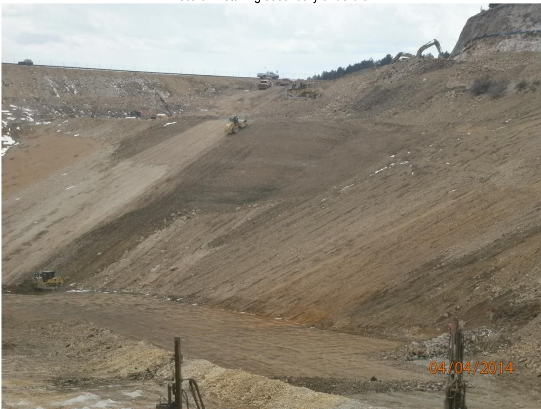
Photo 4: Subgrade finish grading and compaction at the PSSA.
