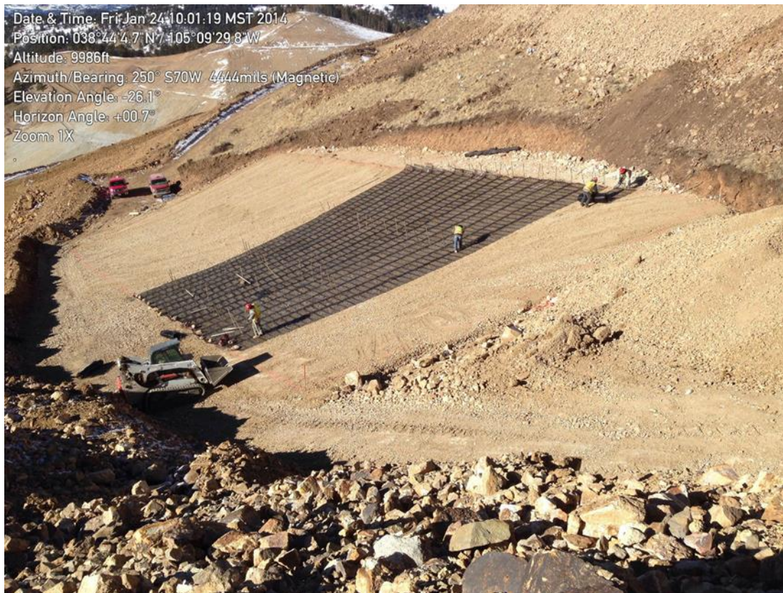
Photo 3: Placement of the second layer of geogrid at Underground Working UG 6123.
