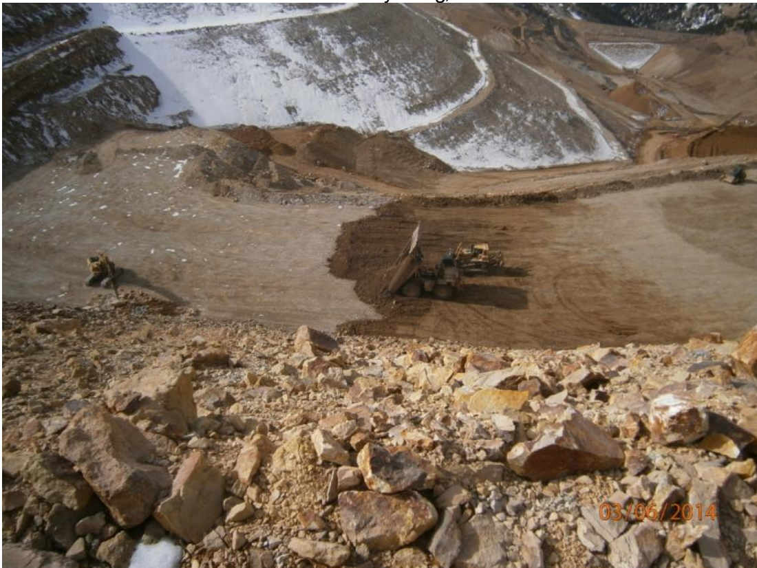
Photo 4: Fill placement at the buttress fill.
