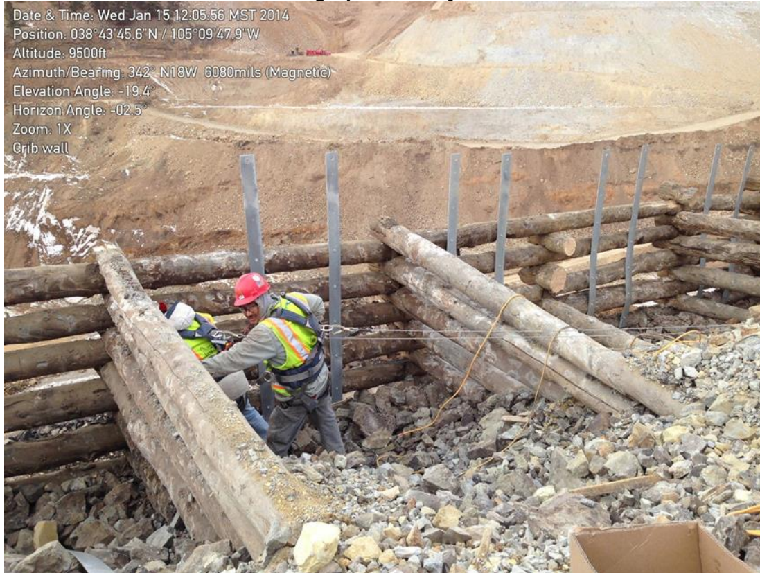
Photo 1: Historical Crib Wall dismantling.
