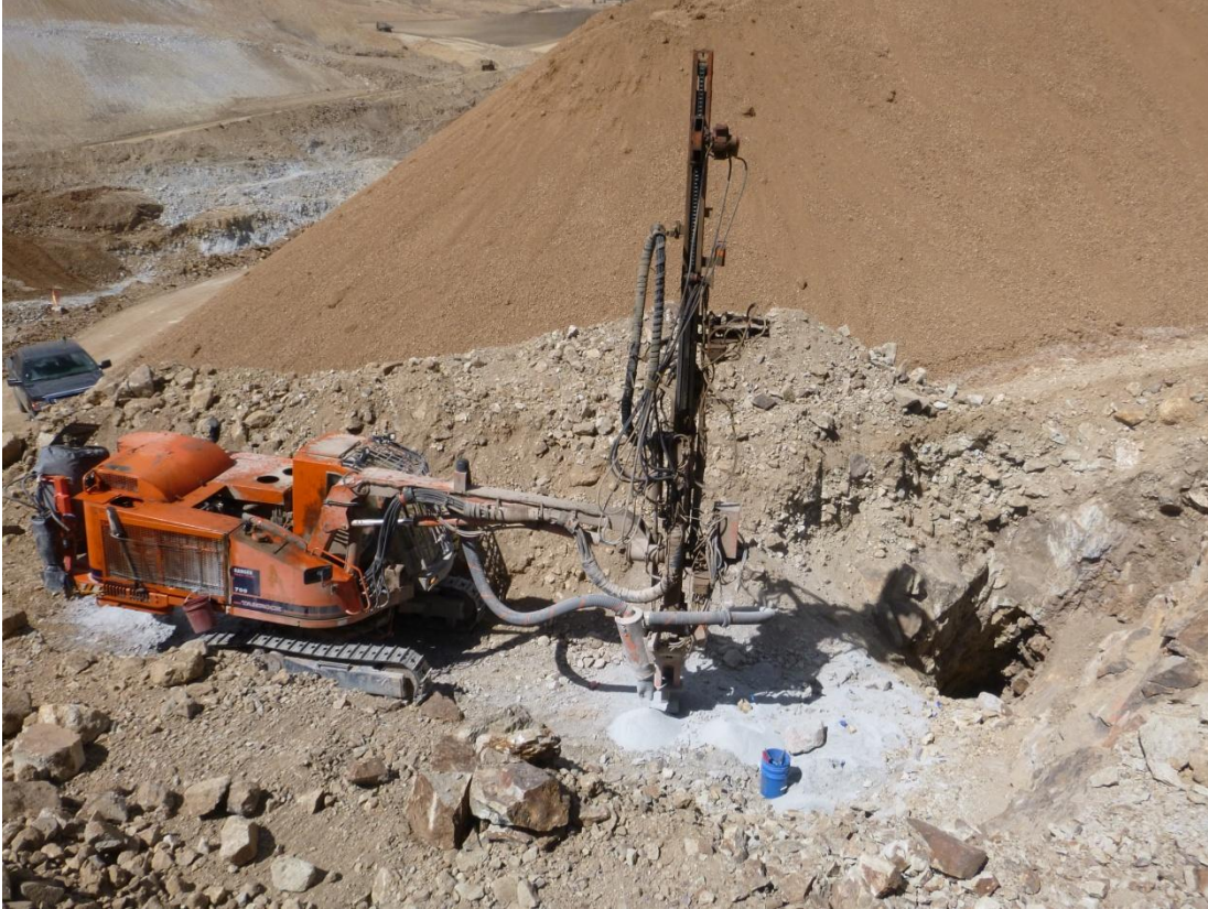
Photo 1: Confirmatory drilling at UG working #U6318.
