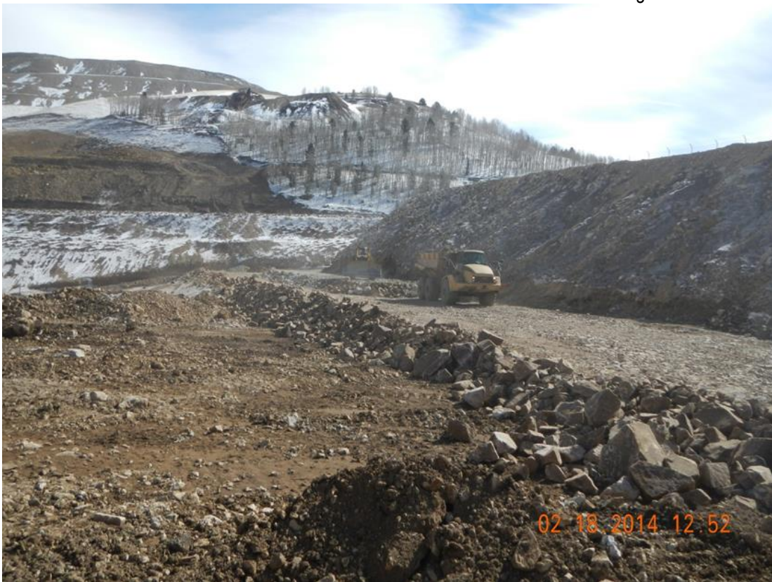
Photo 2: Fill placement at the PSSA toe berm embankment.
