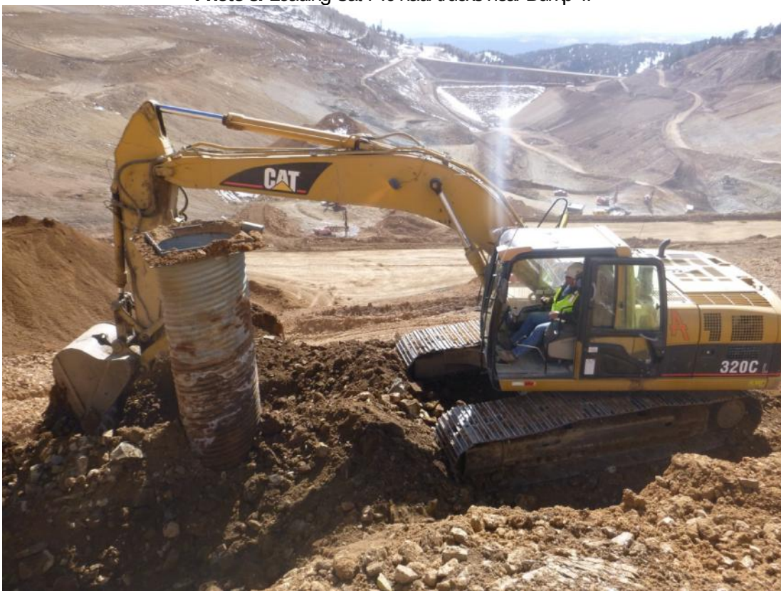
Photo 4: UG#6153; removing CMP, prepping for concrete plug.
