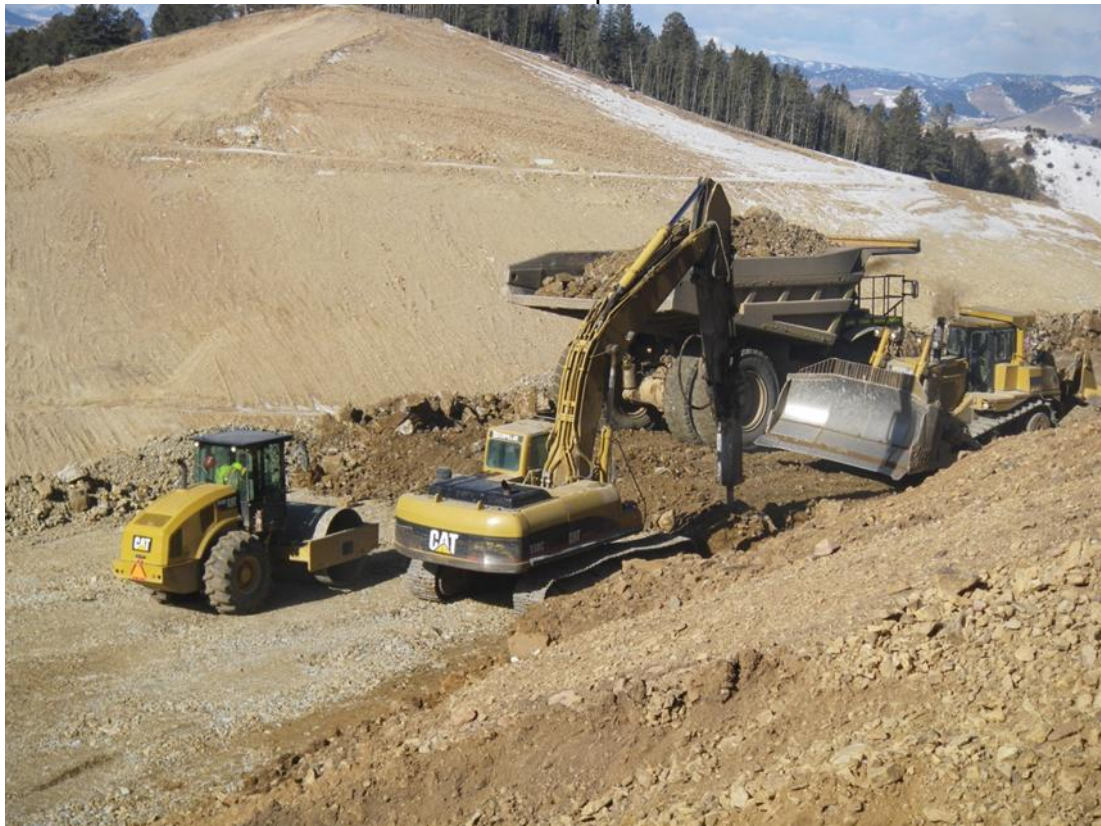
Photo 4: Fill placement at the ADR Haul Road.
