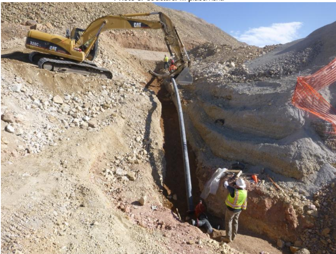
Photo 4: Installing HDPE pipe for water stand pond.
