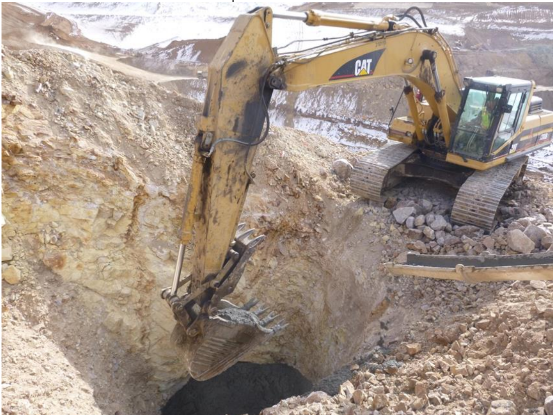
Photo 4: Concrete plug placement at Underground Working # 6302.
