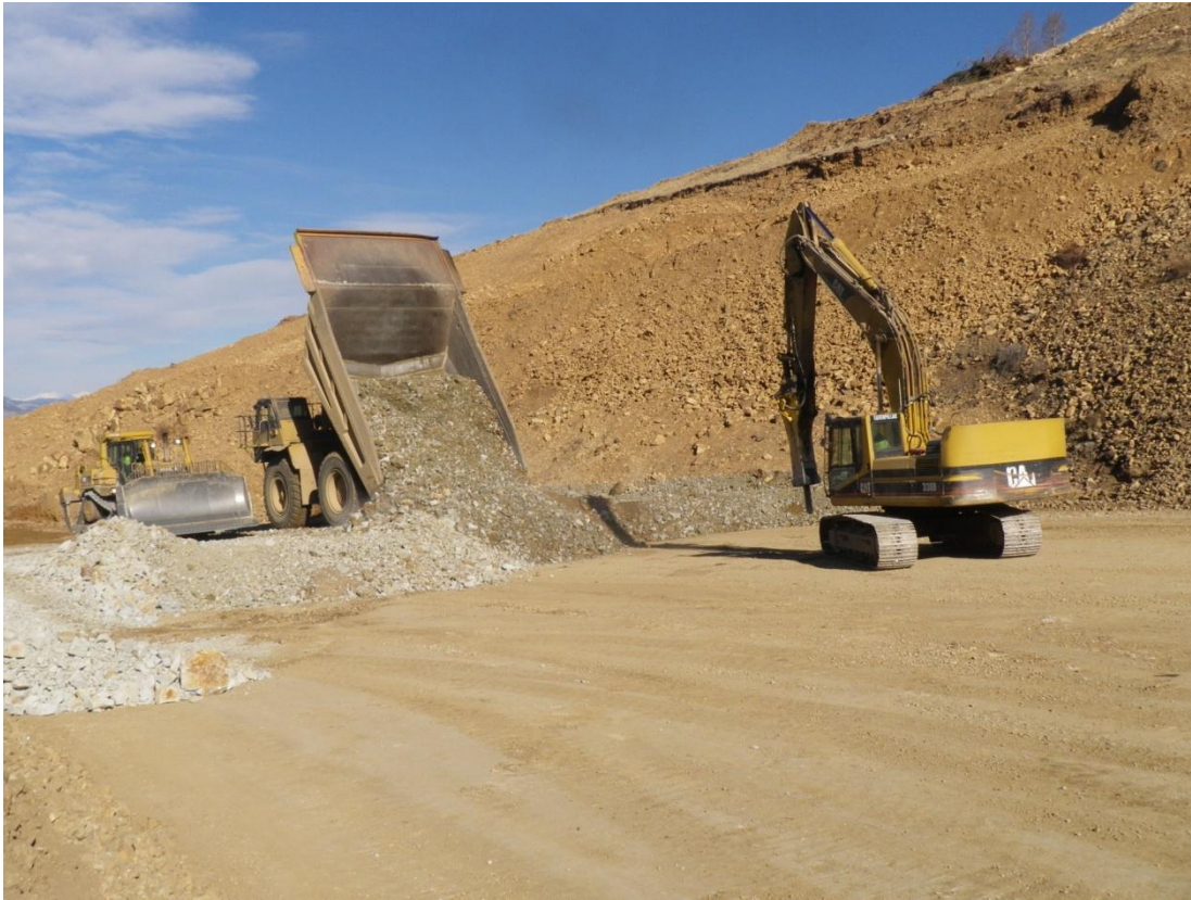
Photo 3: Fill placement at the buttress fill area.
