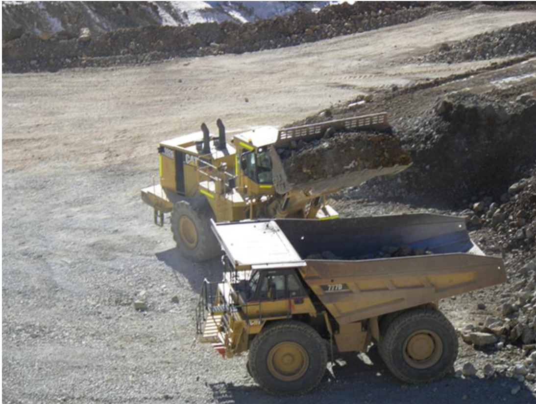
Photo 3: Cut operations near station A14+00.
