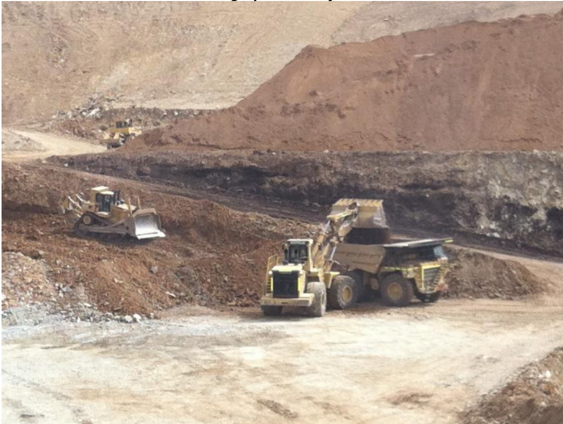
Photo 1: Loading Cat 777 haul trucks with structural fill.
