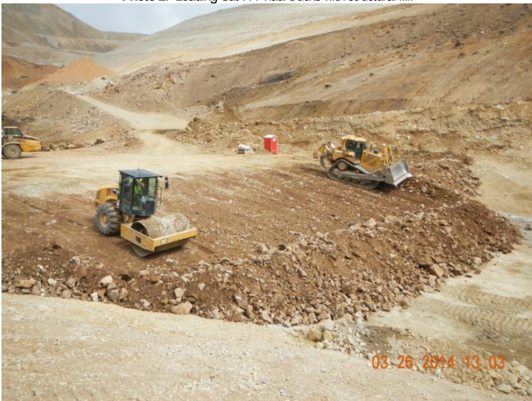
Photo 2: Structural fill placement.
