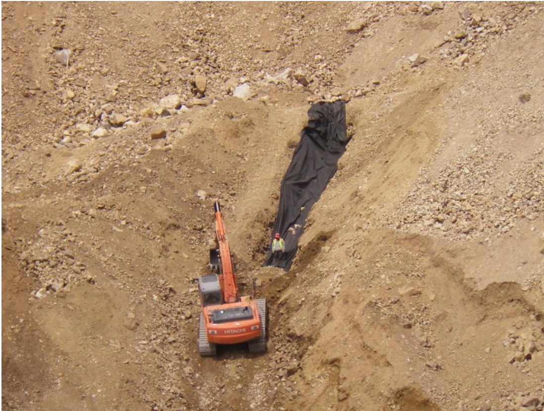
Photo 3: Installing secondary underdrain.
