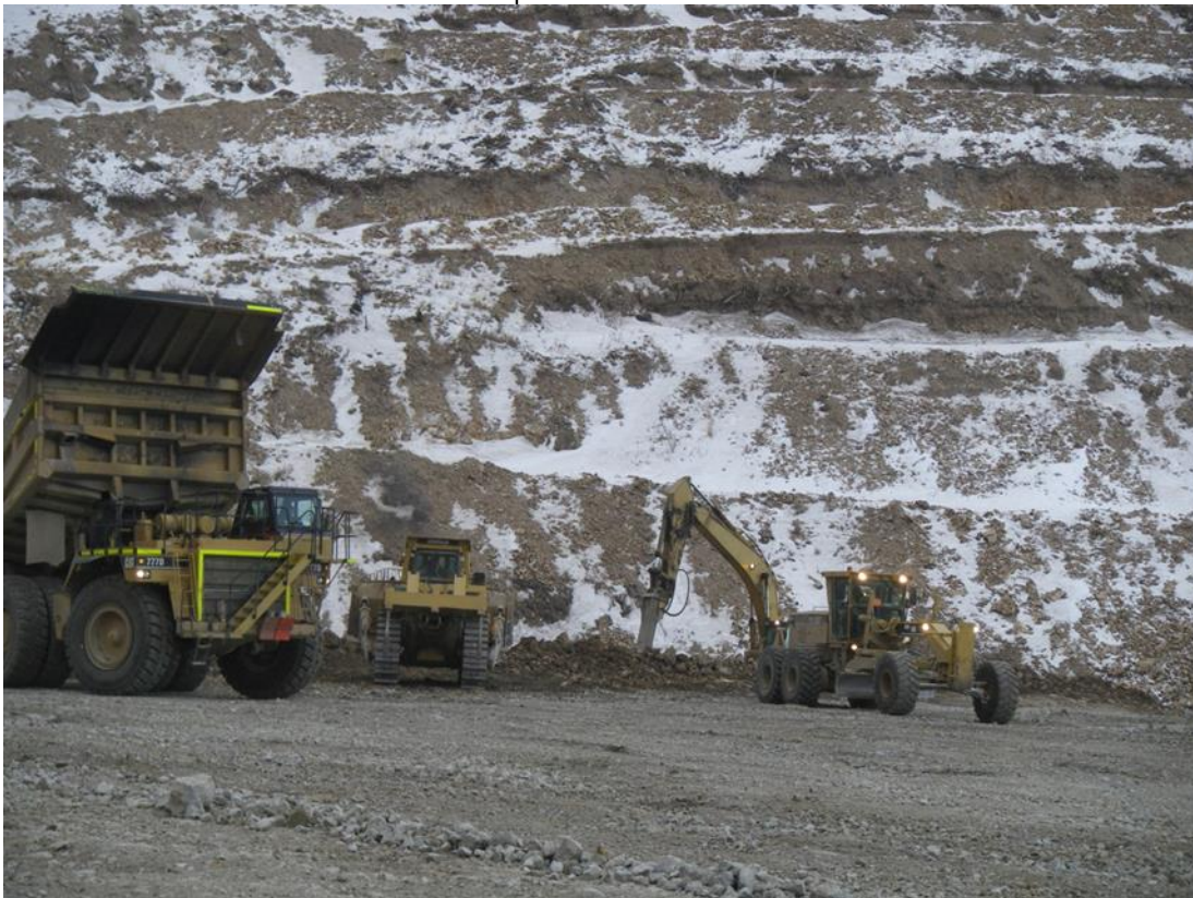
Photo 4: Fill placement at the Butress Fill area.
