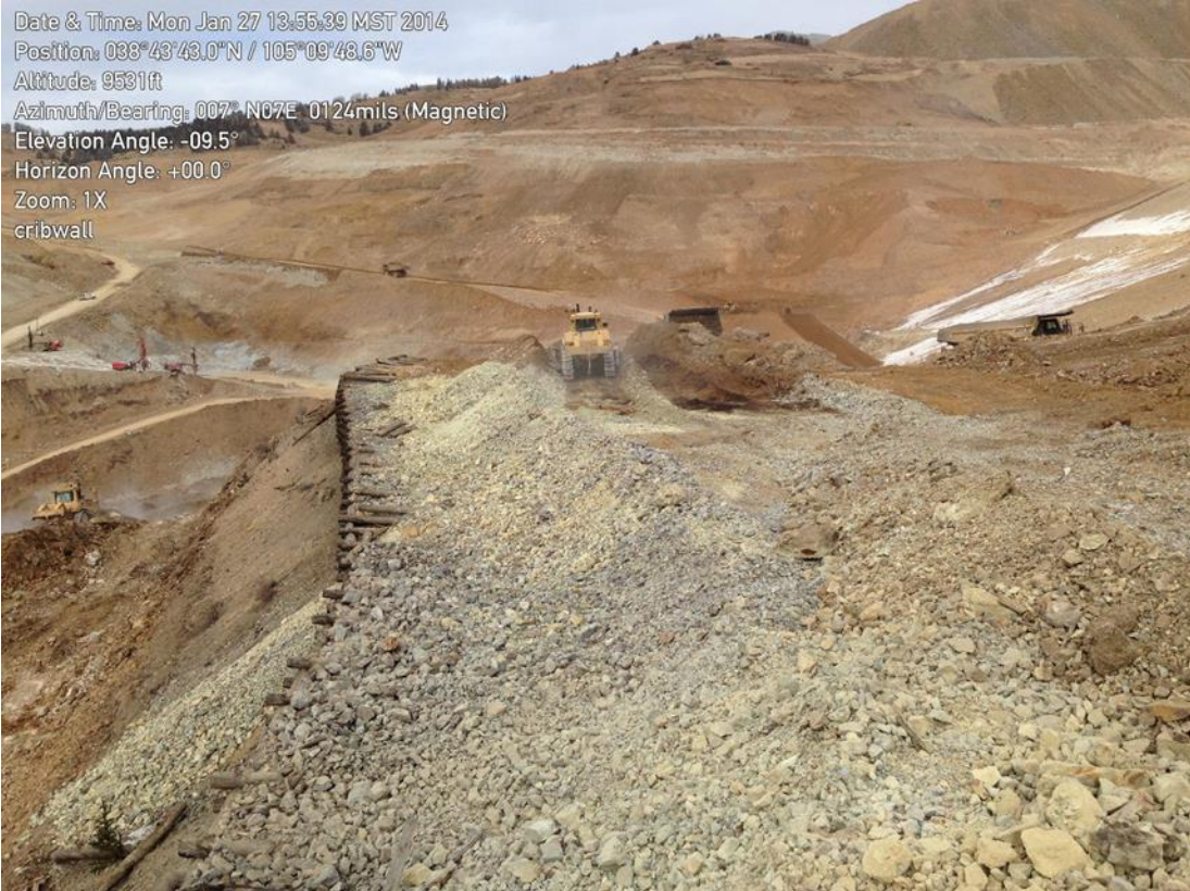
Photo 4: Tailings removal at the Crib Wall.
