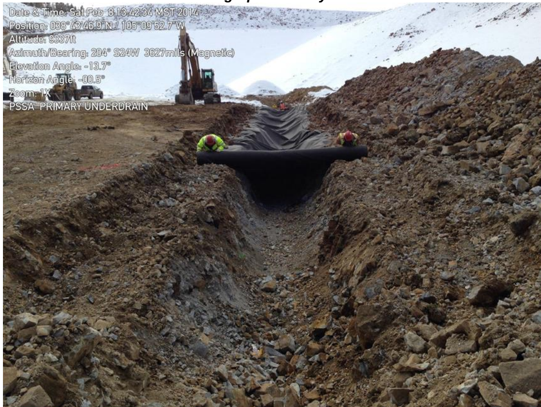
Photo 1: Primary underdrain installation at the bottom of the PSSA.
