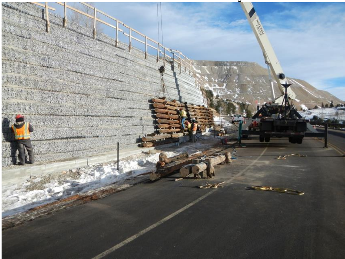
Photo 2: Installed timber panels at the South MSE Wall..
