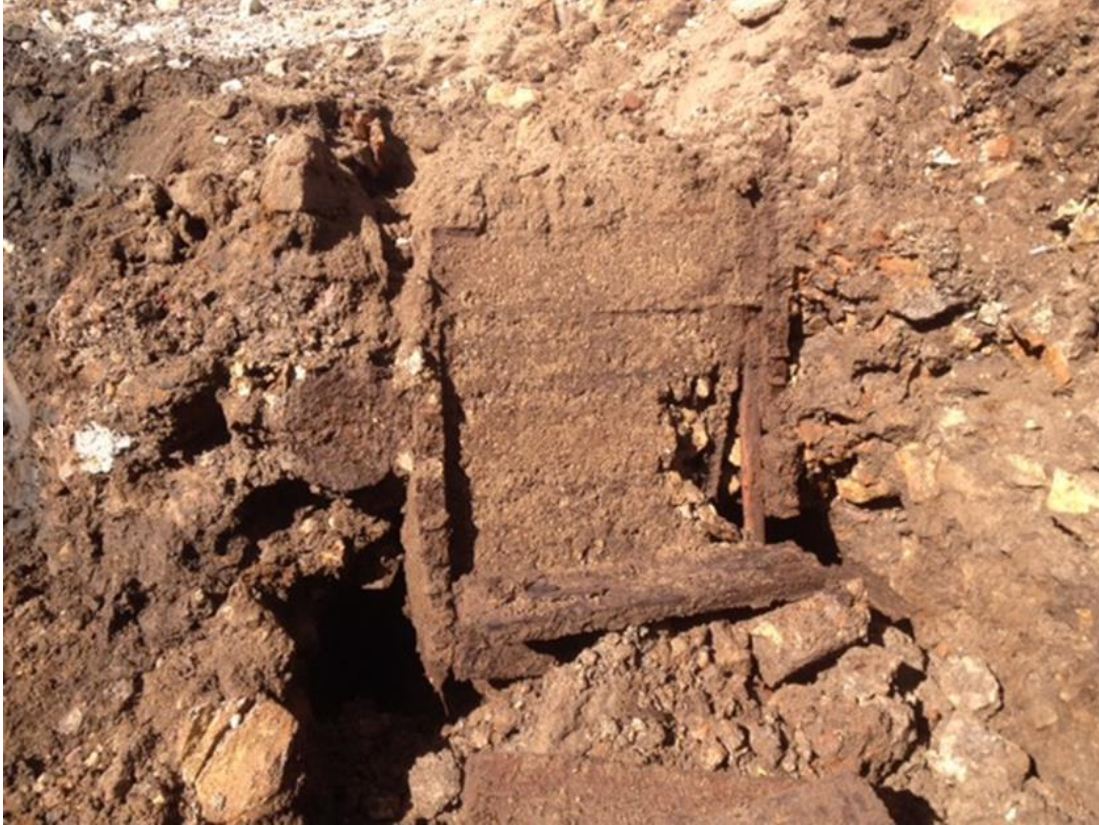
Photo 1: UG # U6334 near the termination of the wood and timbered drainage culvert.
