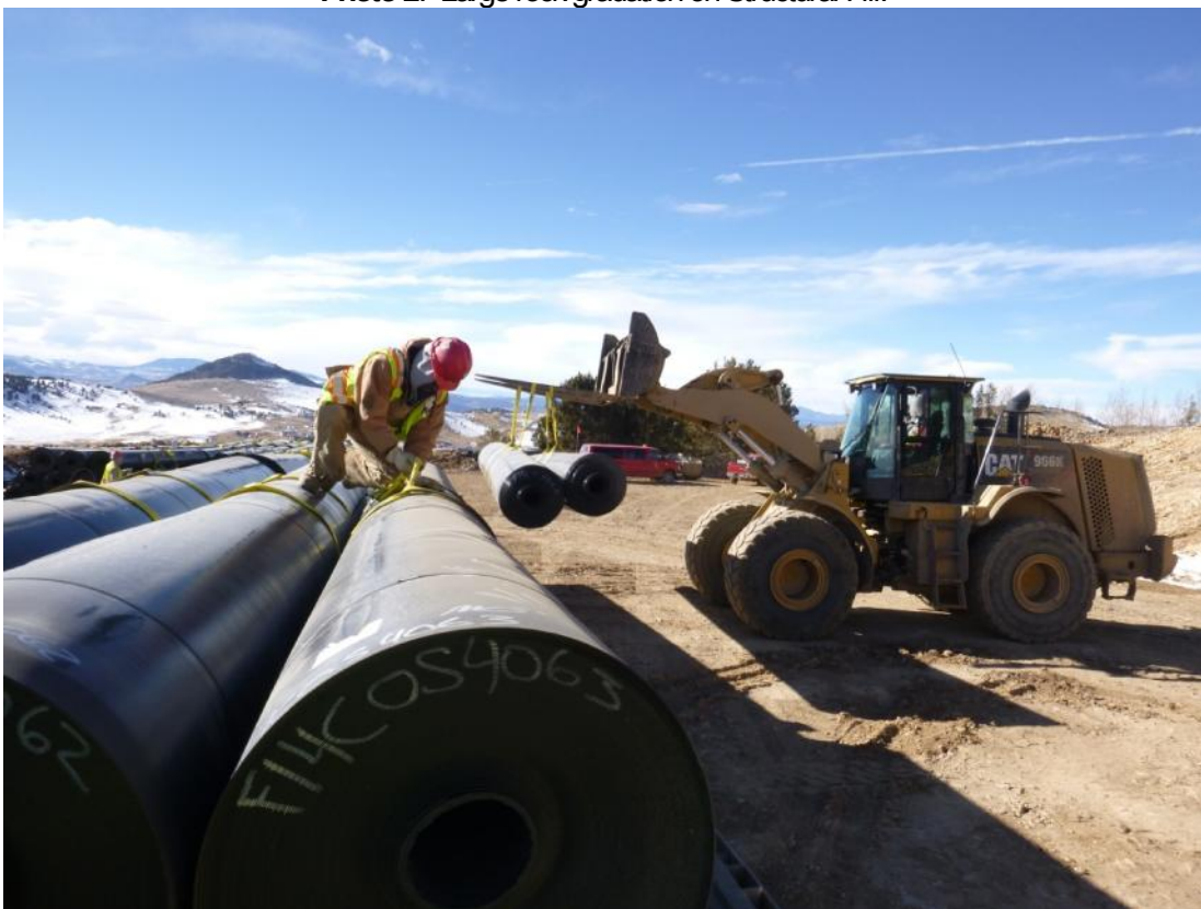
Photo 2: Liner delivery (100-mil smooth LLDPE).
