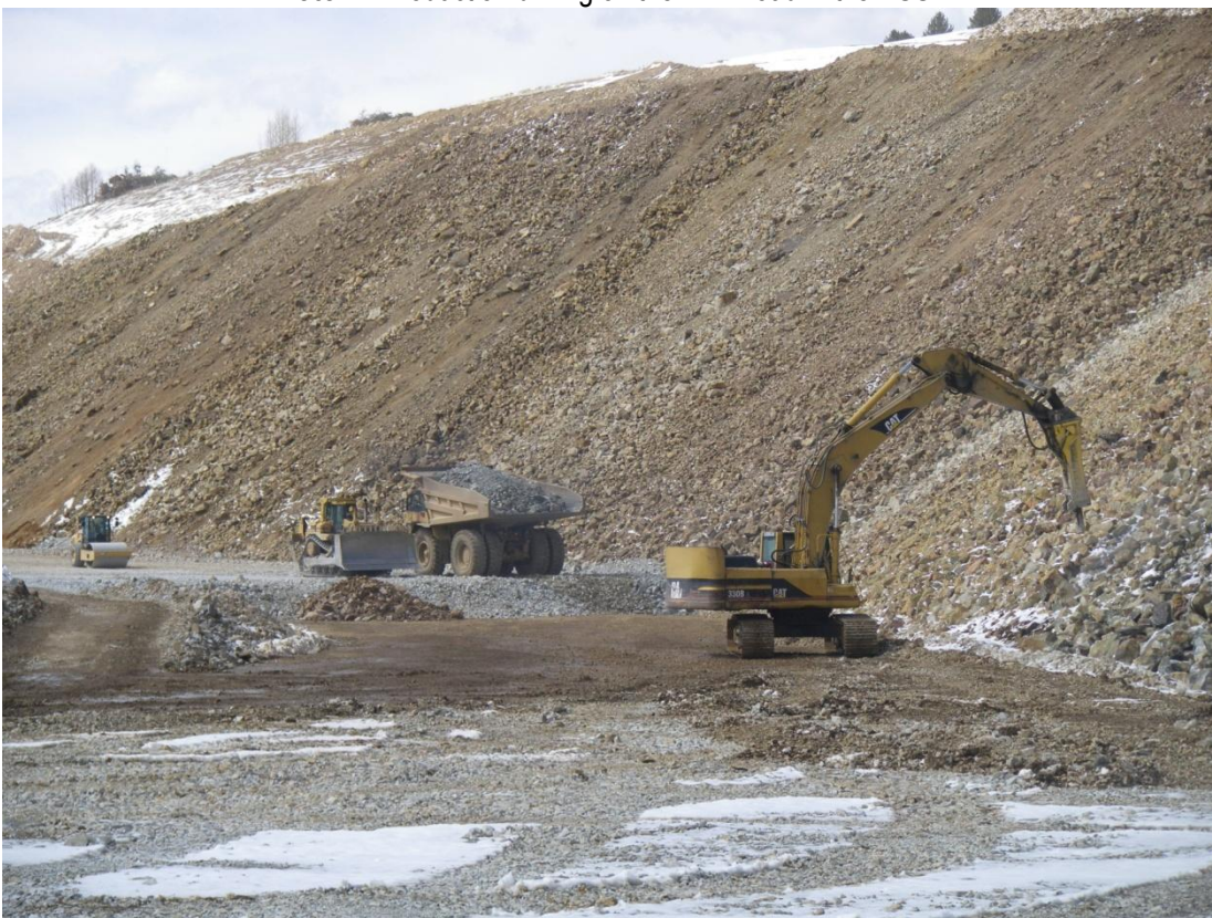
Photo 2: Fill placement at the Buttress fill area.
