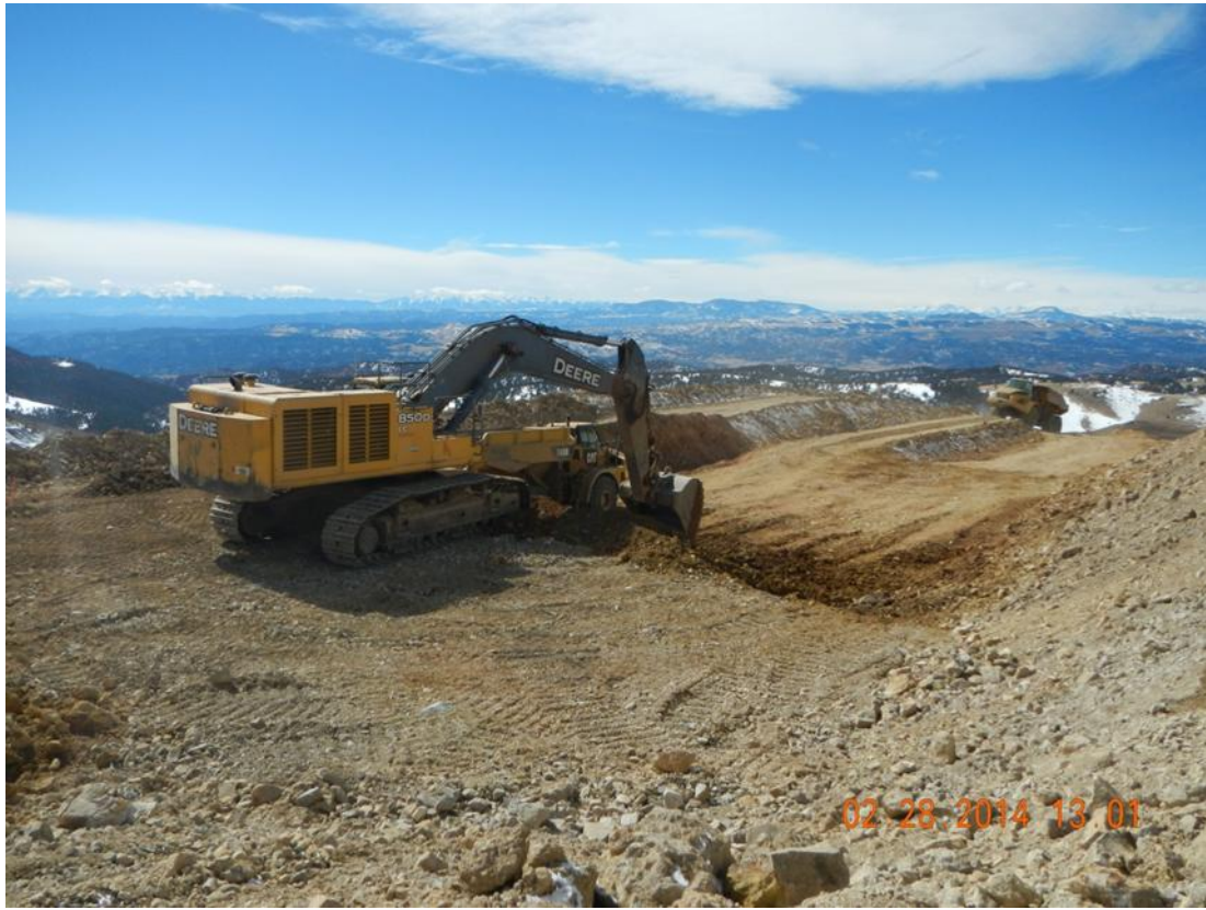
Photo 3: Material removal at Dump 4 for use as structural fill.
