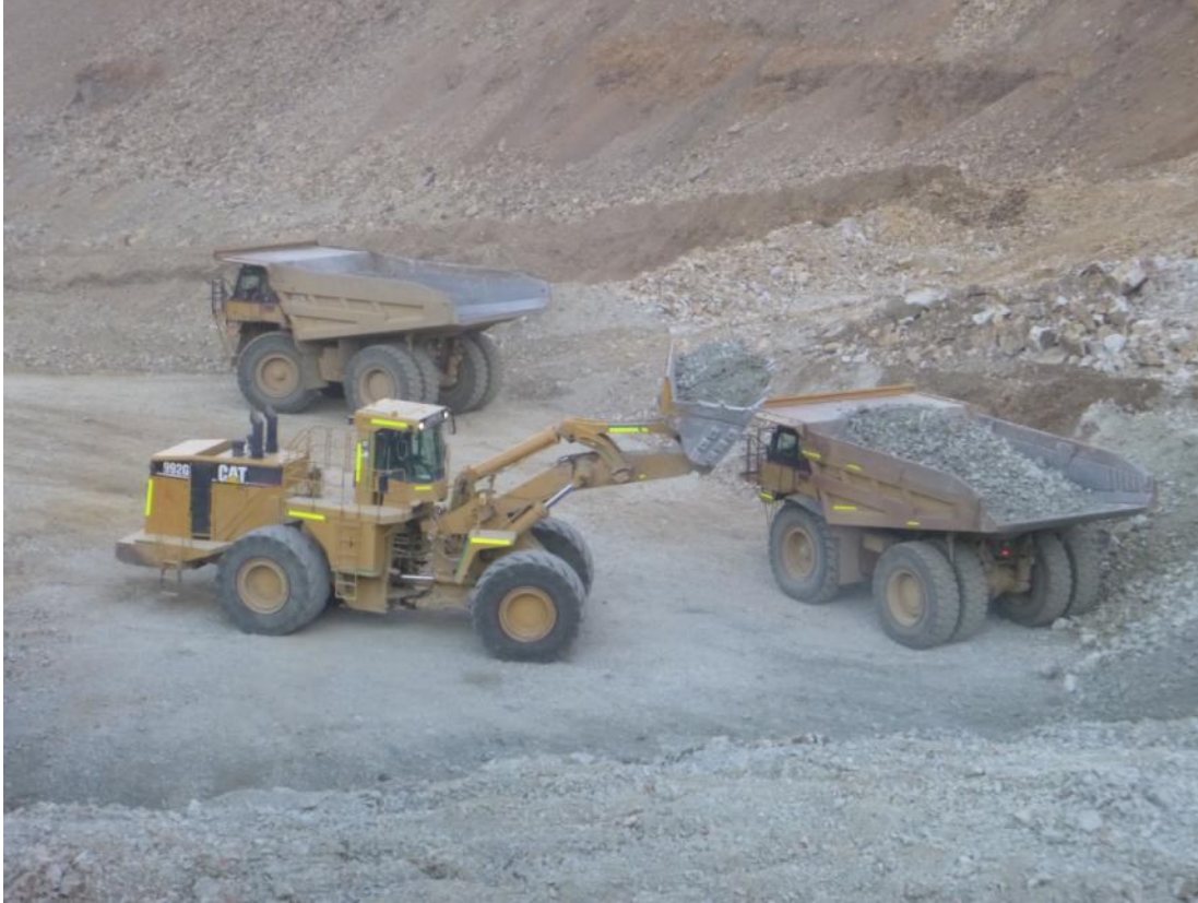
Photo 1: Loading Cat 777 haul trucks with structural fill.
