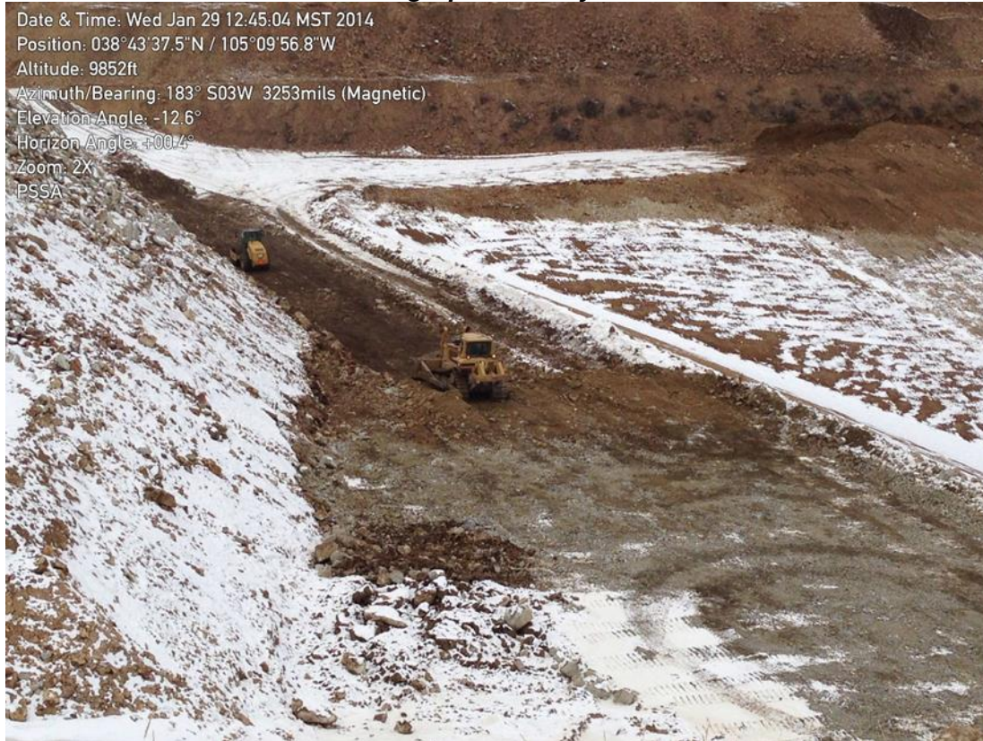
Photo 1: Fill placement at the PSSA toe embankment..
