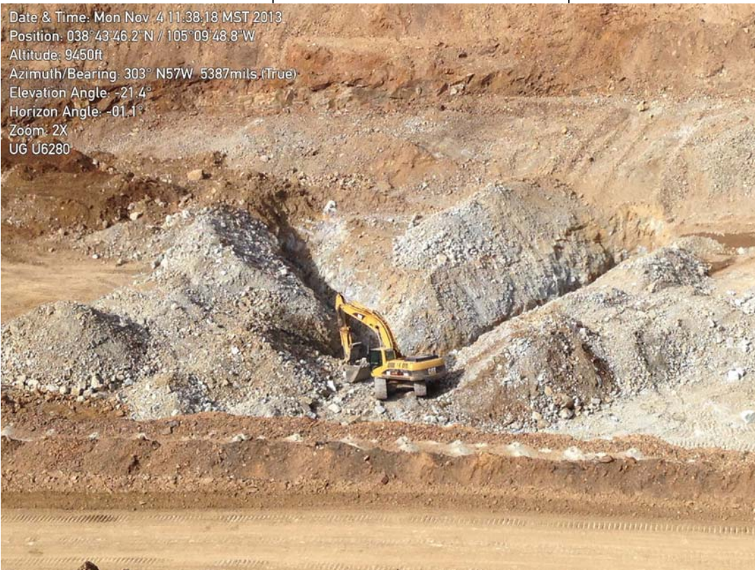
Photo 2: Fill placement at UG U6280.
