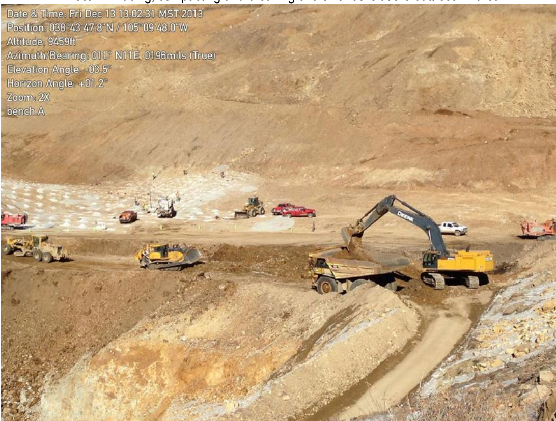
Photo 2: Production drilling near Station A16+00 and cut removal near station A18+00.
