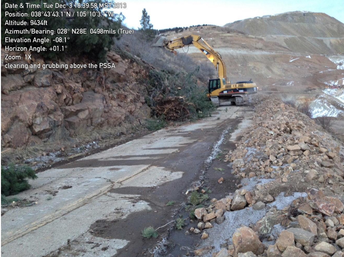
Photo 1: Clearing and grubbing above the PSSA Toe Berm near station A0+00.
