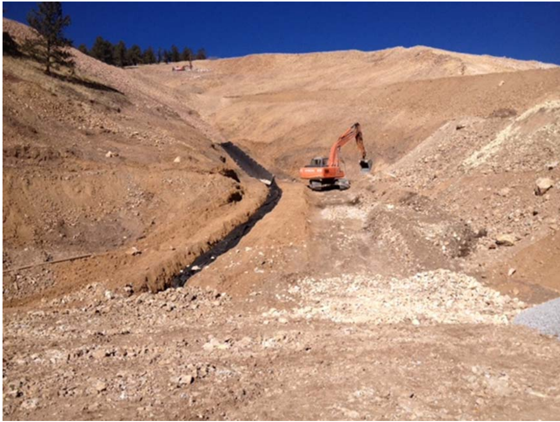
Photo 3: Secondary Underdrain installation near station A6+00.
