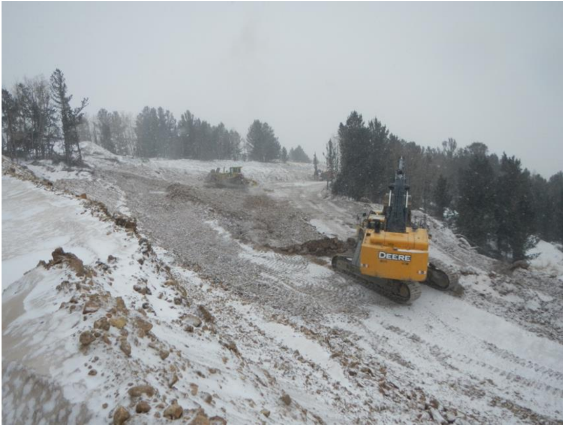
Photo 3: Cut operations in the Phase 2 Diversion Channel area.
