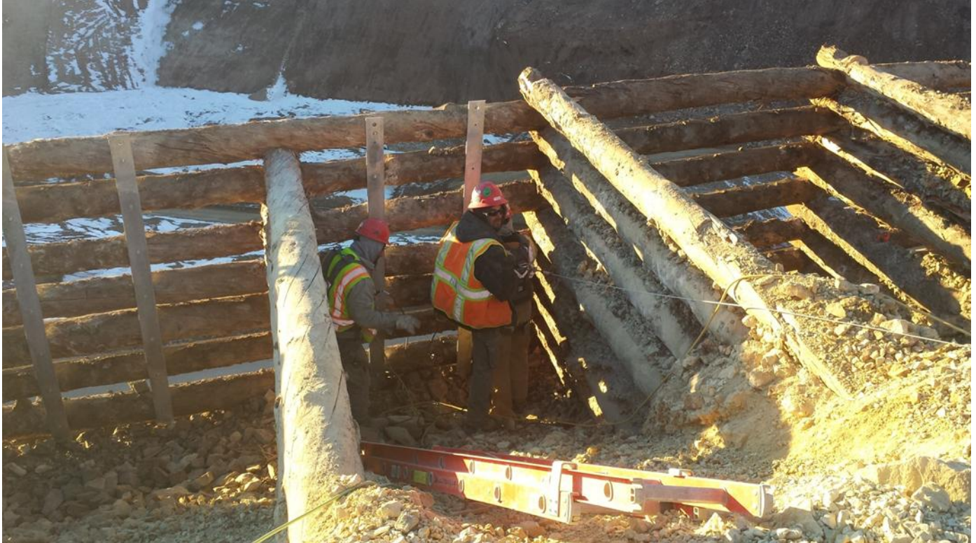
Photo 3: Preparation for timber removal at the Crib Wall
