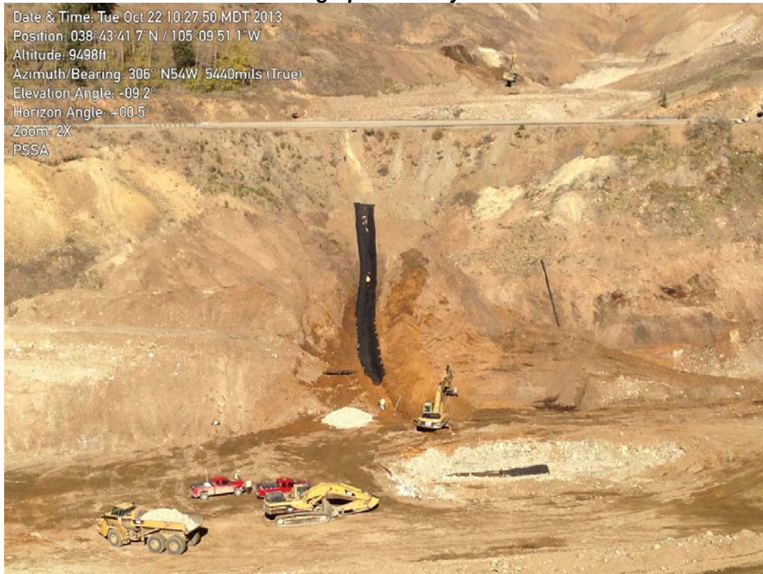
Photo 1 Secondary underdrain construction in the PSSA area.
