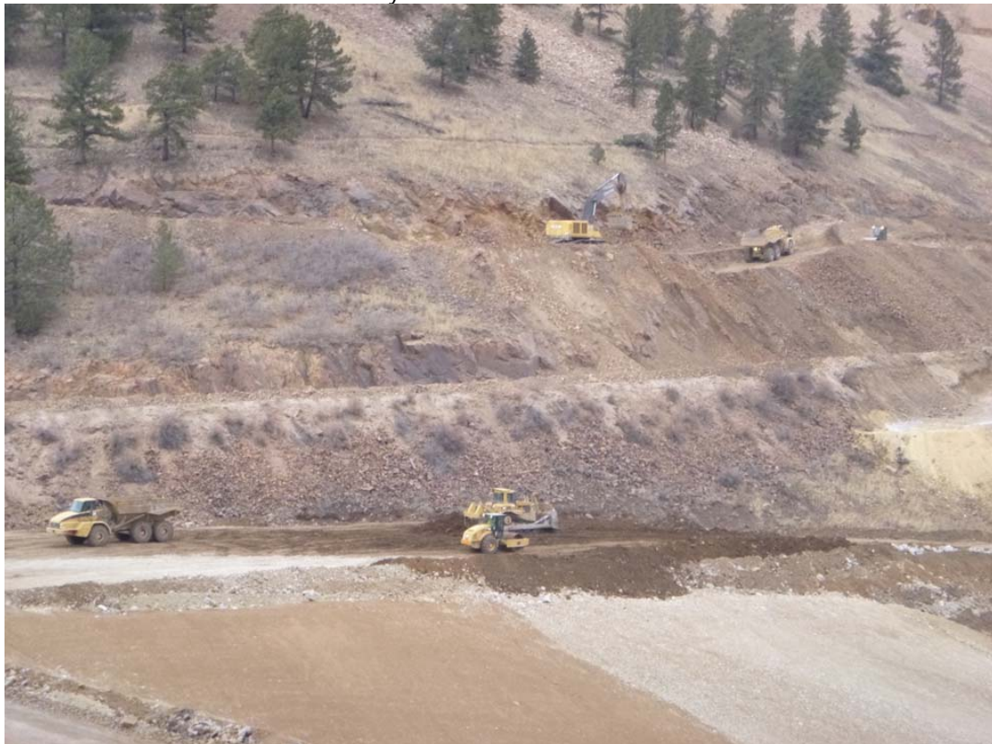
Photo 4: Fill Placement at the PSSA (lower) and cut and fill operations near stations A4+00 to A6+00(upper).
