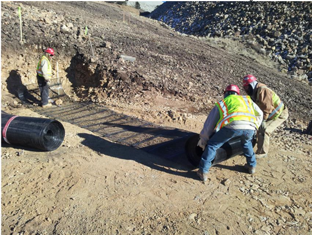
Photo 4: Geogrid installation on UG #6372.
