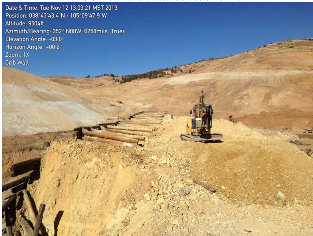
Photo 2: Crib wall removal.
