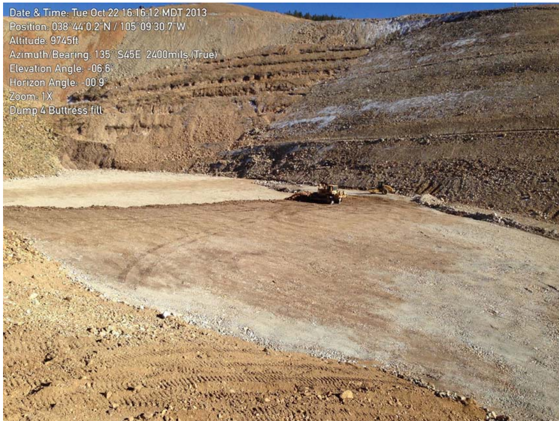
Photo 3: The buttress fill below Dump 4.
