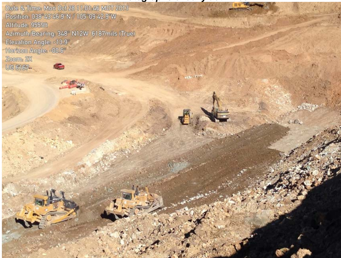
Photo 1 Fill placement at UG 6167 and UG U6273.
