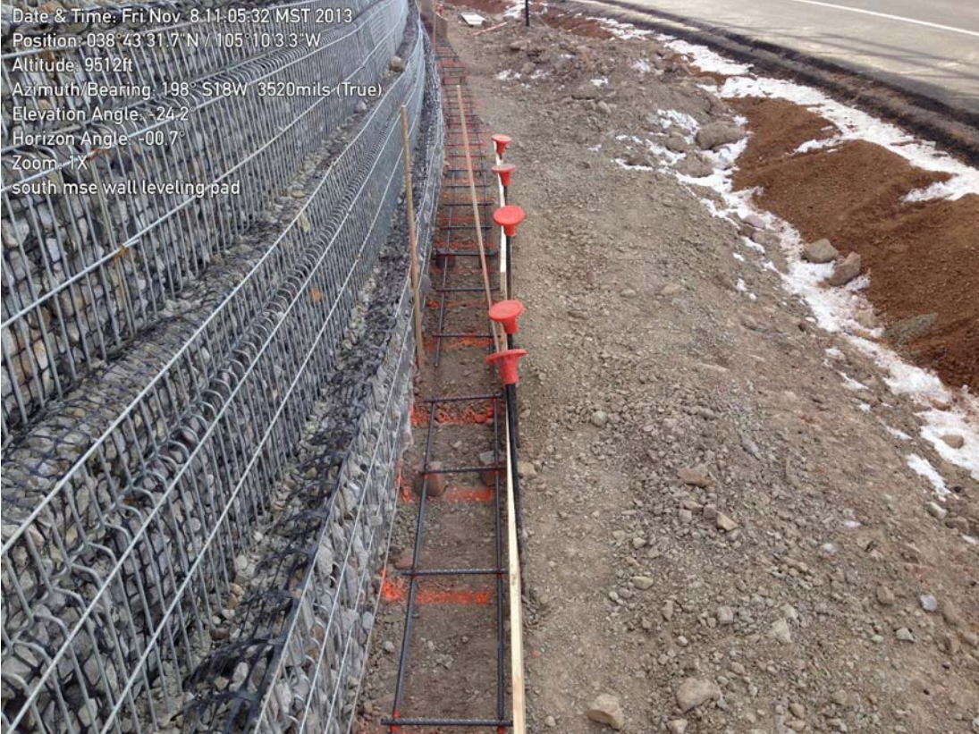
Photo 4: Rebar and concrete formwork for the leveling pad along the base of the South MSE wall.
