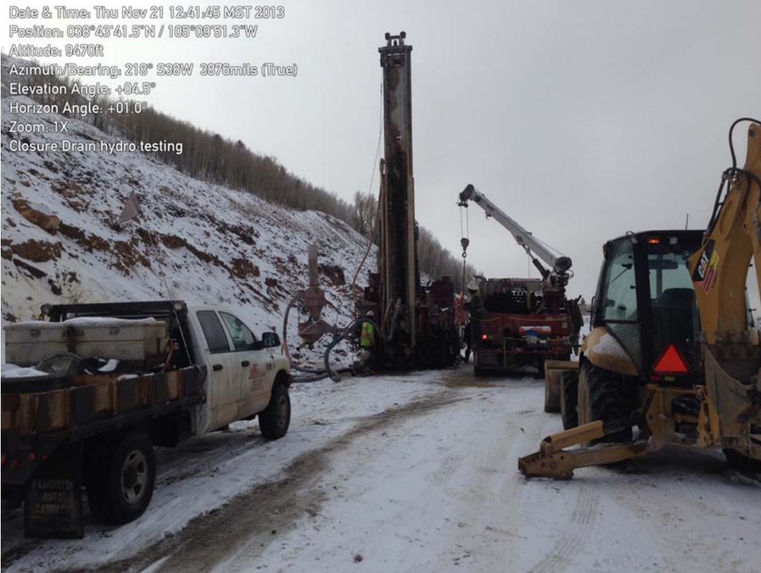
Photo 3: Closure Drain hydro testing borehole abandonment (Borehole #1).
