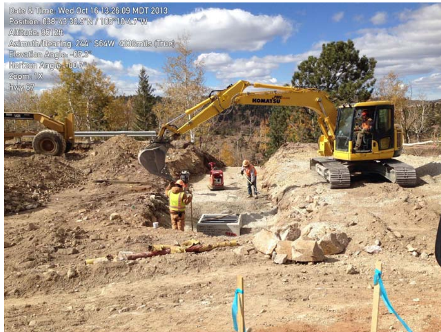
Photo 3: Culvert Installation at the overlook
