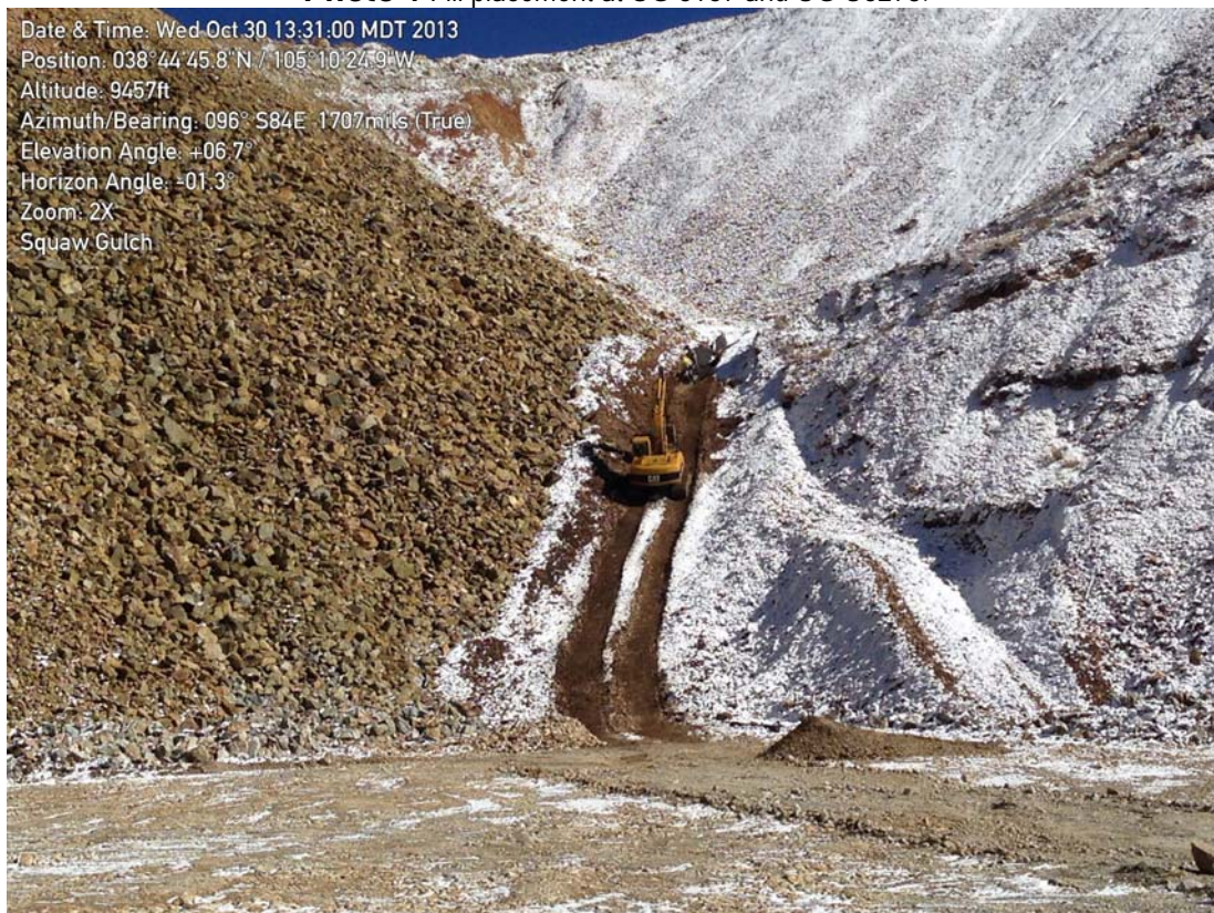
Photo 2: Secondary underdrain construction at Squaw gulch.
