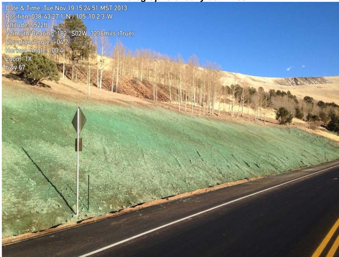
Photo 1: Hydro-seeding southeast of the South MSE Wall.
