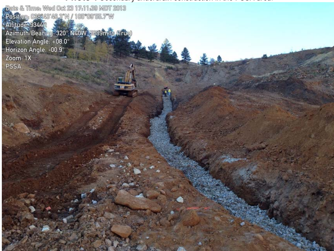
Photo 1 Secondary underdrain construction in the PSSA area.
