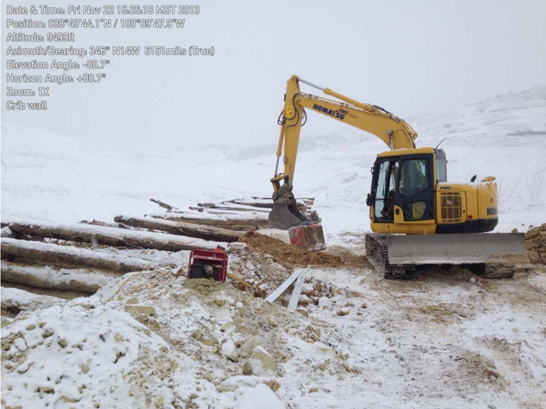
Photo 4: Tailings removal behind the Crib Wall.
