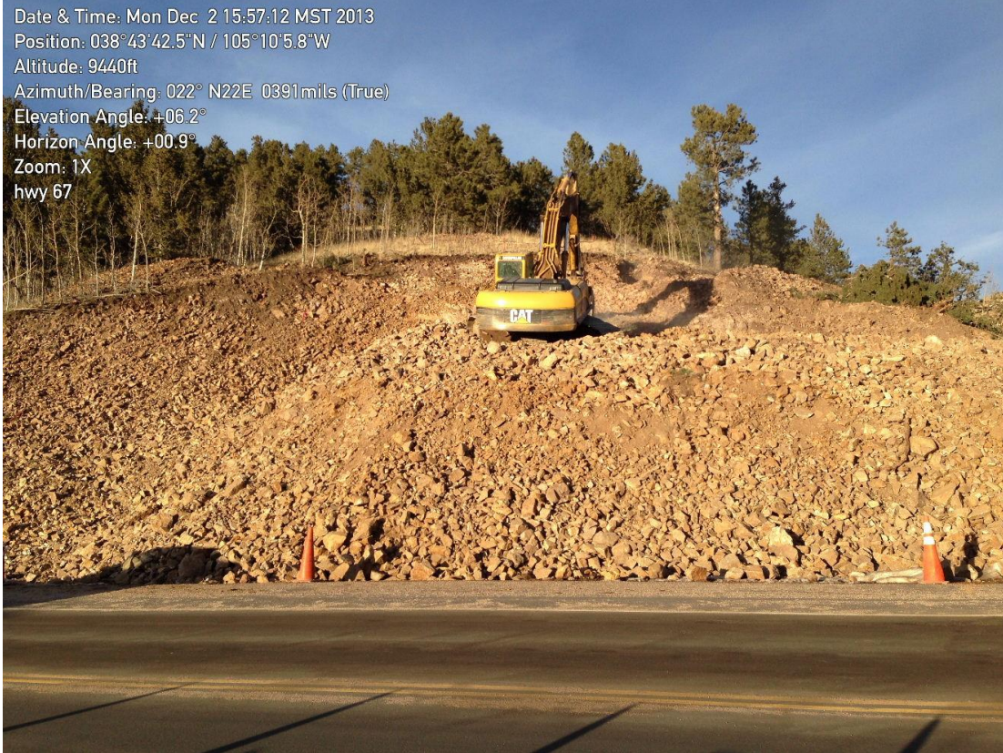
Photo 3: Slope grading near the Cripple Creek tie-in above Hwy 67.
