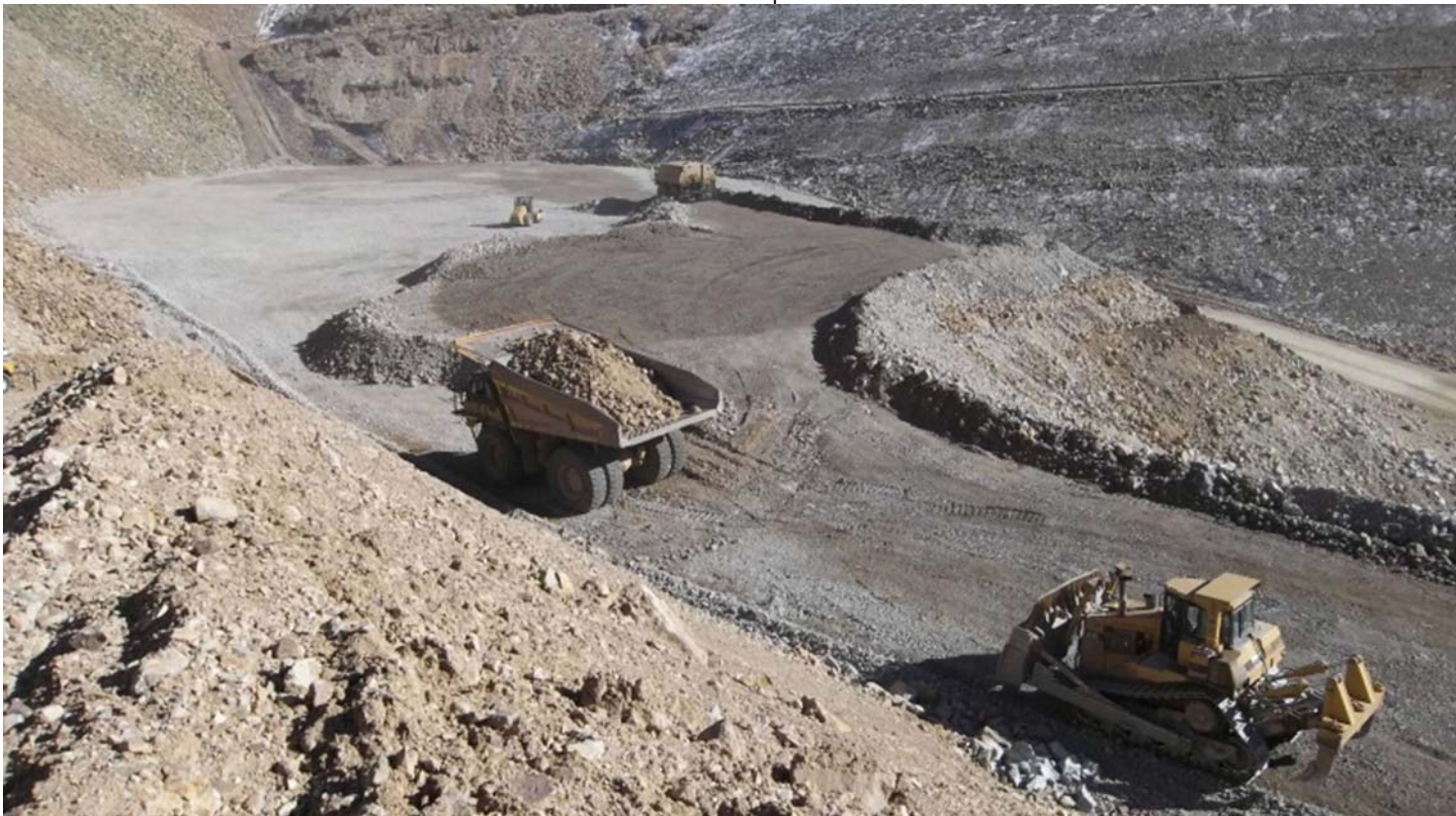
Photo 4: Buttress fill operations below Dump 4.
