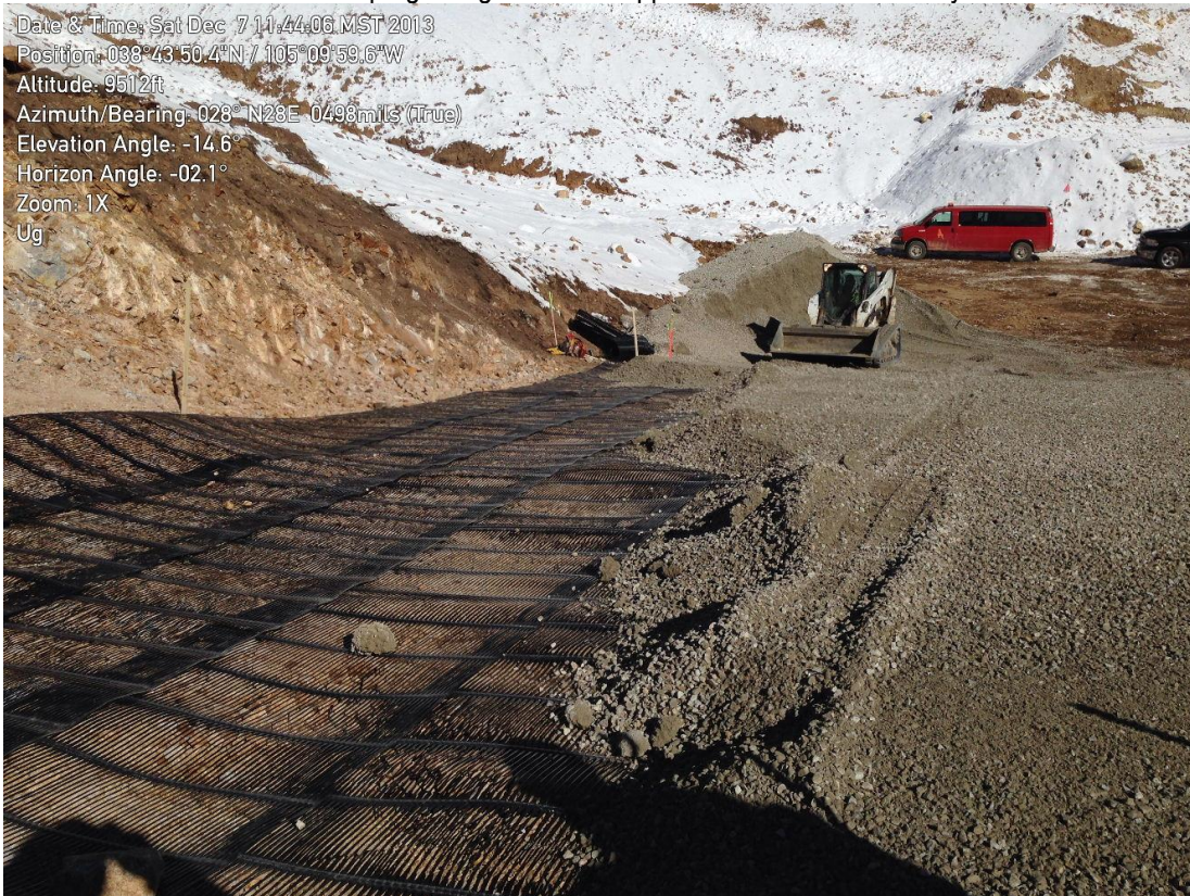
Photo 4: Geogrid placement and fill covering at UG6304.
