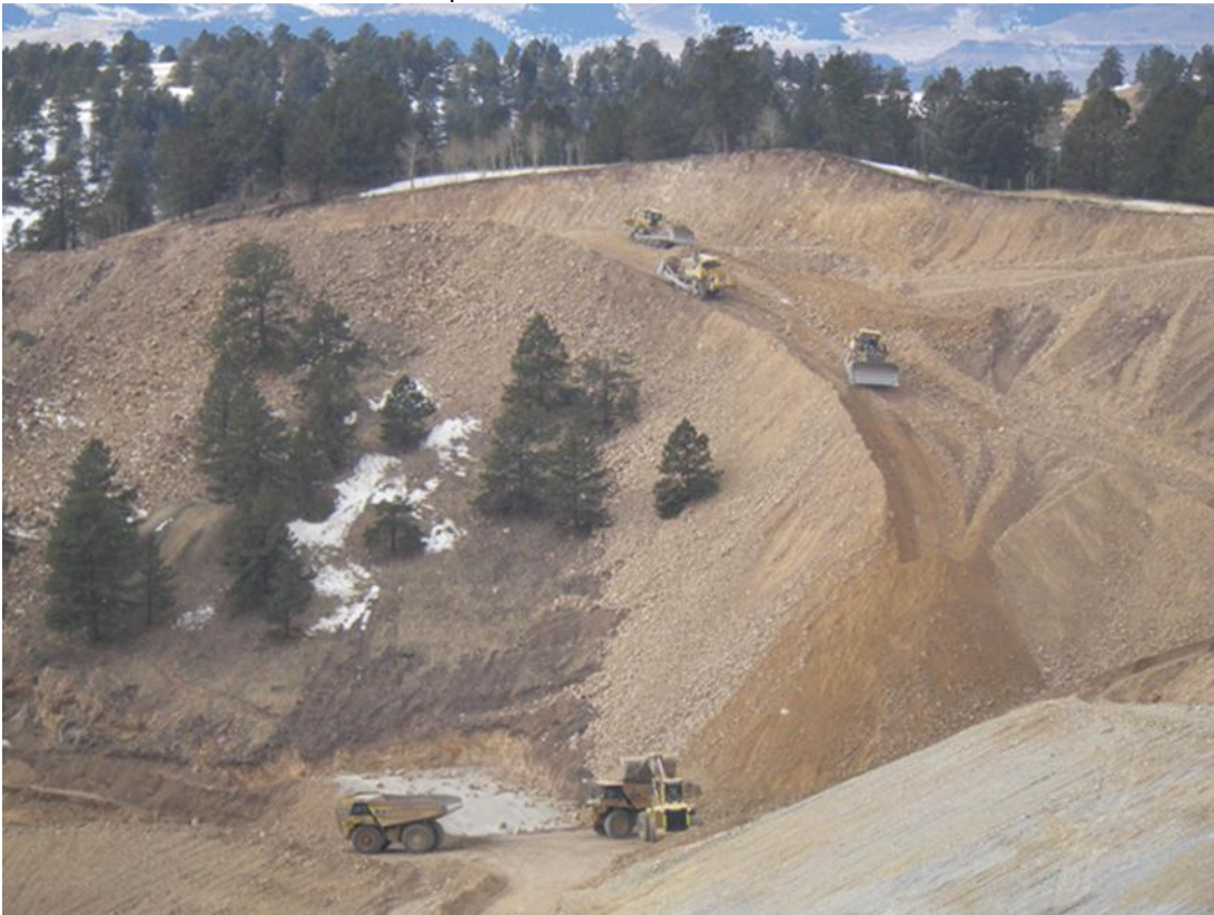
Photo 4: Cut operations between stations Q6+00 and A6+00.
