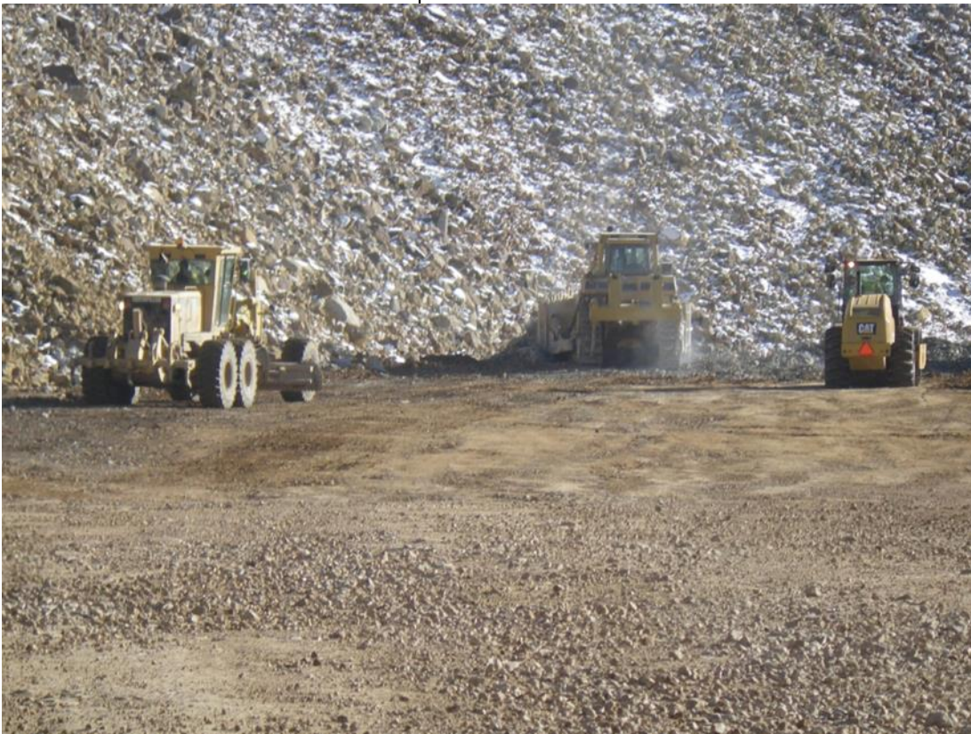
Photo 4: Fill placement at the Butress Fill area.
