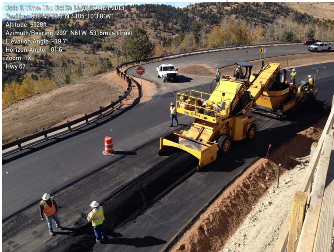
Photo 4: Paving operations adjacent to the South MSE Wall on the Hwy 67 Realignment.
