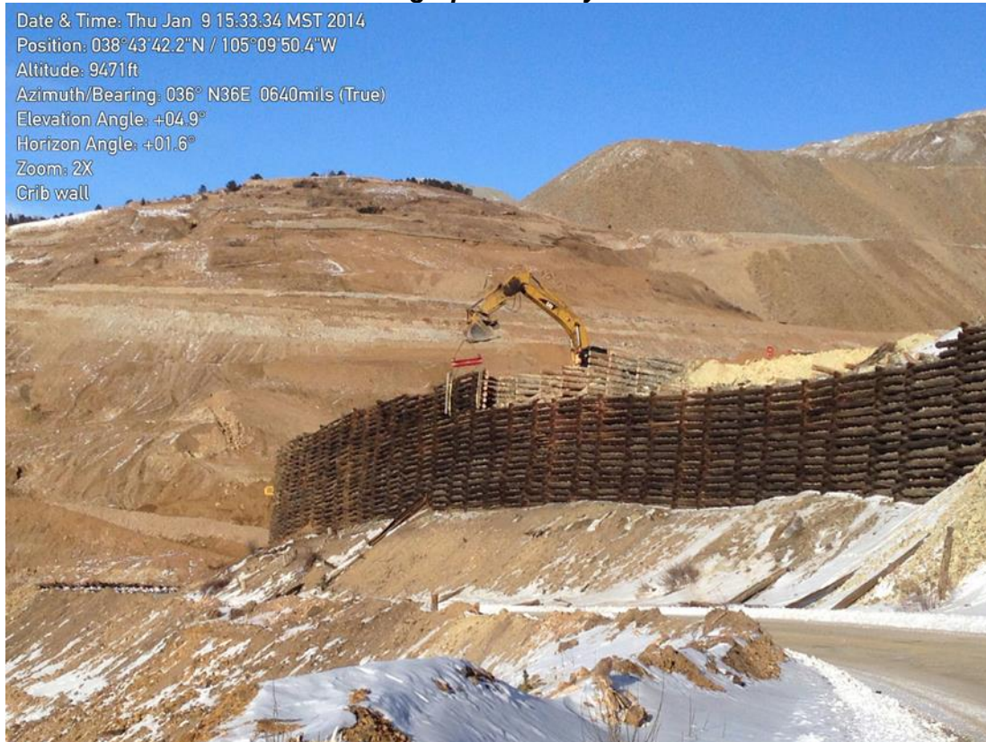
Photo 1: Historical Crib Wall dismantling.
