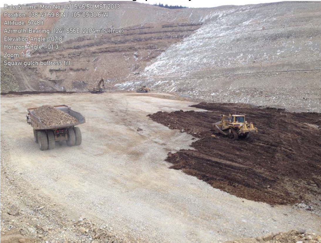
Photo 1 Fill placement at the Buttress fill below Dump 4.
