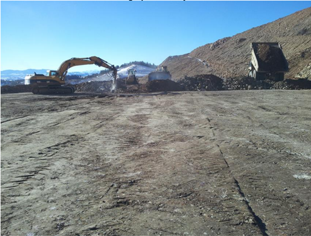
Photo 1: Placing, compacting and breaking oversize rocks at the buttress fill area.
