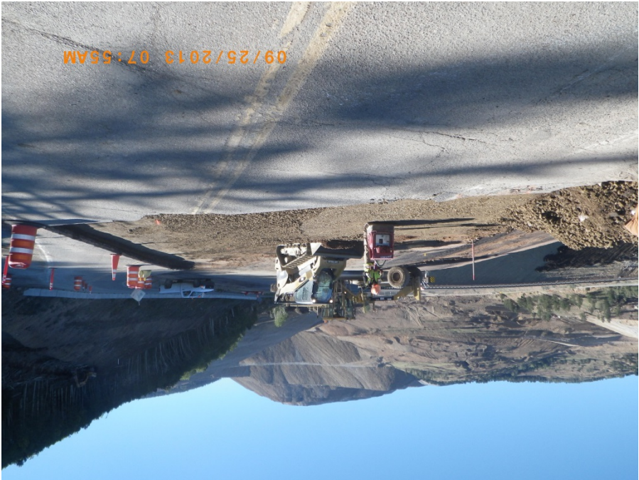
Photo 2: South end of embankment HWY 67 prep for paving
