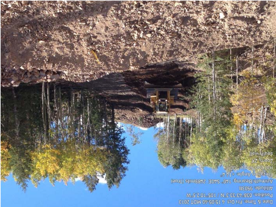
Photo 3: Topsoil placement (Natural Gas Line ROW)
