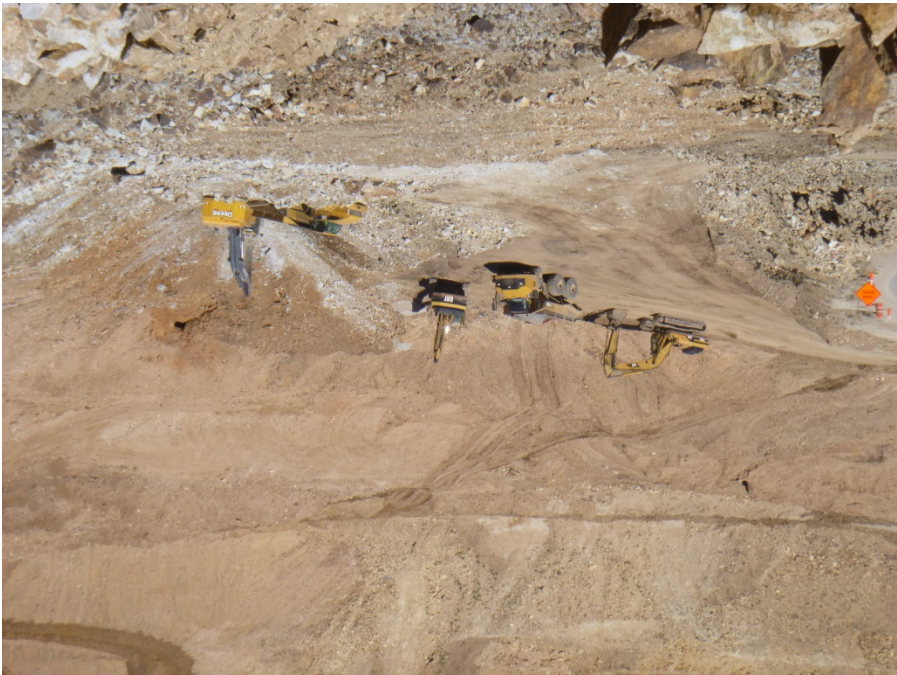
Photo 3: Underground Workings UG#6167 and UG#U6273 – Shot rock removal
