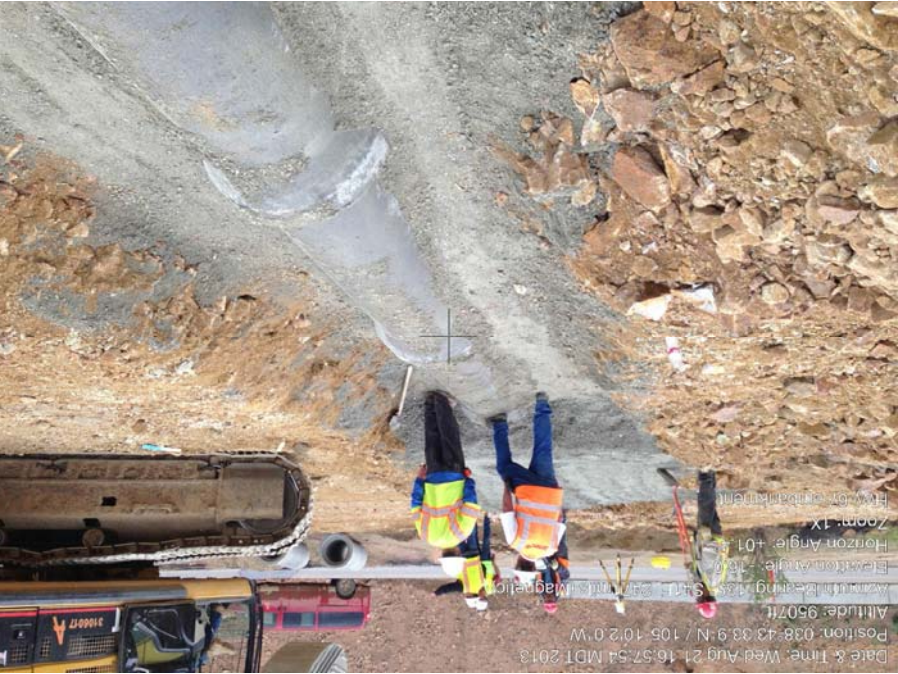
Photo 3: RCP and fill placement, Highway 67 Realignment Embankment
