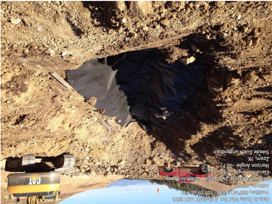
Photo 3: Secondary Underdrain construction
