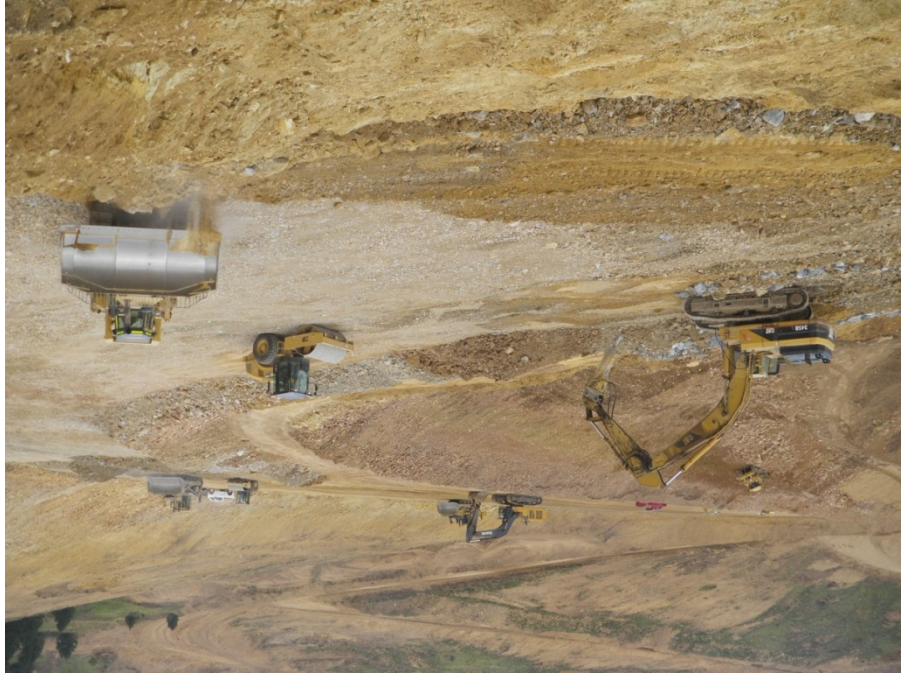
Photo 1: Structural fill placement – Midway ADR Haul Road
