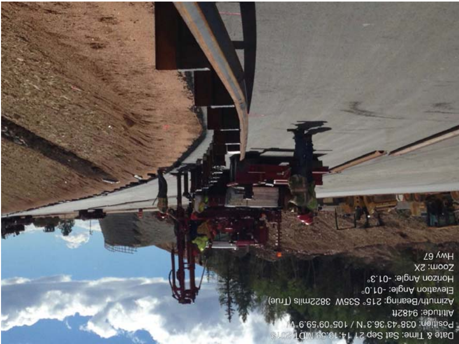
Photo 4: Guardrail Installation – HWY 67
