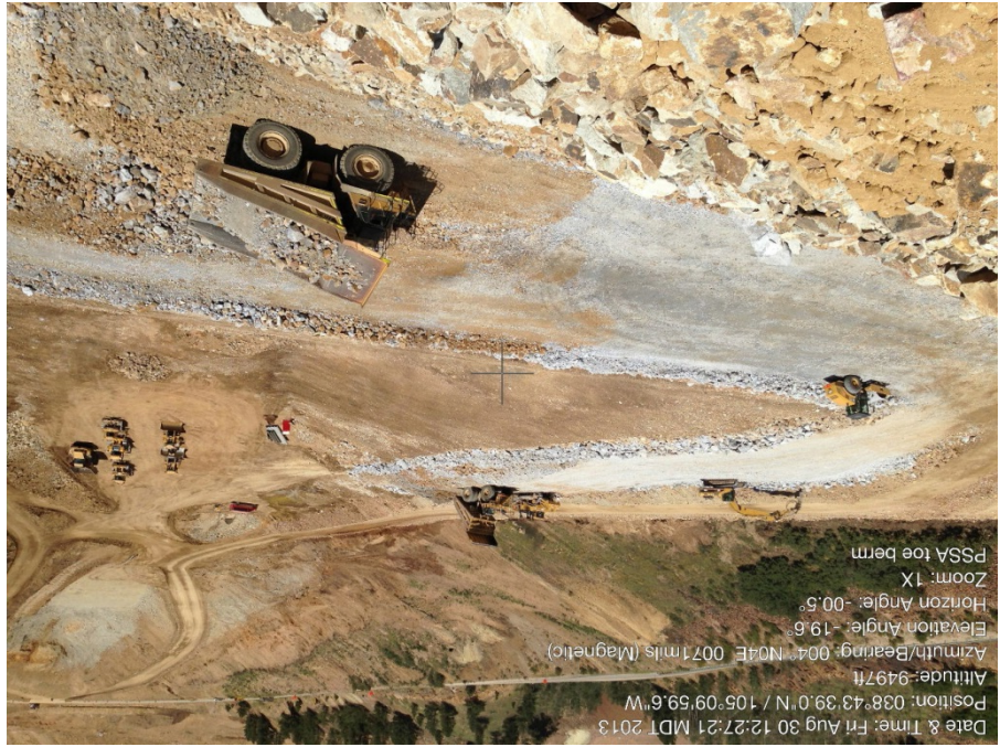
Photo 1: Structural fill placement - PSSA Toe Berm
