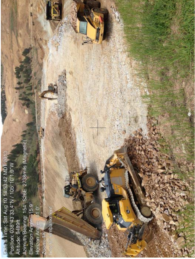
Photo 3: Hwy 67 Embankment Structural Fill Placement
