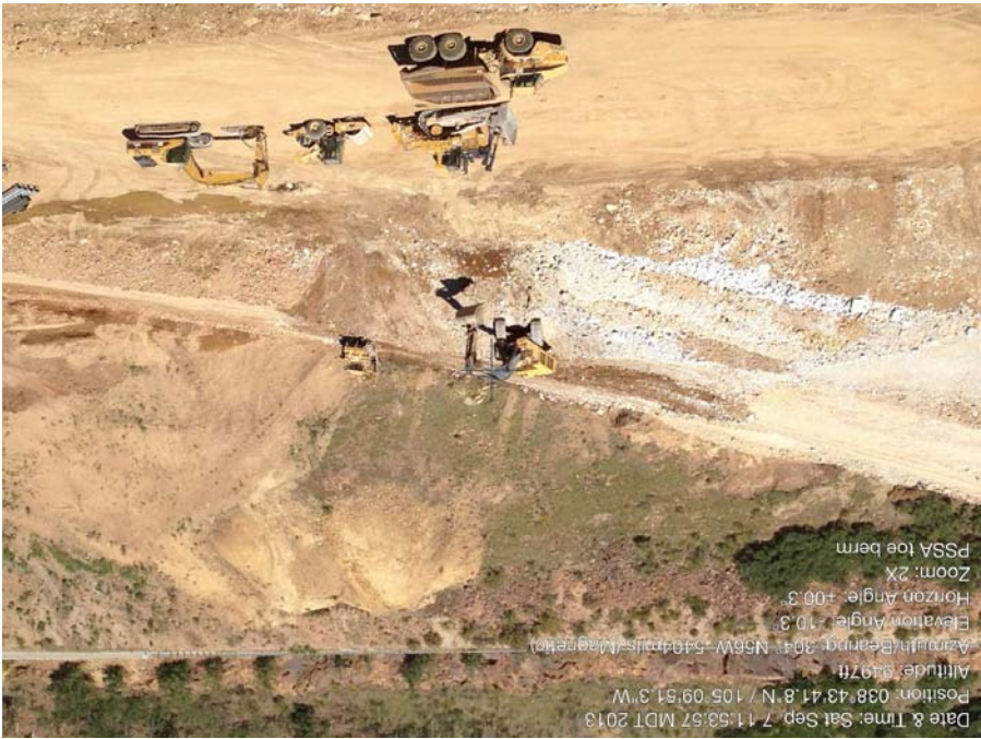
Photo 4: Slope contouring – PSSA Toe Berm
