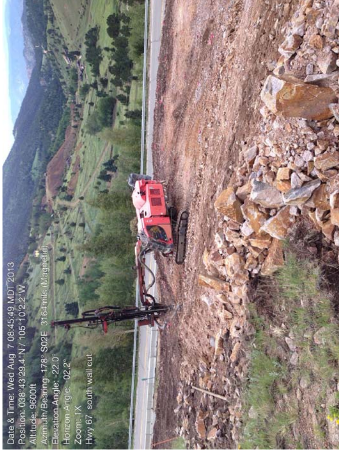
Photo 2: South Crib Wall – Production Drilling
