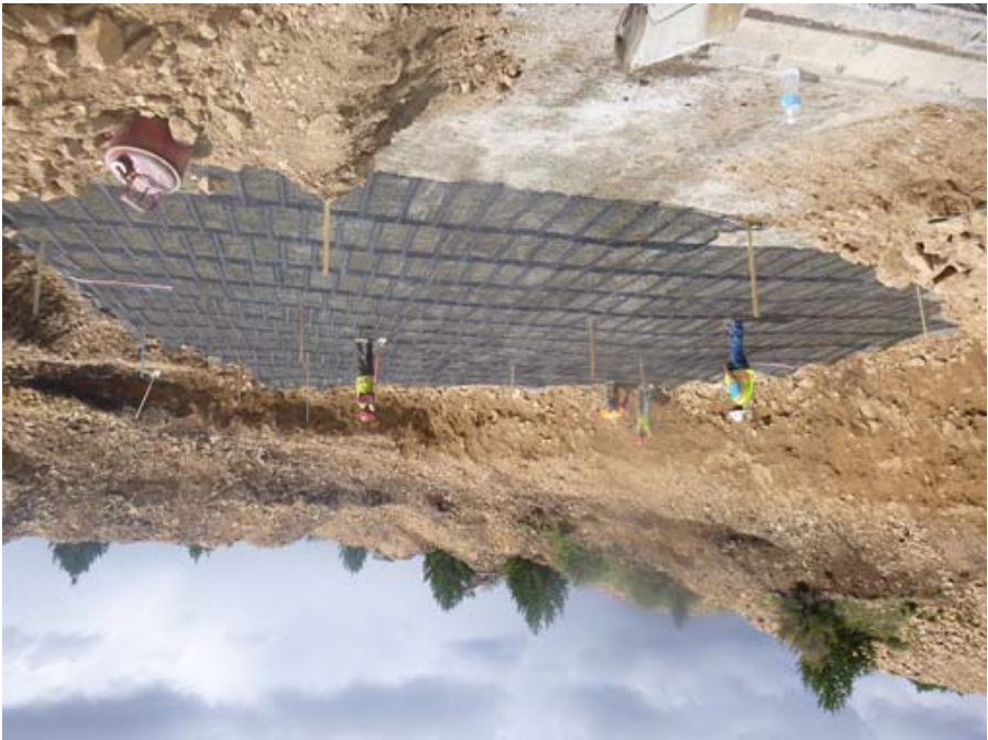
Photo 4: Geogrid placement, Underground Working UG #6239
