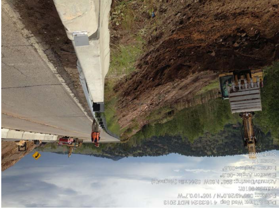
Photo 2: Clearing and Grubbing – HWY 67, Prep for Silver Fill Placement.
