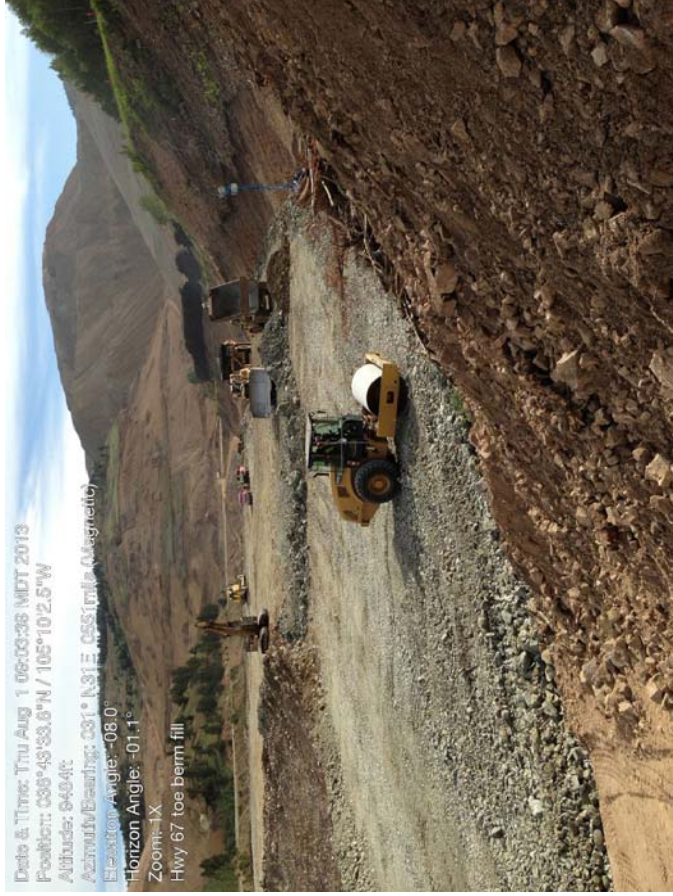
Photo 2: Hwy 67 Embankment compaction and structural fill placement
