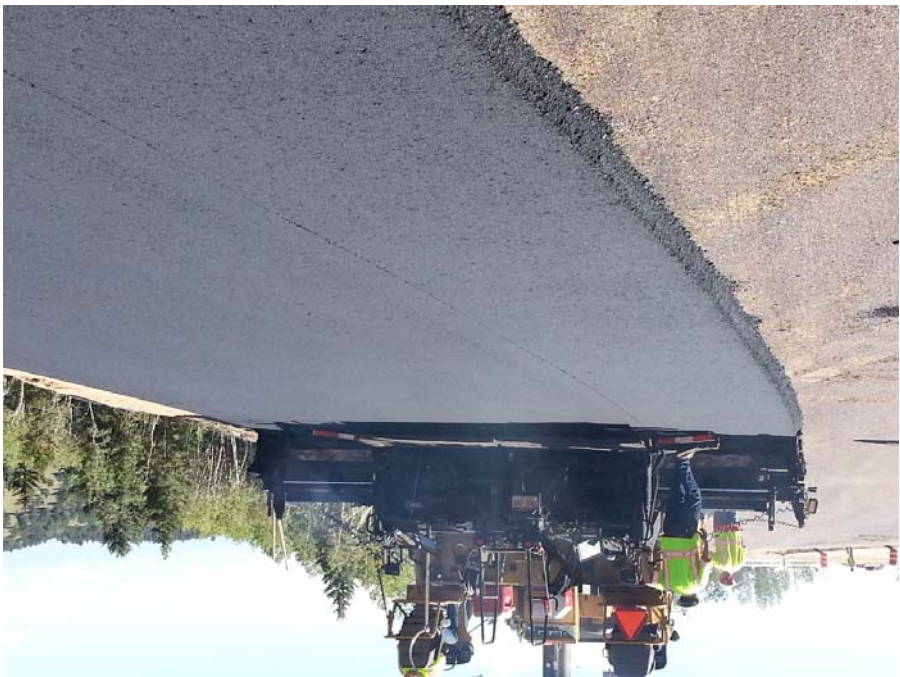
Photo 3: HWY 67 Embankment Paving Bottom 3 inch Mat
