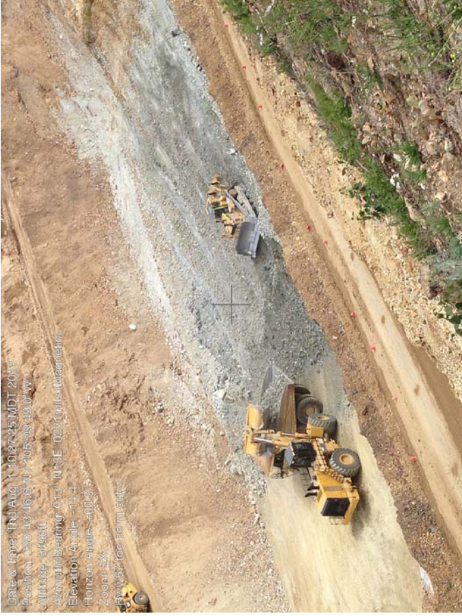
Photo 3: Generated Structural Fill (PSSA Floor)
