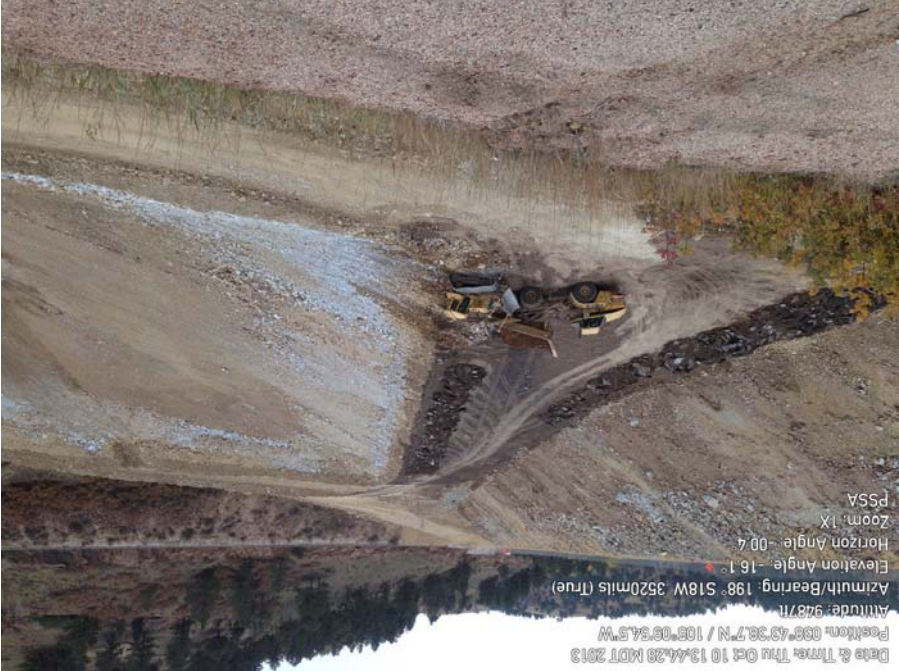
Photo 1: PSSA Toe berm fill placement
