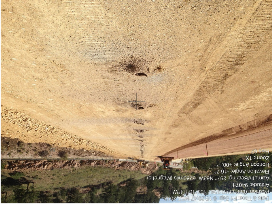
Photo 3: Fence Post Drill Holes – HWY 67 Embankment
