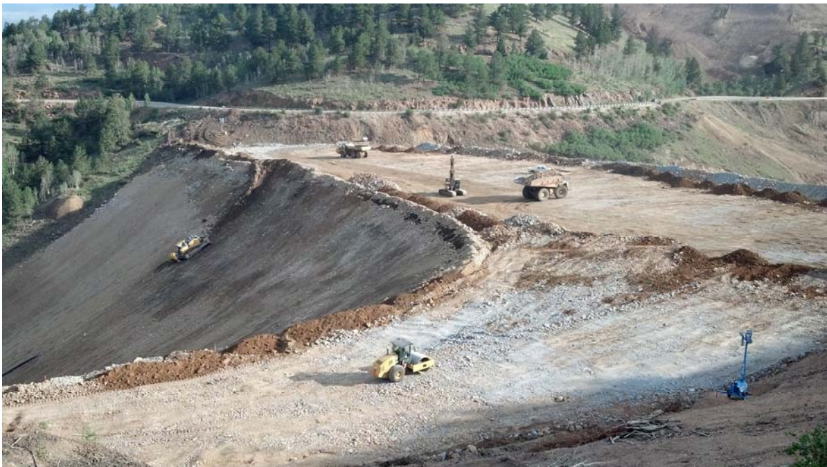
Photo 2: Hwy 67 embankment – Structural fill placement, compaction and slope contouring
