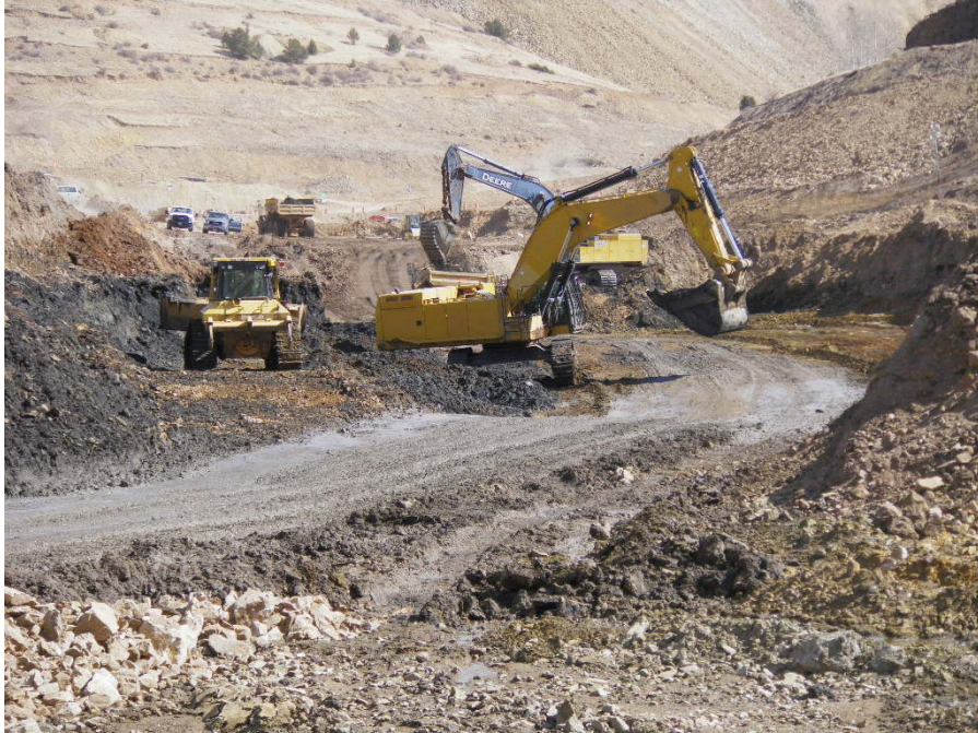
Photo No. 3; Topsoil/unsuitable material removal within the planned HWY 67 embankment footprint
