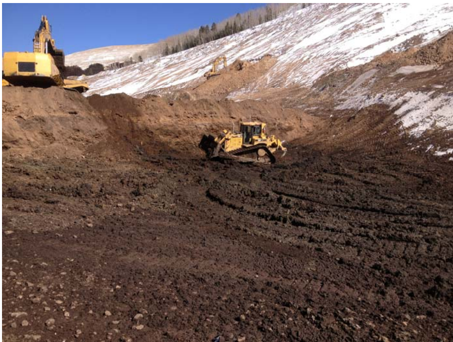
Photo No. 2; Unsuitable material, removal 200 feet east of Proposed Underdrain Pond location
