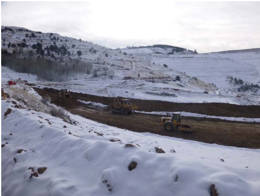
Photo No.2; Structural fill placement and compaction efforts at approximate Sta. 37+00 thru 42+00
