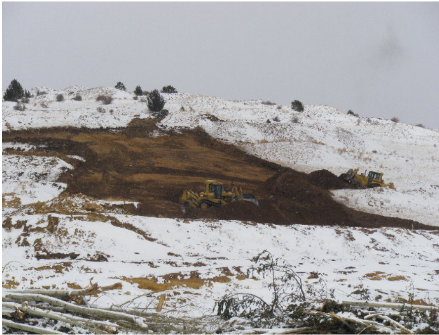
Photo No.3; Topsoil stripping
