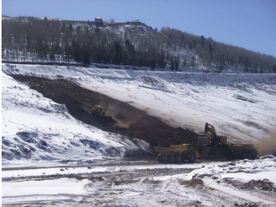
Photo No.3; Topsoil Stripping and Loading, West of HWY crossing
