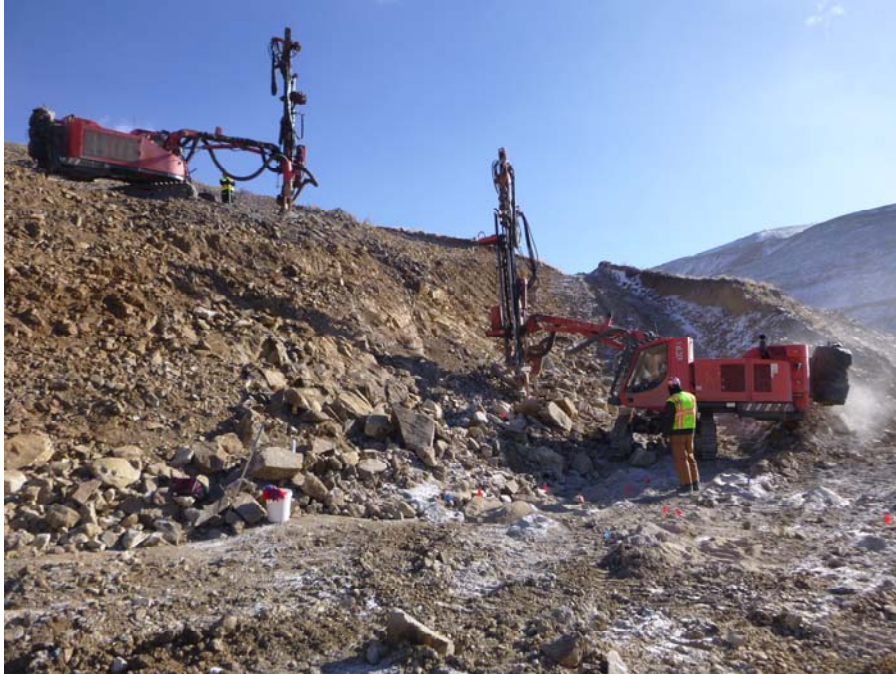
Photo No.3; Continue drilling the “upper/lower drill line” at UG #5126
