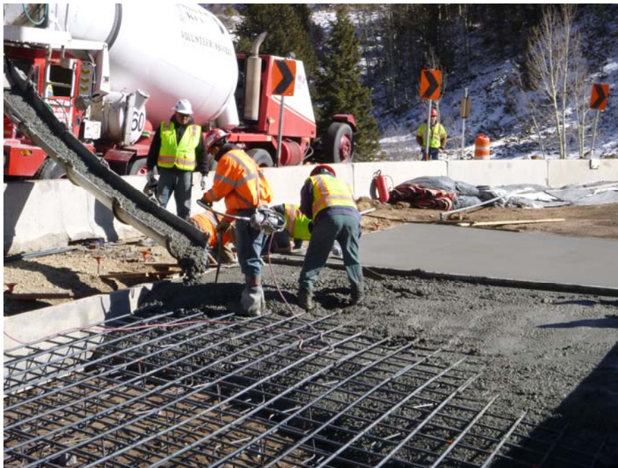
Photo No.2; Concrete placement East portion of crossing HWY 67
