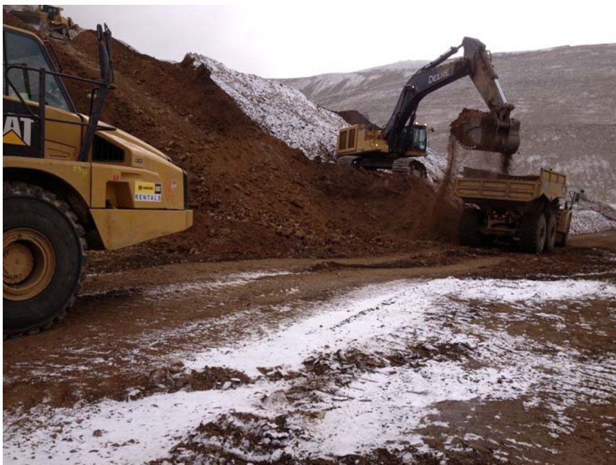
Photo No. 2; Cut material (structural fill) transported to the embankment fill.
