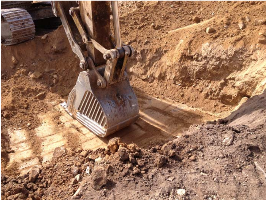
Photo No. 3; UG #6058, UG #6059, backfilling surface workings
