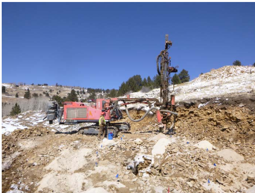
Photo No. 2; Confirmatory drilling at UG #U6113
