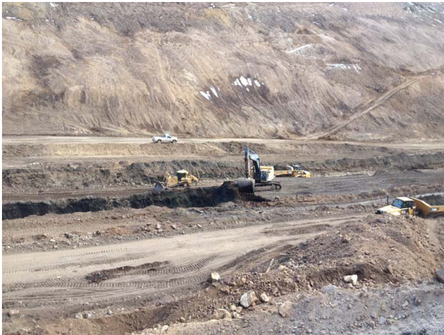
Photo No. 2 removing unsuitable material from within the planned footprint of the Hwy 67 embankment
