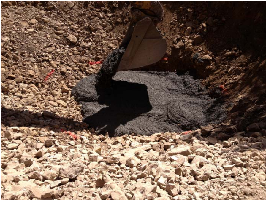
Photo No. 3; UG #6061 (Historical # 338) known as a shaft: placing the concrete “plug”.
