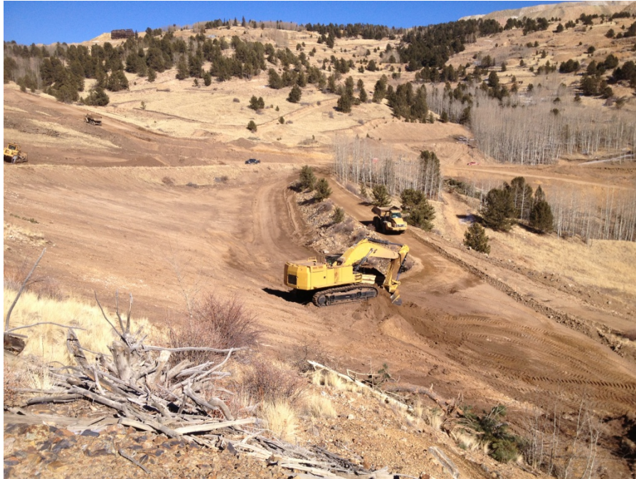
Photo No.3; completing the removal of topsoil, approximate Station 42+00, Left centerline ADR Haul route
