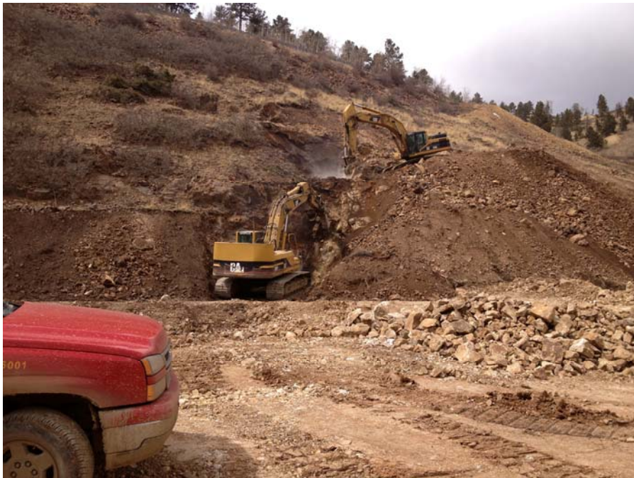
Photo No.4; UG #6030: Removing shot rock and breaking out the remaining crown pillar
