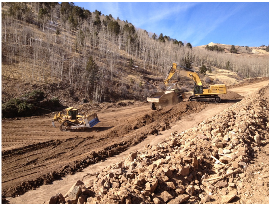
Photo No.4; Topsoil removal, looking northwest. Left Station 23+00 ADR haul route
