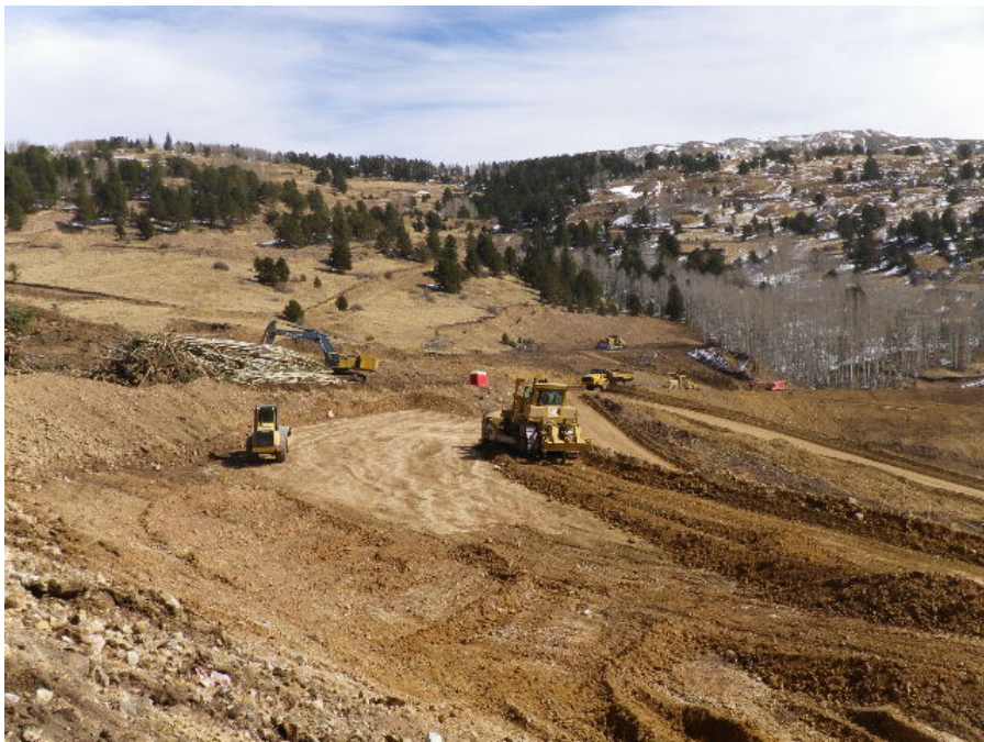
Photo No. 4; Structural Fill placement and compaction
