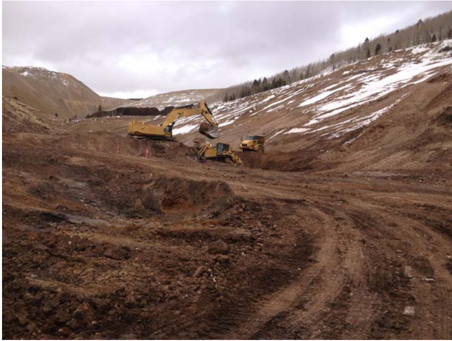
Photo No. 1; Topsoil removal view looking east from the proposed underdrain ponds
