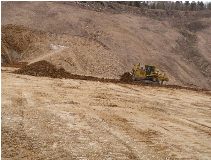
Photo No. 2; Structural Fill placement within the VLF Phase I
