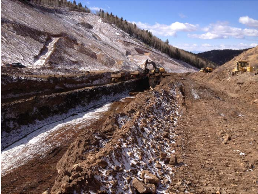
Photo No. 1; Removal of unsuitable material from the embankment footprint
