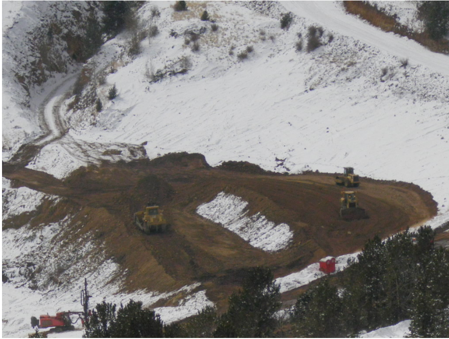
Photo No.3; Structural fill placement and compaction efforts at approximate Sta. 37+00 thru 42+00
