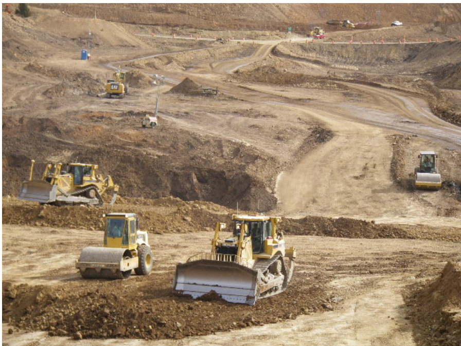
Photo No. 4; Structural fill placement and compaction
