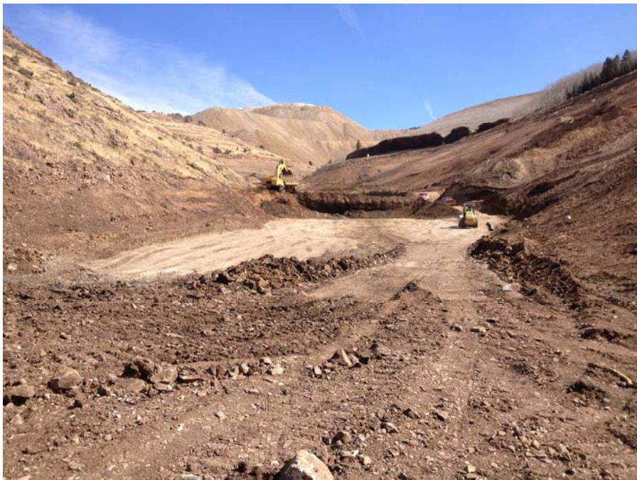
Photo No. 2; “Proof rolling” the approved subgrade within the downstream toe of the embankment
