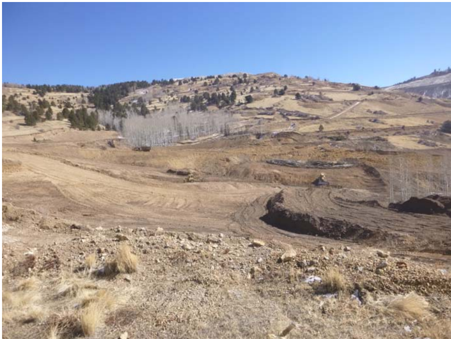
Photo No.4; Topsoil removal and stockpile tree/slash relocation left of the ADR haul route Station 35+00(+/-)
