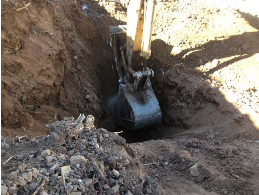
Photo No. 1; UG #6077 known as a collapsed shaft, excavated to about 12 feet into competent rock
