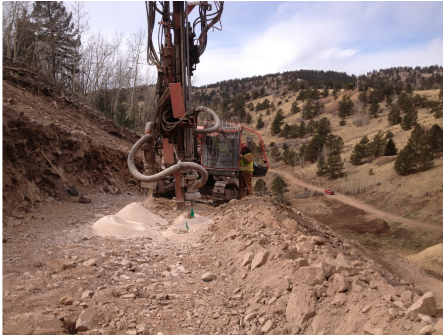
Photo No.1; Upper bench conformation drilling UG #6017
