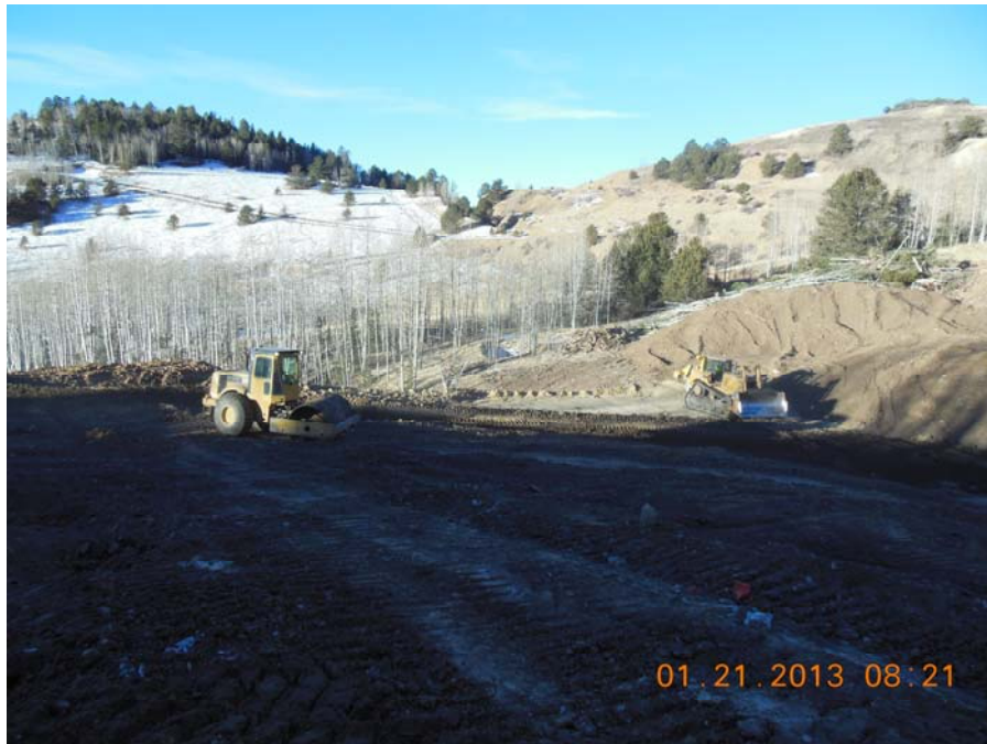
Photo No.1; Fill and Compaction efforts - Planned 740 haul route
