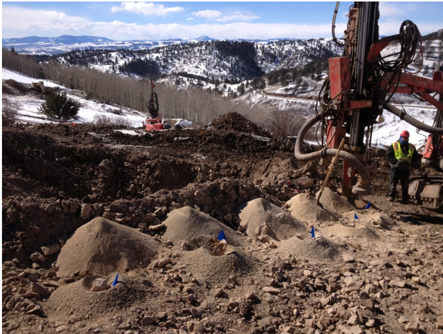
Photo No.2; Confirmatory drilling UG #6037, background: drilling at UG #6036
