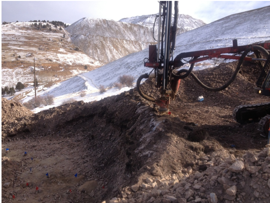
Photo No.4; UG #6037, drilling upper access provided
