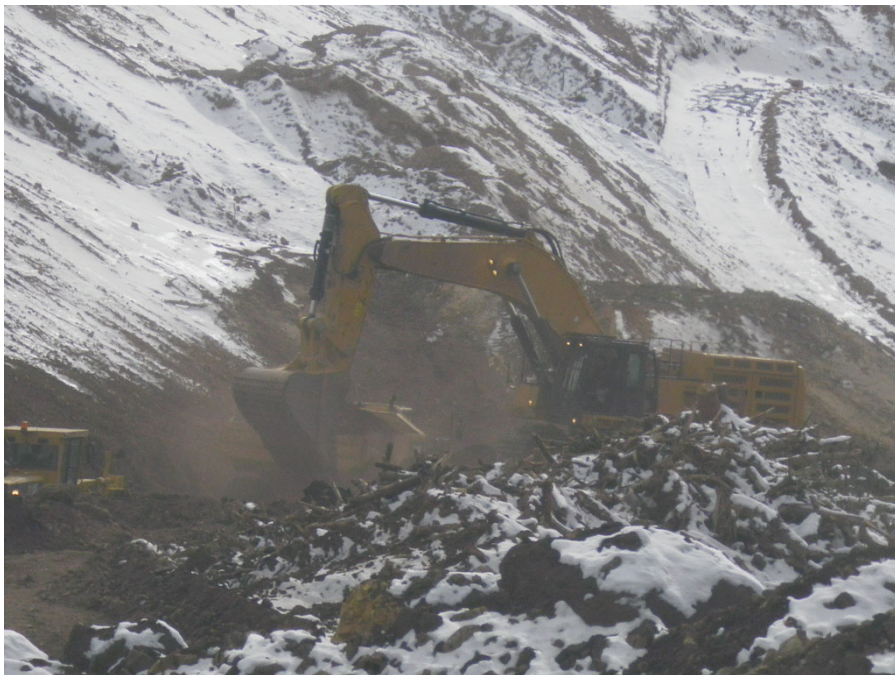
Photo No.3; Topsoil removal within the PSSA limits (West of Hwy 67 crossing)
