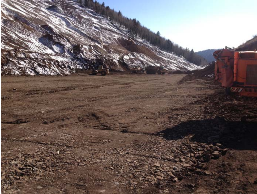
Photo No. 1; Embankment fill: First lift, view west
