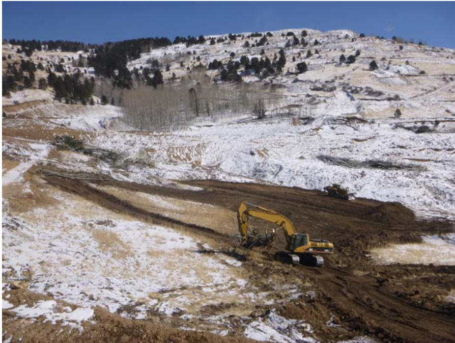
Photo No.1; Topsoil removal and stockpile and tree/slash relocation left of ADR haul route Station 33+00(+/-)
