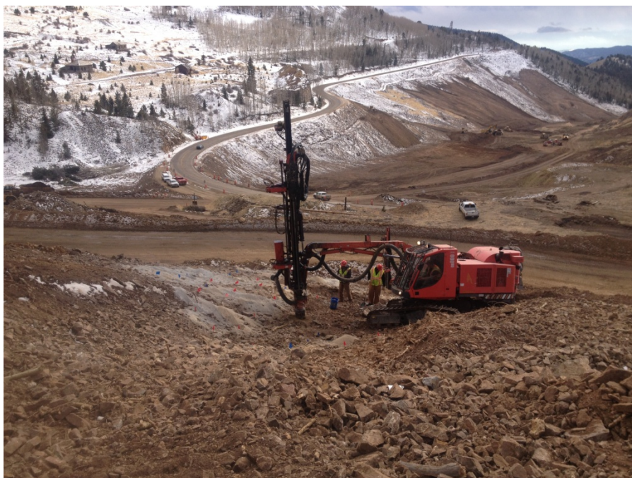
Photo No.2; Continue drilling the “upper drill line” at Historical UG #372
