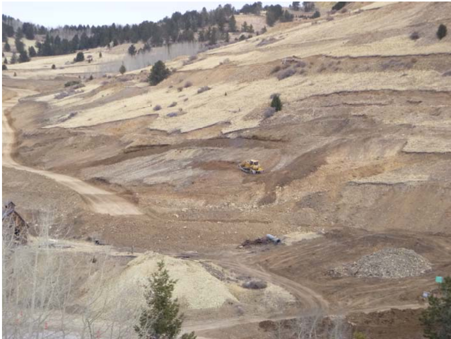
Photo No.4; Topsoil clearing/removal
