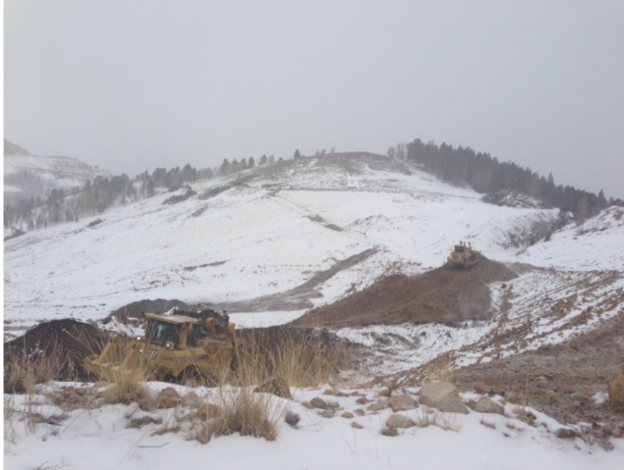
Photo No.1; structural fill placement and compaction efforts, prior to shut down
