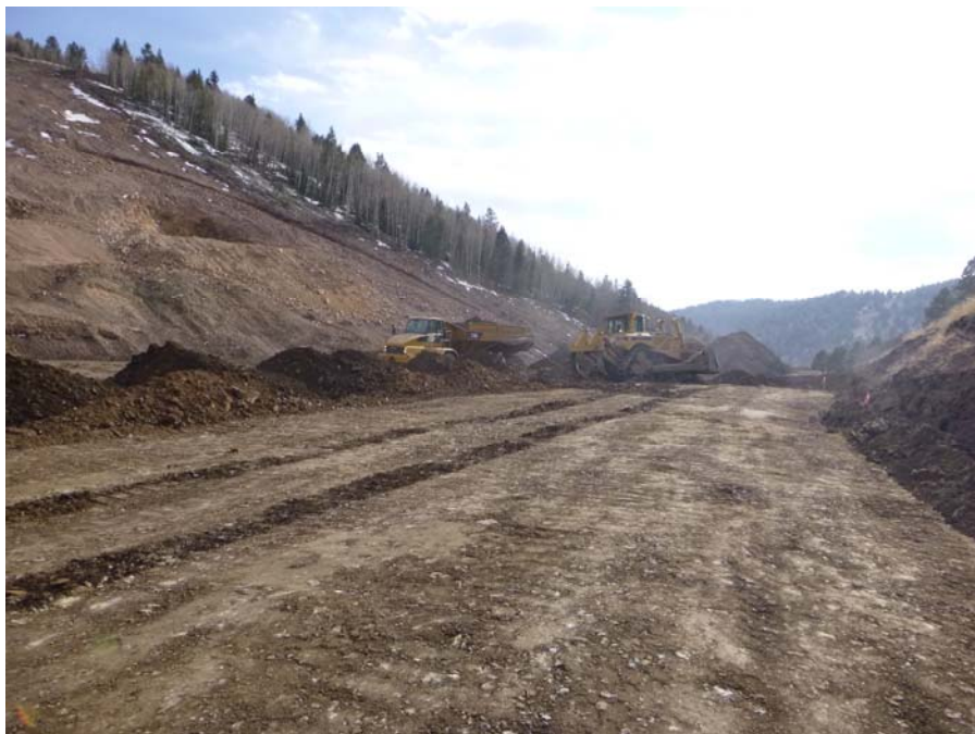
Photo No. 4; Continuing embankment fill placement
