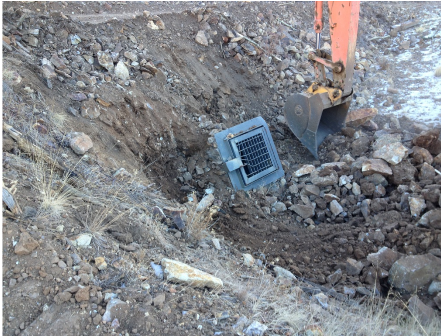
Photo No.1; UG # 5260 Exposing 36" CMP and grate
