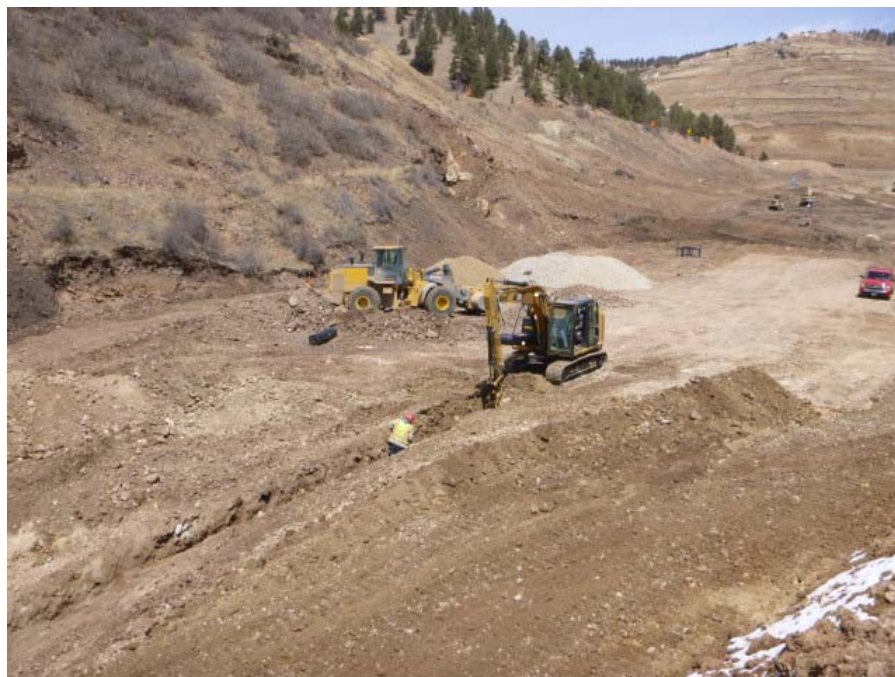
Photo No. 2; Primary Underdrain construction.
