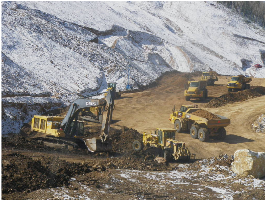
Photo No. 1; Structural Fill Haul for the embankment.
