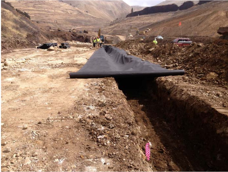
Photo No. 1; Preparing to install the primary underdrain, view east
