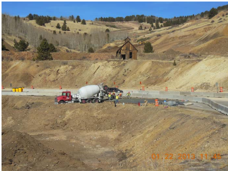
Photo No.2; Concrete placement West portion of crossing HWY 67
