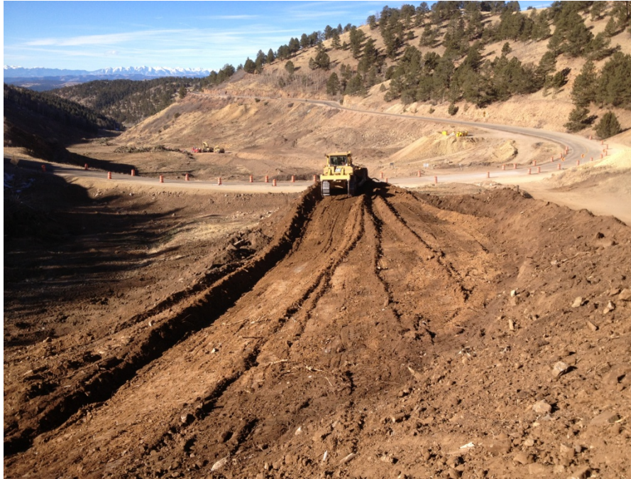
Photo No.3; Topsoil removal right ADR haul route Station 10+00(+/-)
