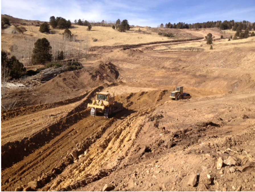
Photo No.3; Fill and Compaction efforts - Planned 740 haul route
