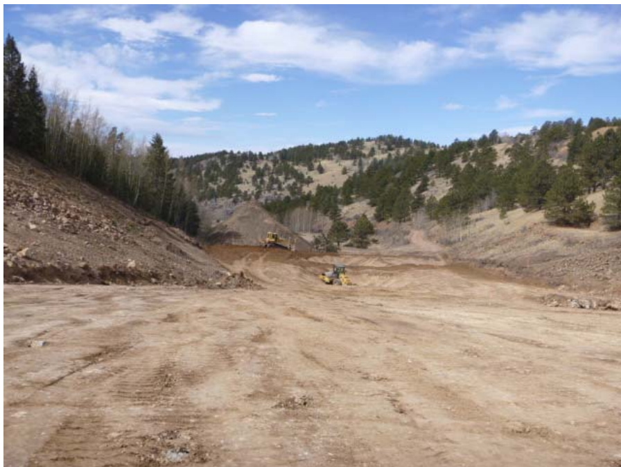
Photo No. 4; Structural fill placement and compaction.
