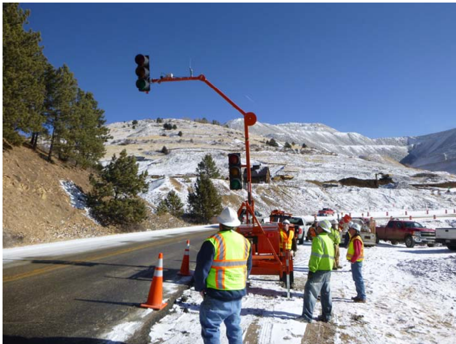
Photo No.2; Remote stop light set up HWY 67
