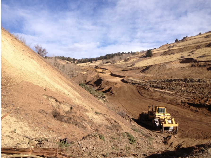
Photo No.1; Looking north uphill, within the natural drainage channel, where the secondary underdrain is planned.
