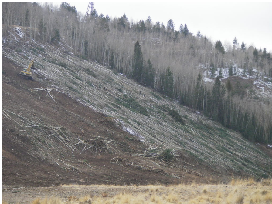
Photo No.4; Tree clearing - West of HWY 67
