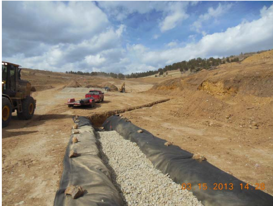
Photo No. 2 Phase I secondary underdrain construction.
