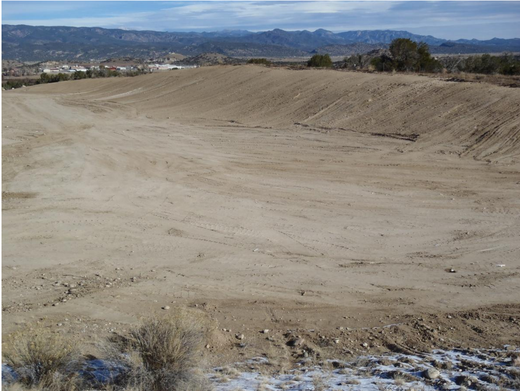
Photo 1. Recontoured east highwall (looking ENE).
