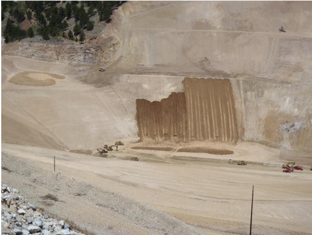
Photo 3. Placement of soil liner fill (SLF) in the PSSA (looking NW).
