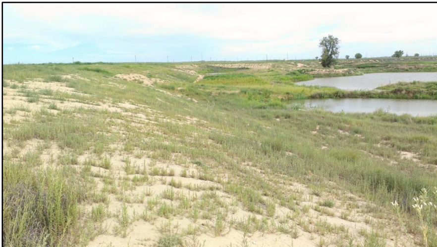
Photo 6. View looking north from southwestern portion of permit area, showing mined slope gradients of 3H:1V or flatter.
