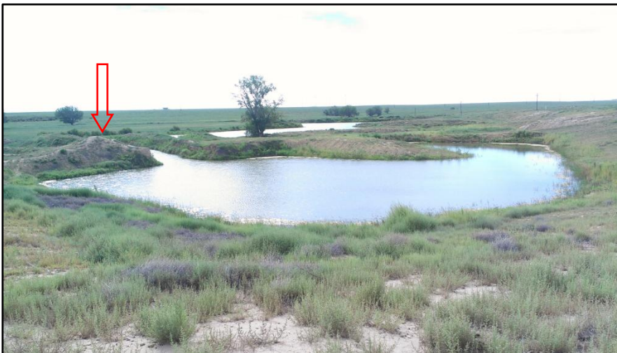
Photo 3. View looking southeast from northwestern portion of permit area, showing water present in recharge pond. Note knob (indicated) that will need to be graded to 3H:1V.
