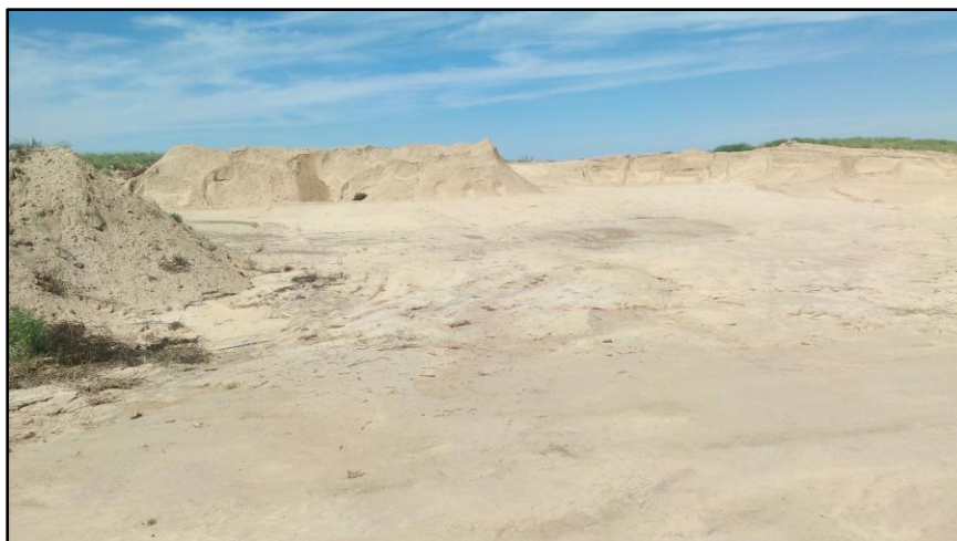
Photo 3. View looking north into pit, showing mined wall that daylights to the south, material stockpile, and portion of topsoil stockpile (at left).
