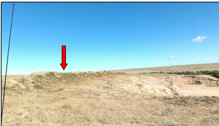
Photo 3. View looking north from haul road, showing topsoil stockpile stabilized with vegetative cover (indicated) located on western edge of current permit area.
