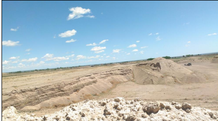
Photo 7. View looking northeast from western edge of pit at northern, south-facing pit wall approximately 250 ft long with a 2H:1V slope.
