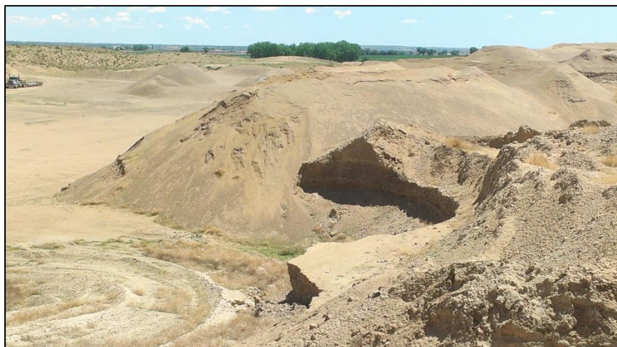
Photo 9. View looking east from southwestern corner of pit, showing north-facing cut approximately 150 ft long with a 1H:1V slope.
