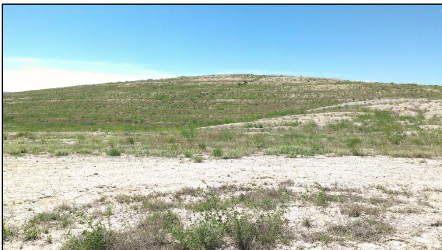
Photo 6. View of large topsoil stockpile stabilized with vegetative cover located at northwestern corner of permit area.
