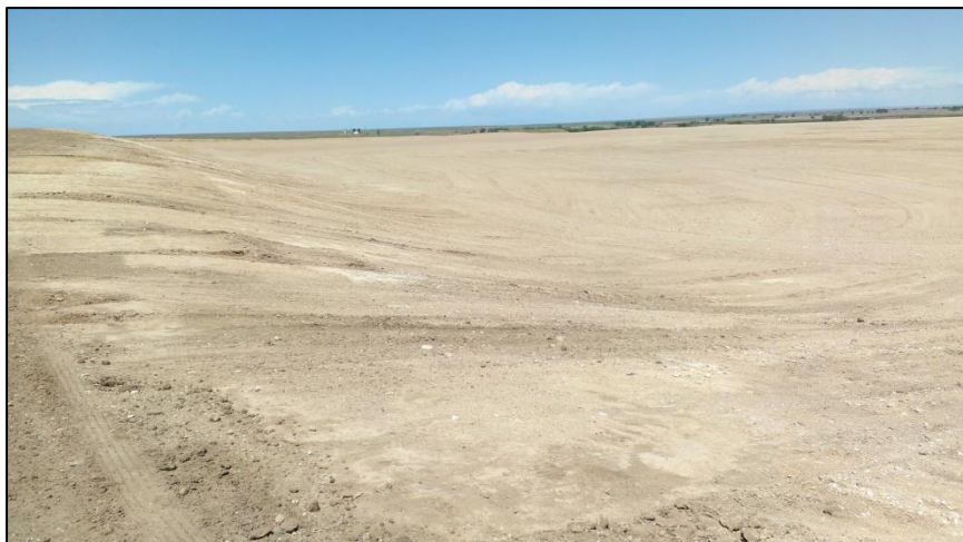
Photo 12. View looking west from southeastern corner of permit area, showing previous north-facing highwall graded to 4H:1V slope.
