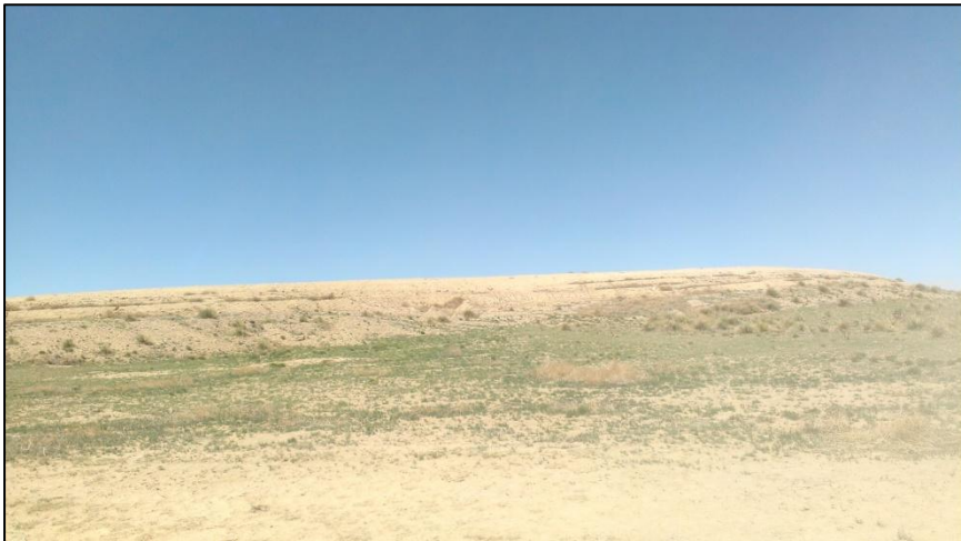
Photo 8. View looking south at berm constructed along northern edge of site to contain stormwater basin.
