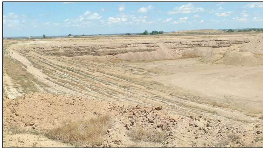
Photo 8. View looking northeast from southwestern corner of pit, showing western, east-facing pit wall approximately 430 ft long with a 3H:1V slope.
