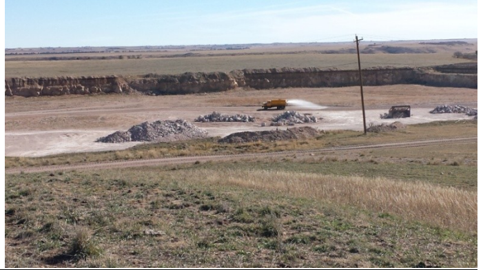
Photo 8 – Water truck spraying for dust control.
