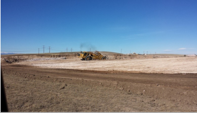
Photo 7 – Scraper removing topsoil.
