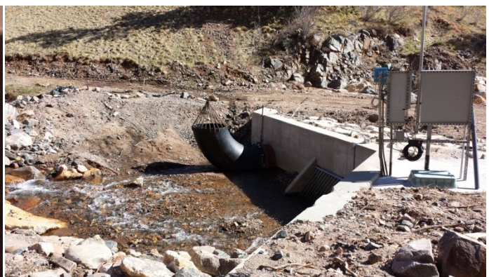
Photo 6 – Ralston Creek diversion inlet pipe with trash rack at upper cutoff wall..
