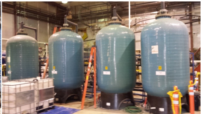
Photo 4 – Resin tanks in ion exchange treatment plant.
