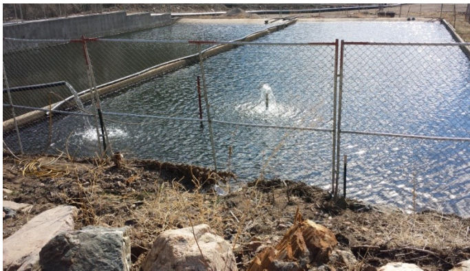
Photo 3 – Concrete-lined ponds outside ion exchange treatment plant.
