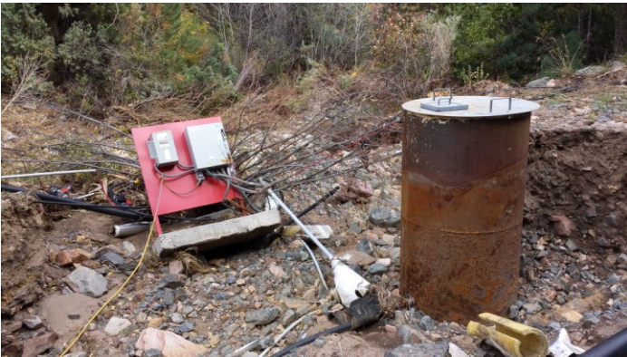
Photo 3 – One of alluvial ground water sumps damaged by storm waters.
