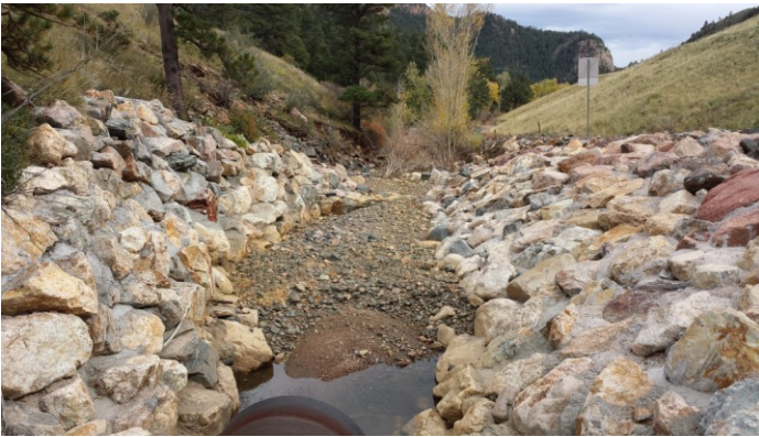
Photo 9 – Ralston Creek channel at outlet end of pipe that extends through diversion cut-off wall on west side of permit area
