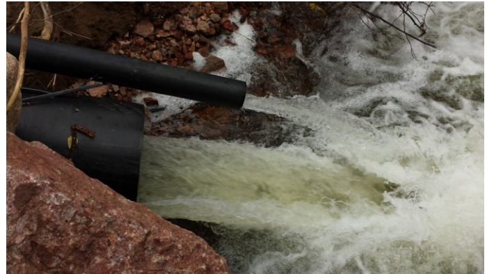
Photo 4 – Discharges into Ralston Creek near BPL from creek diversion (large HDPE) and ion exchange treatment plant (small HDPE).
