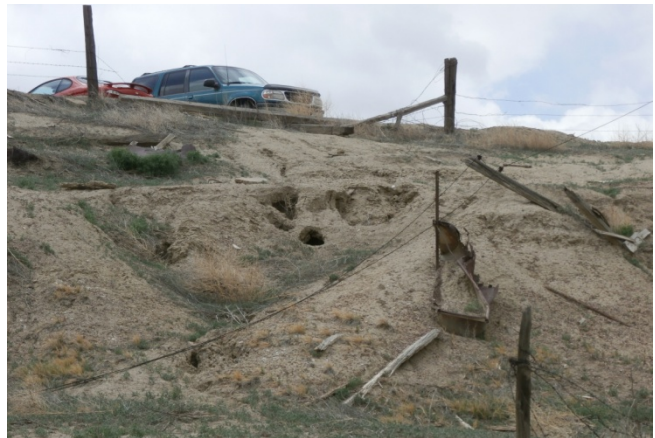
Figure 17: Openings on the slope northwest of Phase 1.
