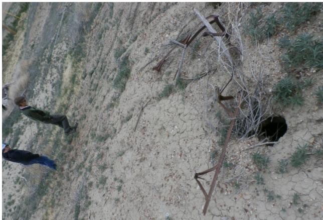
Figure 16: Openings in ground northwest of Phase 1.
