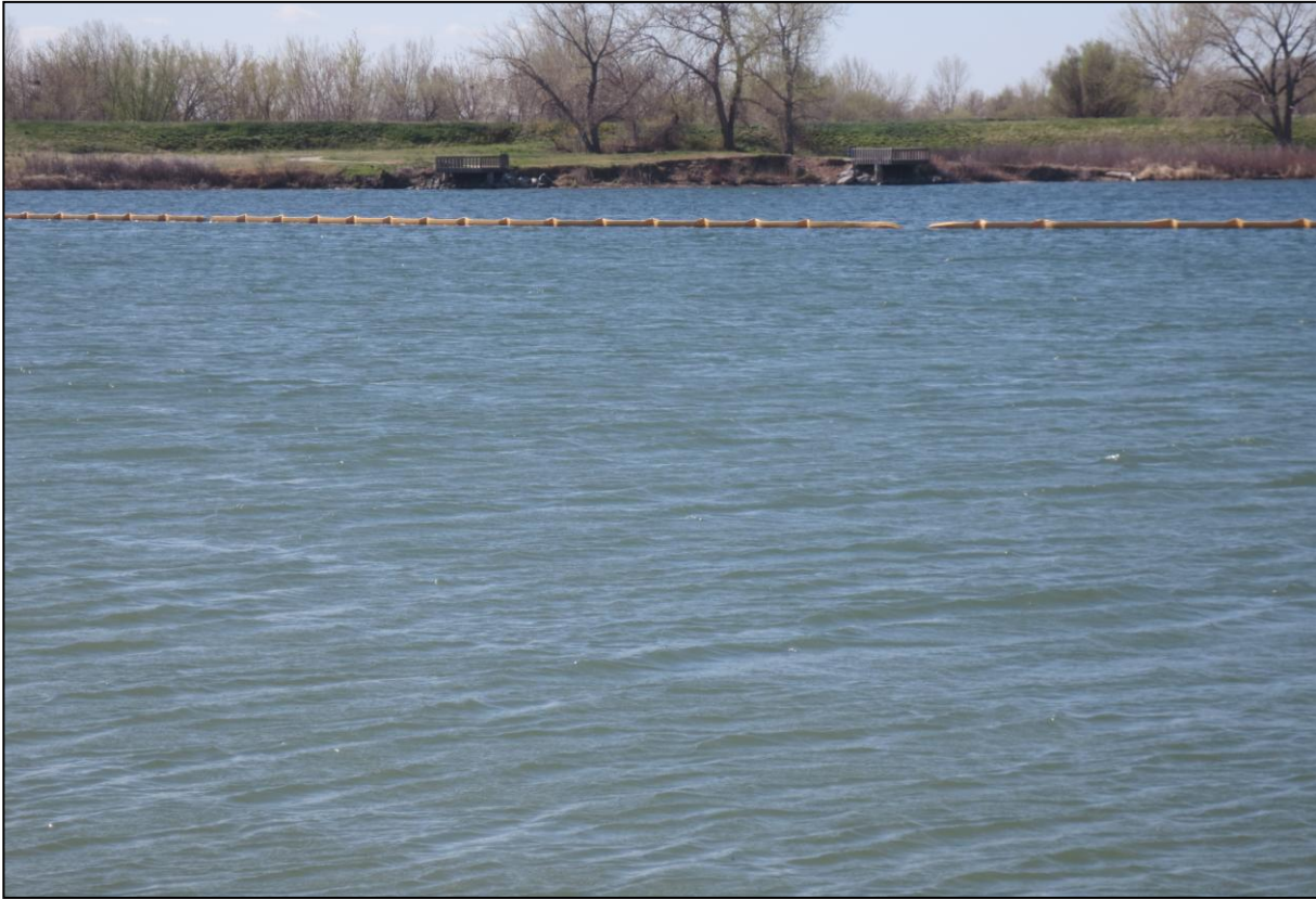
Photo 3: Turbidity curtain in the foreground. Slopes in the background that will need to be re-graded to 3H:1V.
