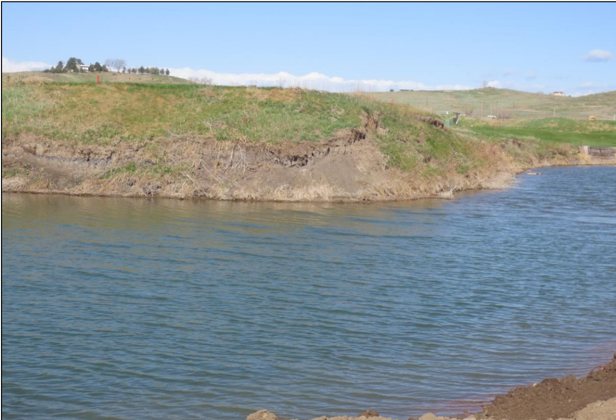
Photo 2: Unstable slope along the shoreline of the golf course. The Operator will need to stabilize and establish vegetation on the slope.
