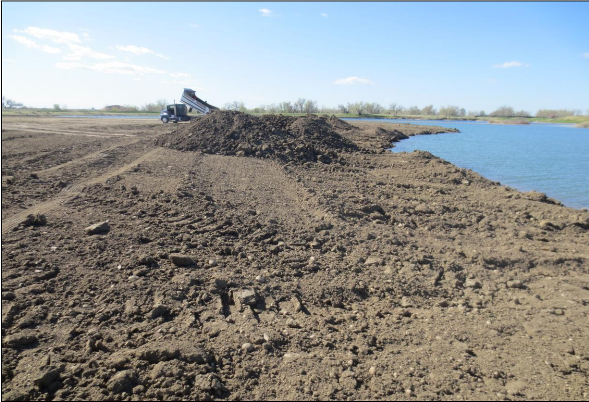
Photo 1: Dump truck placing inert fill in the northern portion of the site.
