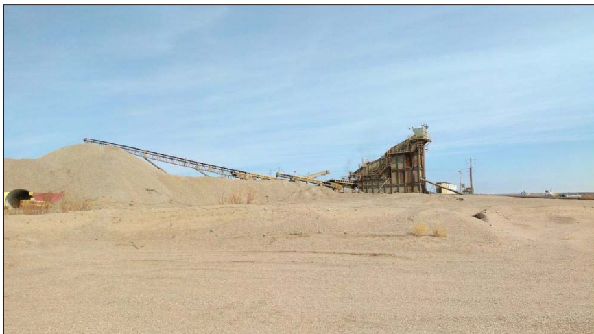
Photo 6. View looking north, showing material processing and stockpiling area located at center of site.
