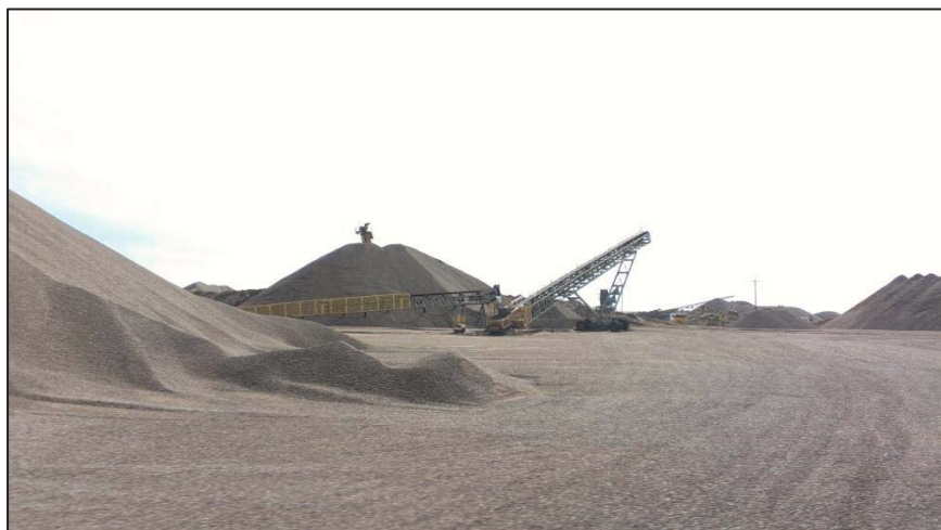
Photo 9. View looking east across western pond, with material processing and stockpiling area shown in the background.
