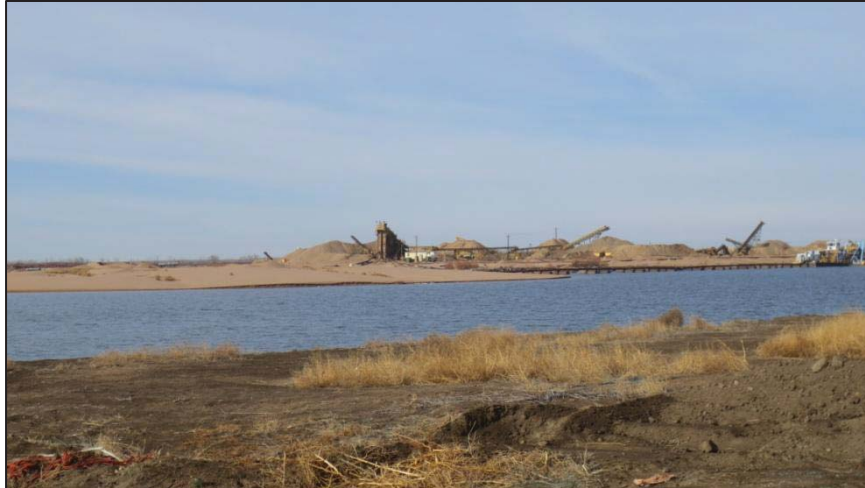
Photo 10. View looking west, showing eastern pond in foreground and processing and stockpiling area in background. Floating suction dredge is shown at far right.
