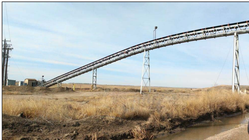
Photo 5. View looking west, showing elevated conveyor that crosses the railroad tracks to the north of the site.
