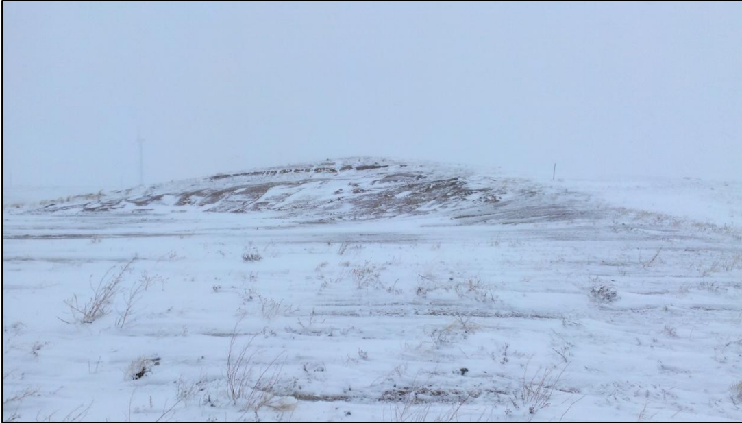
Photo 3. View looking south at southern (north-facing) wall that has been regraded mostly to 3H:1V.
