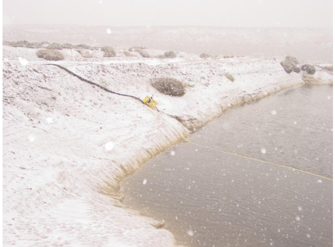
Pumping from dewatering pond 5 to artificial wetlands.
