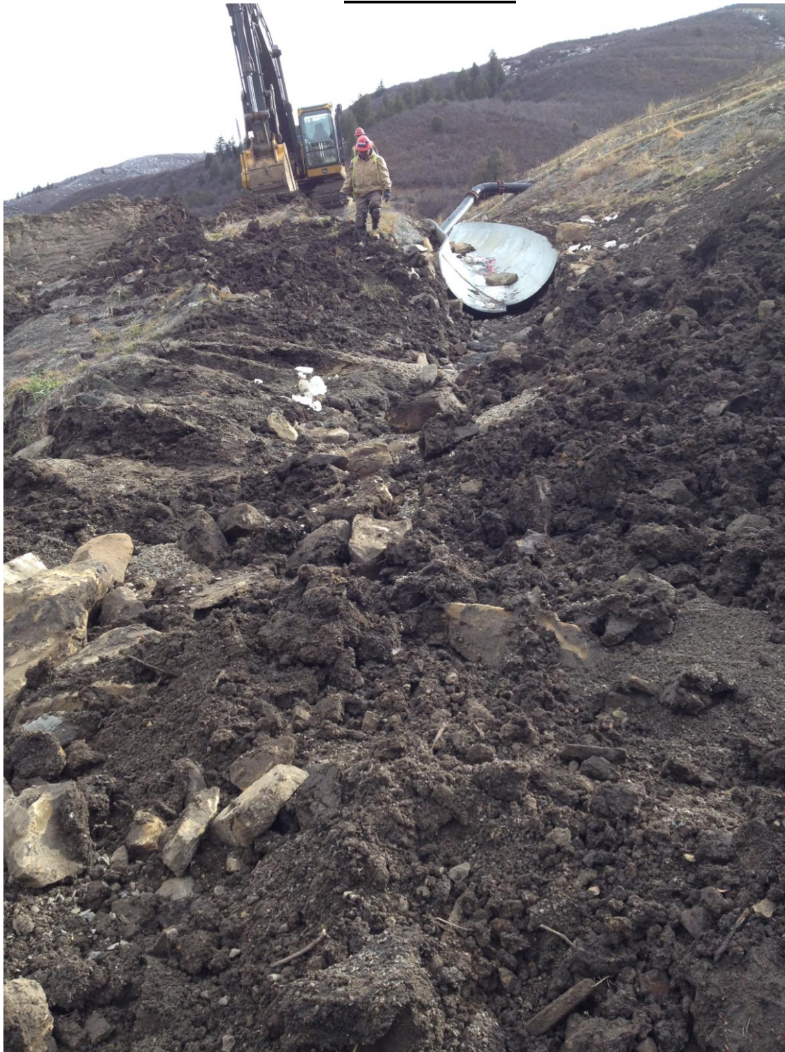
RPEE sediment ditch work
