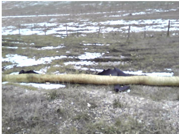
Photo 1: Straw wattles anchored in place at Substation SAE
