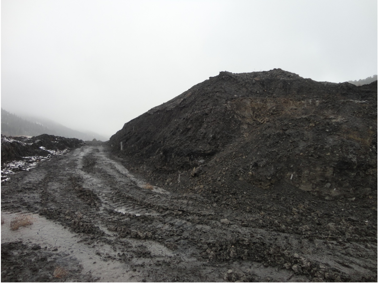
Photo 9: DWDA2, toe to be re-graded
