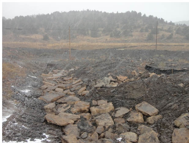
Photo 5: Newly armored ditch below C30 (2)
