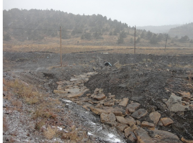
Photo 4: Newly armored ditch below C30
