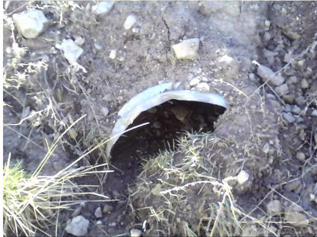
Photo 2: Culvert PM-3 outlet needs clean out
