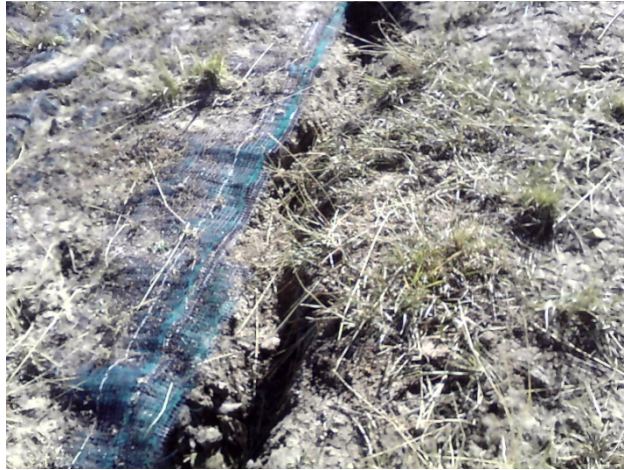
Photo 6: side cutting along TRM in gully repair upslope from PM-3 culvert
