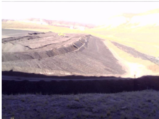
Topsoil Placement
