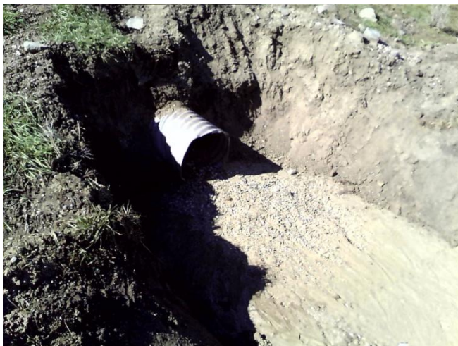
18RT Access Road Culvert Maintenance Work
