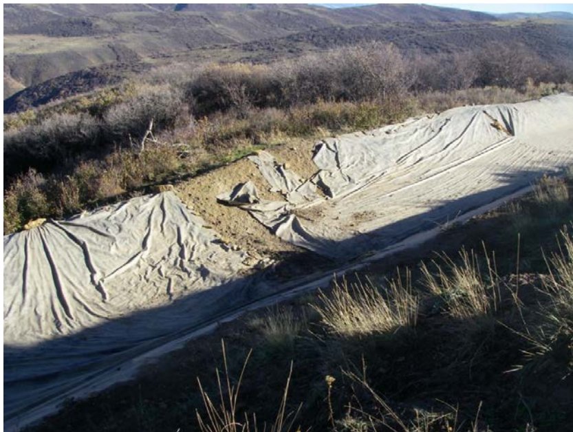
Section 28 Ditch – damaged liner
