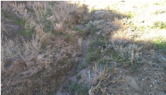
Rill forming on drainage slope.
