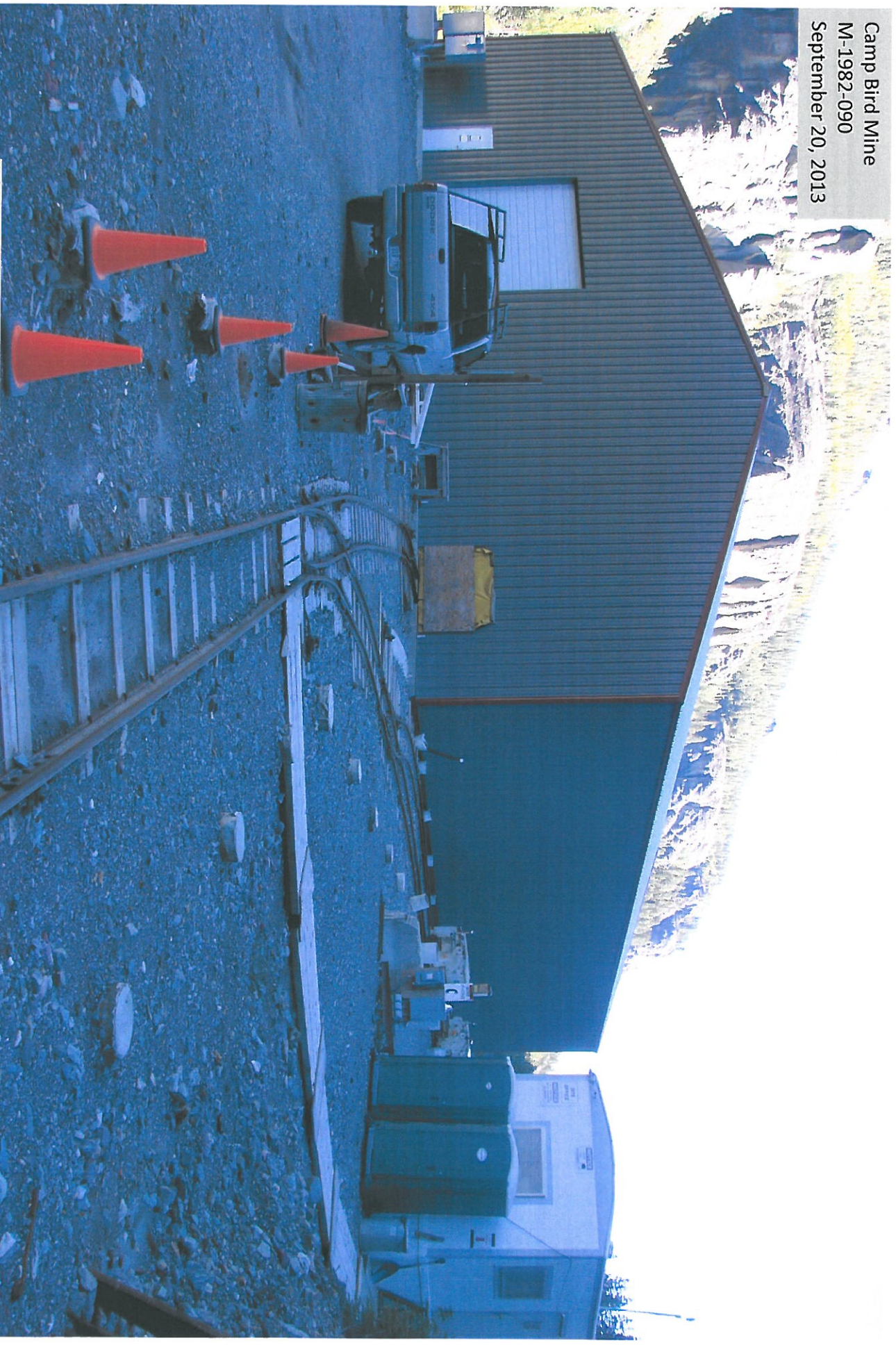
View north, taken from the 14L portal and showing the recently constructed 80 x 100 foot steel building. Concrete footers appeared ready for construction of the snow shed, which will cover the rail line from the steel building to the portal and beyond the steel building to the ore bin.
