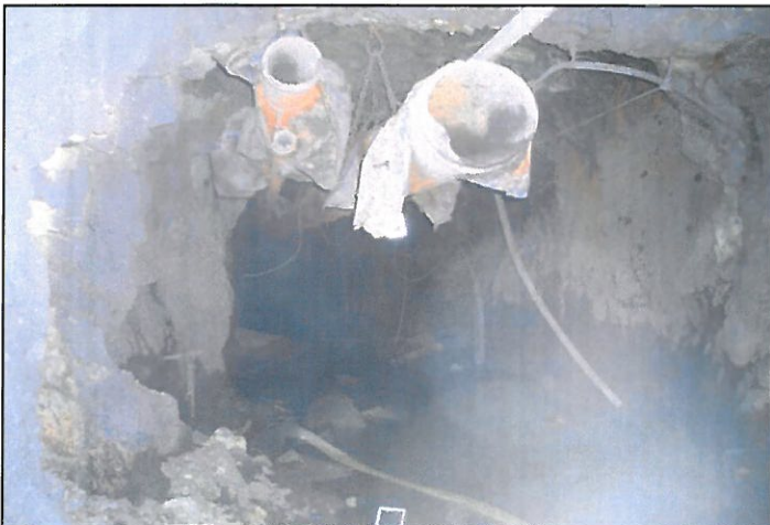
Vent duct and mine pool in old Bulldog 9360 workings
